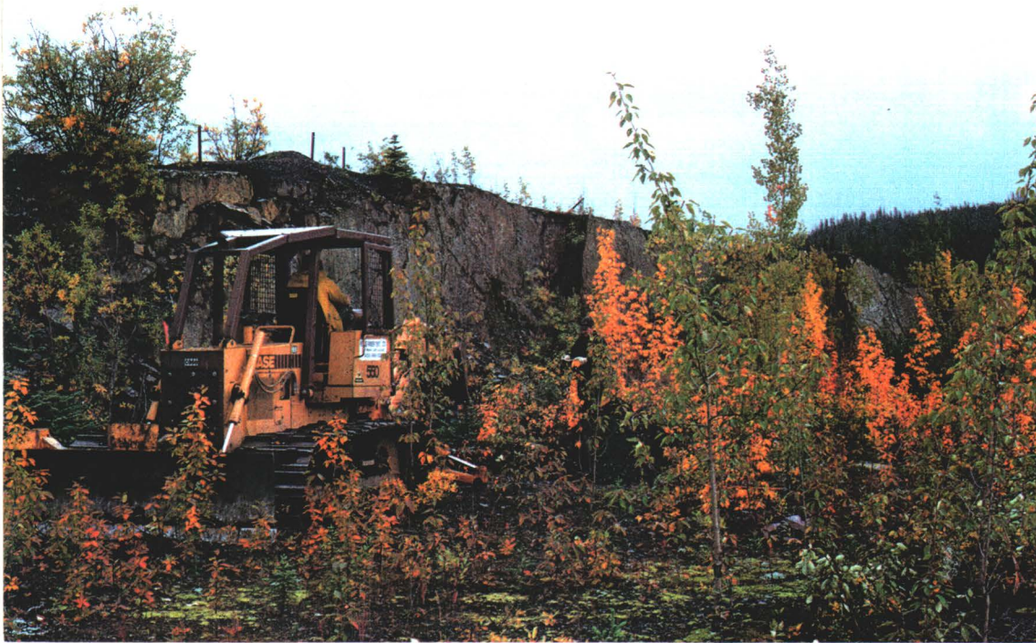
Test pitting soils in front of rock face. Looking west.
