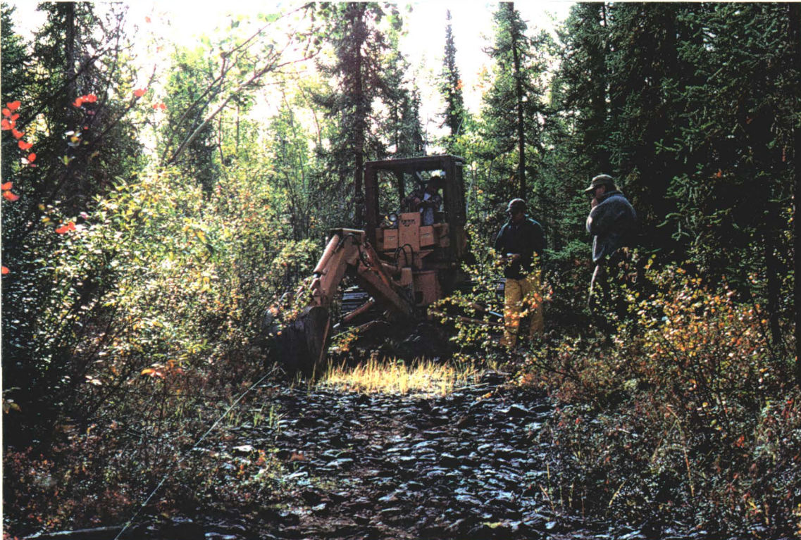
Test pitting shallow soils in area of solidified oil.
