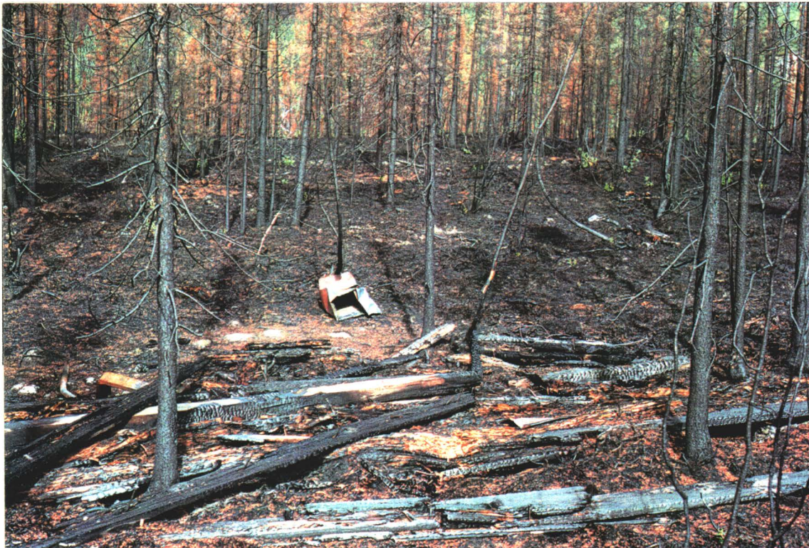
Burned-out wood frame structure.
