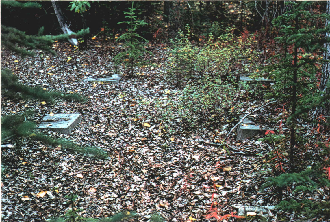
Concrete pads from former above ground storage tank location.
