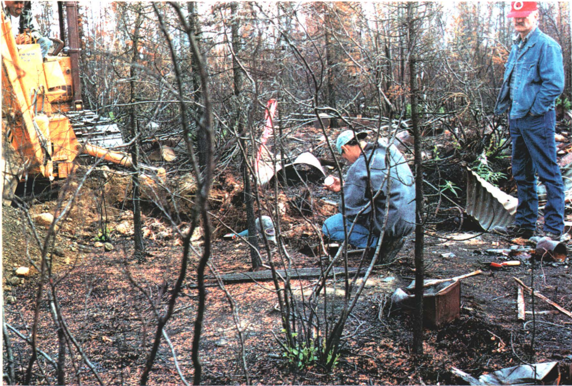
Test pit sampling of soils in refuse area.
