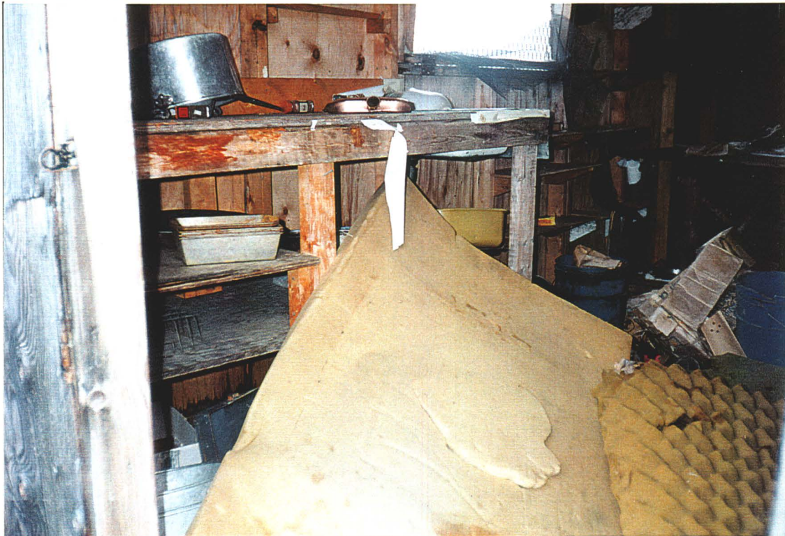
Photo 66: Site 42-CA-34. Interior of frame structure, October 1996.
