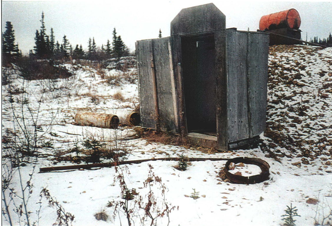
Photo 74: Site 42-CA-34. Former shower building, October 1996.
