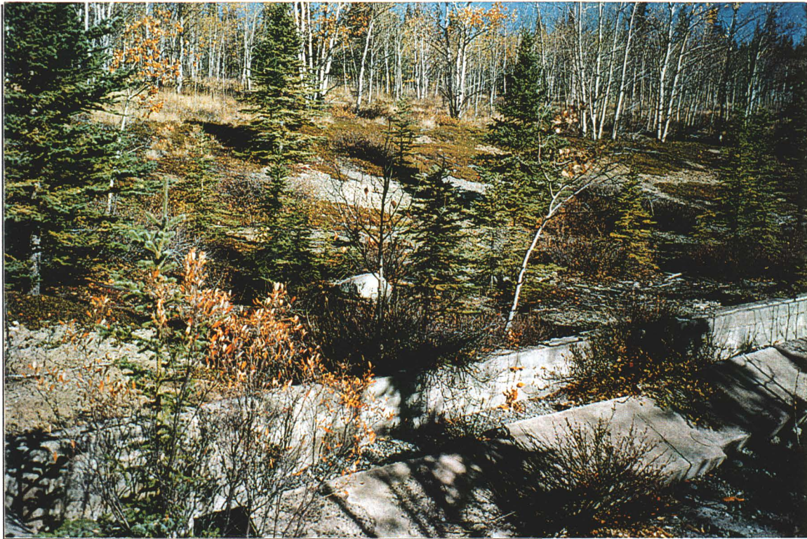
Photo 17: Site 20-A: Pumping station foundation ruins, September 1996.
