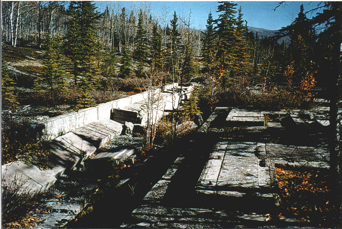
Photo 18: Site 20-A: Pumping station foundation ruins, September 1996.
