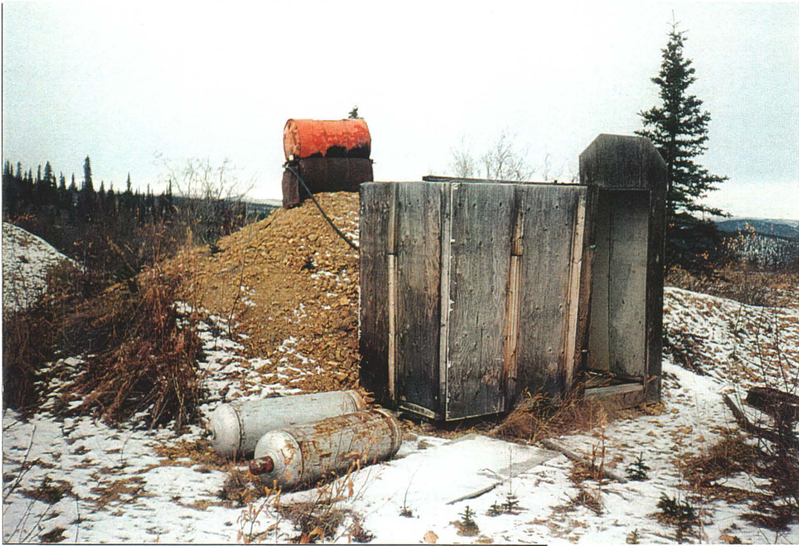
Photo 73: Site 42-CA-34. Former shower building, October 1996.
