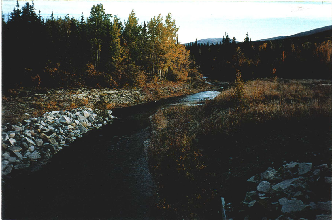
Photo 2: Site 19. Cracker Creek, looking north from Alaska Highway, September 1996.
