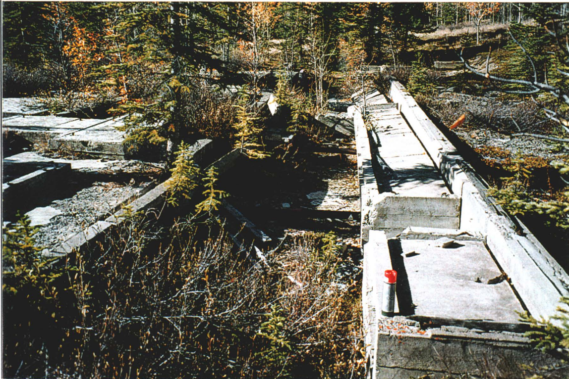
Photo 16: Site 20-A: Pumping station foundation ruins, September 1996.
