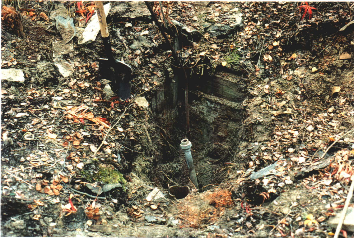
Site 14-A (Note valve rod, galvanized and cast iron pipes.)
