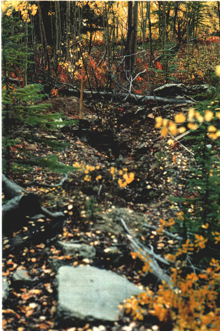
Site 14-A (Note valve handle beside shovel.) (Note broken concrete at bottom of photograph.)
