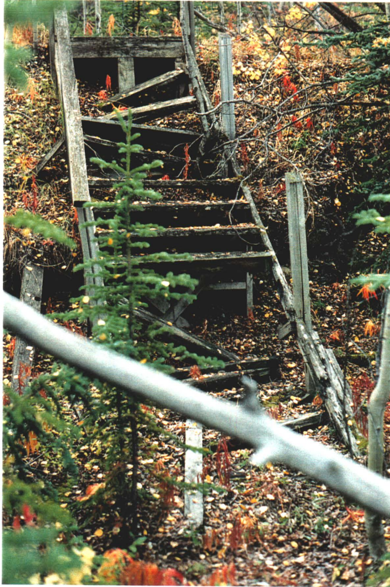
Site 14 - A Upper Staircase
