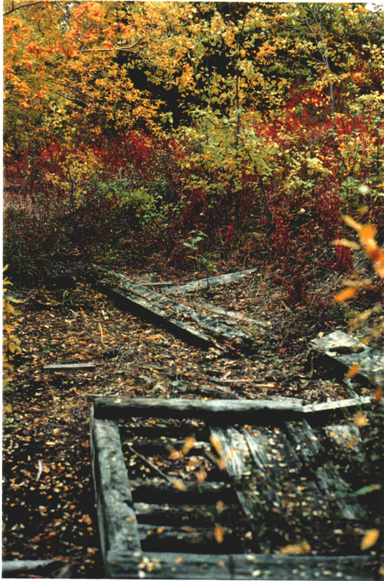
Site 14 - B Wooden Debris
