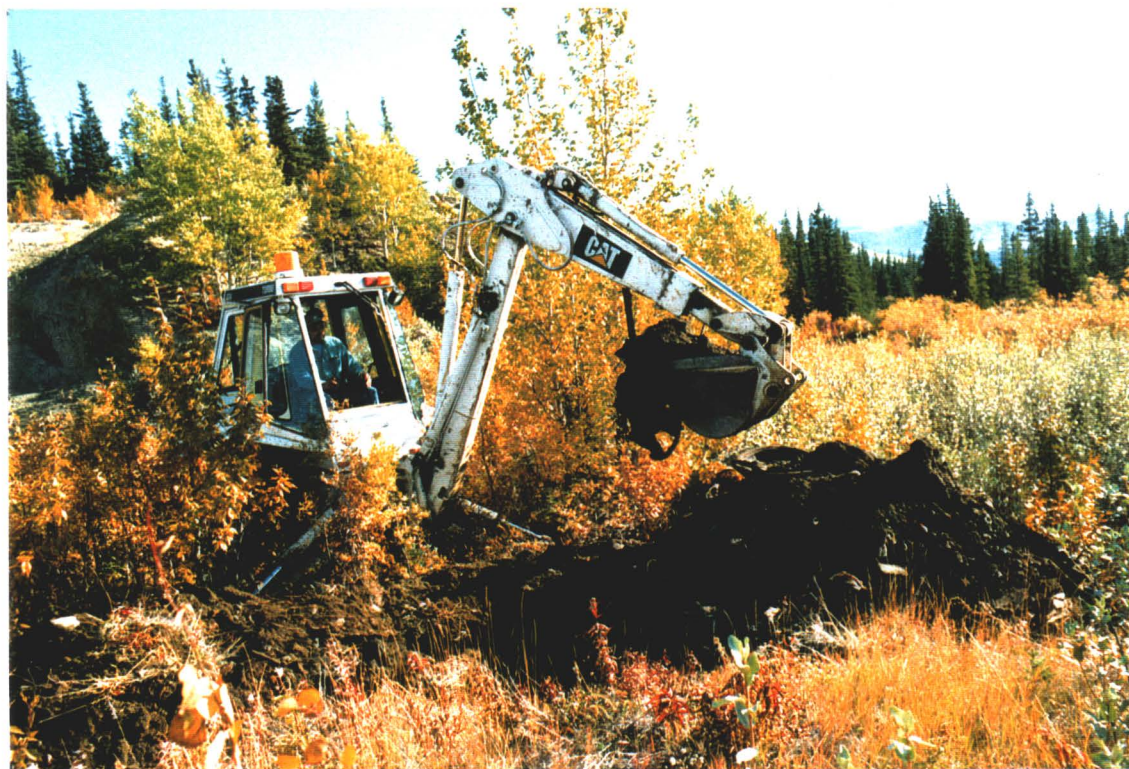
PLATE S4 - Test pit S-2 at southeast extent of buried dump.
