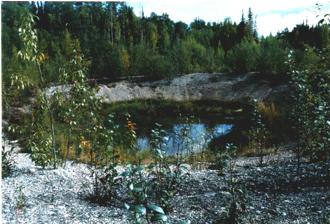
PLATE 14 - Unused sewage disposal pit in clearing south of camp. According to local residents, the pit was never used.
