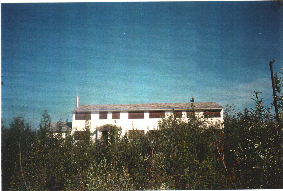
Multi-family Dwelling, exterior. Wooden siding, coated with lead-based paint.
