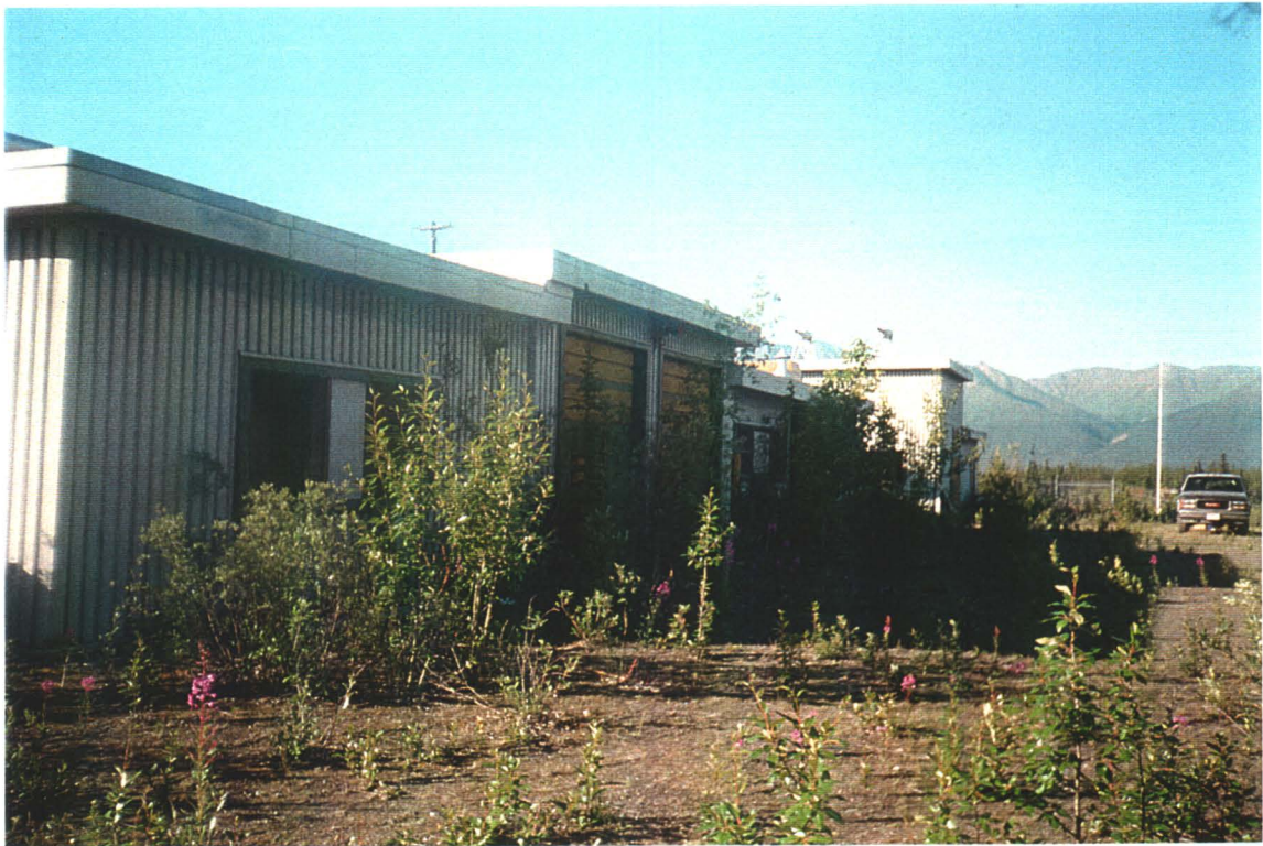
Main building. View of front from opposite end.
