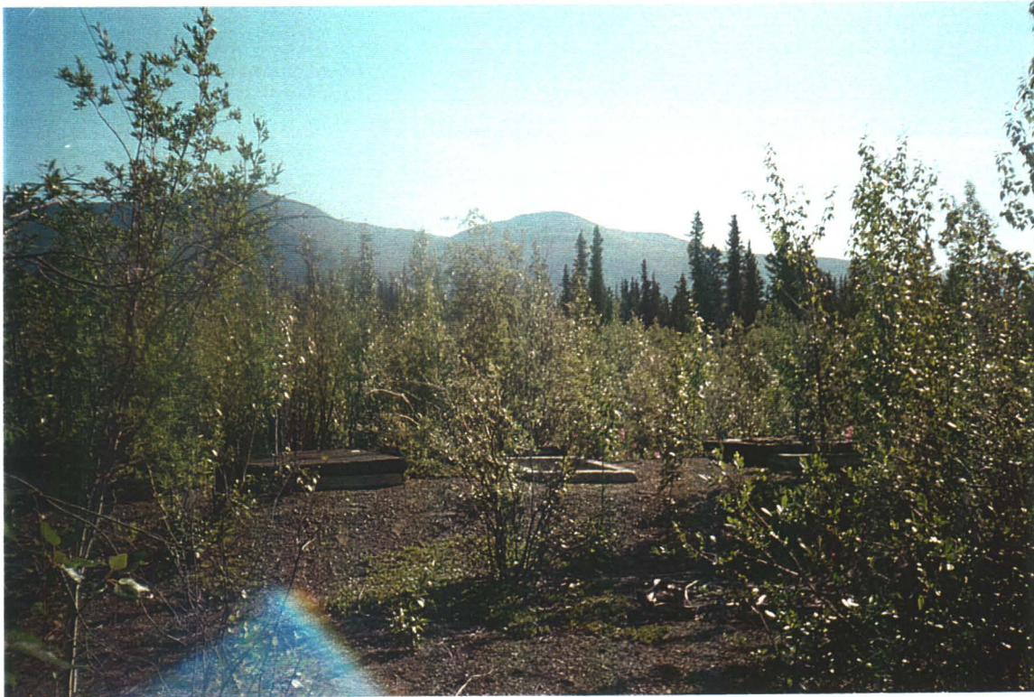
Sewage system vault array.
