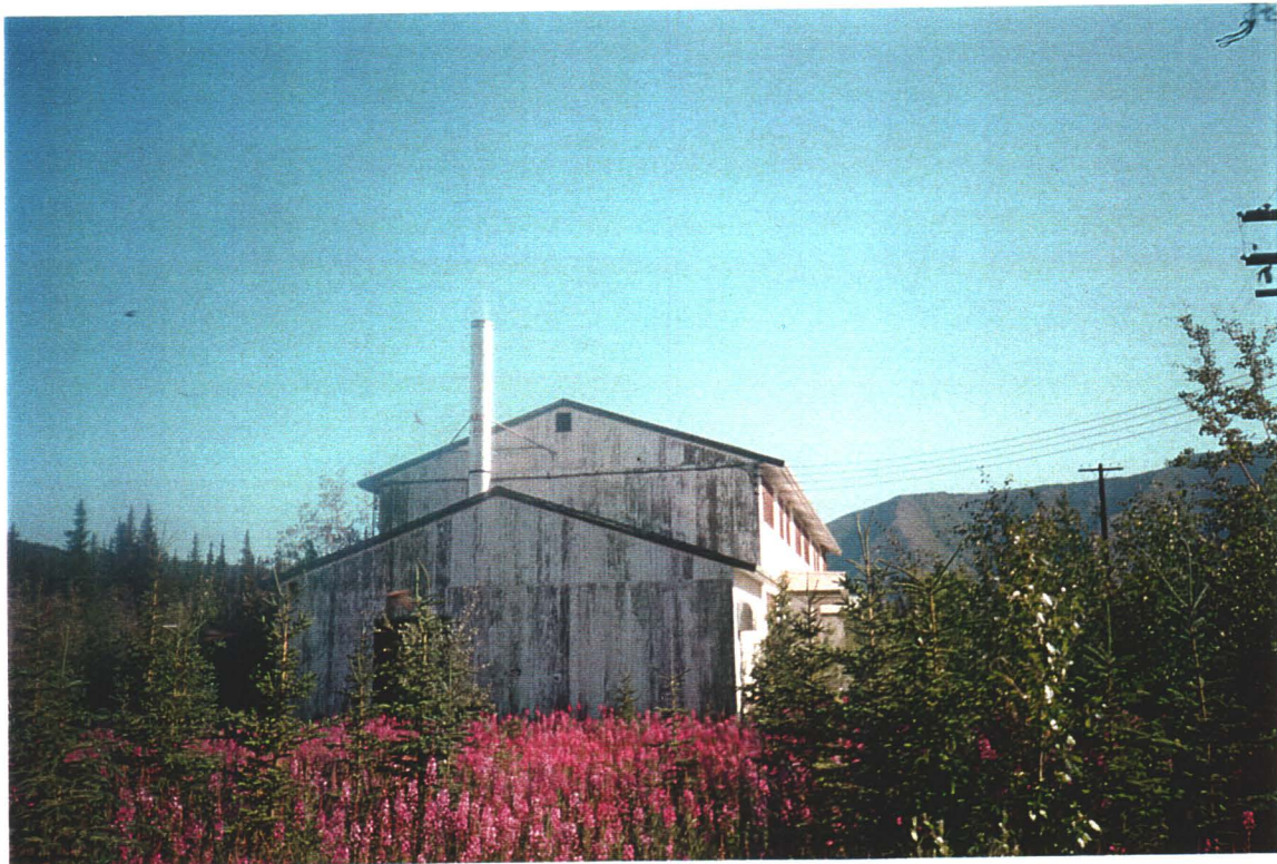
Multi-family Dwelling. Exterior view. Lower end building is the boiler house, which supplies heat to this dwelling as well as to Main Building and Compressor Building by underground steam piping system.
