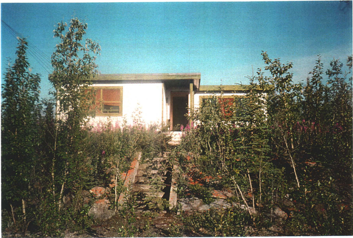
Single Residence, exterior front.
