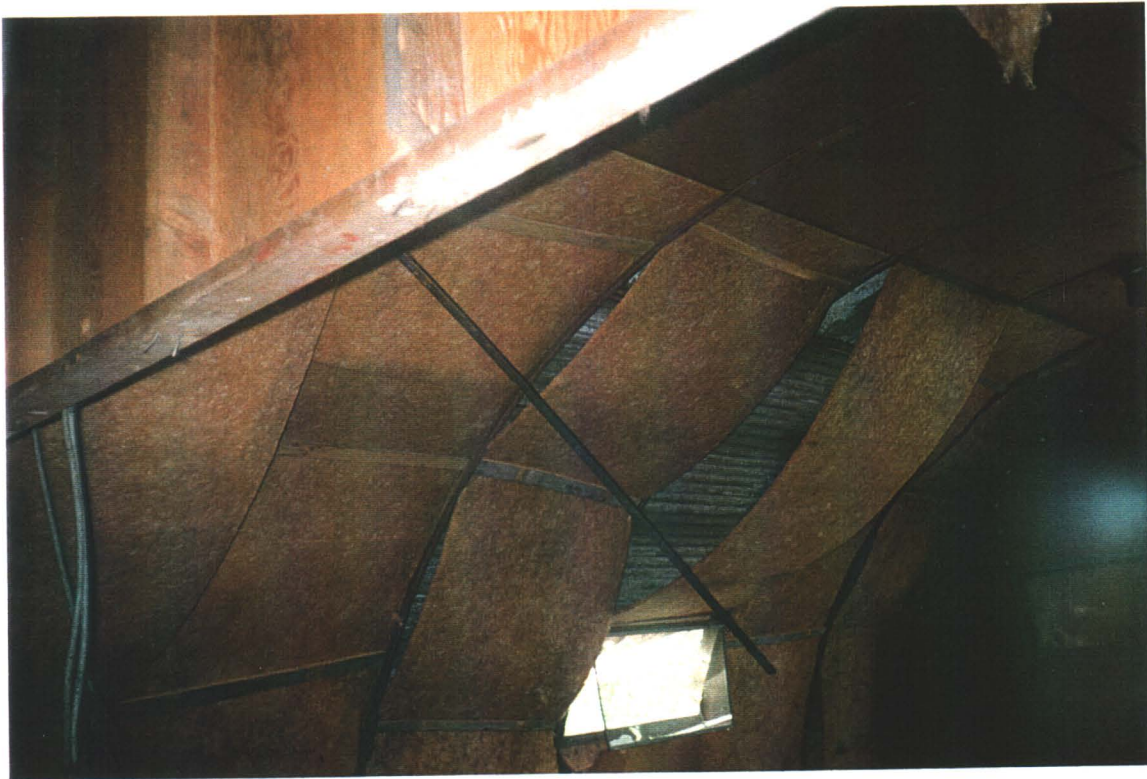
Interior of Quanset. Loose fibreglass insulation.
