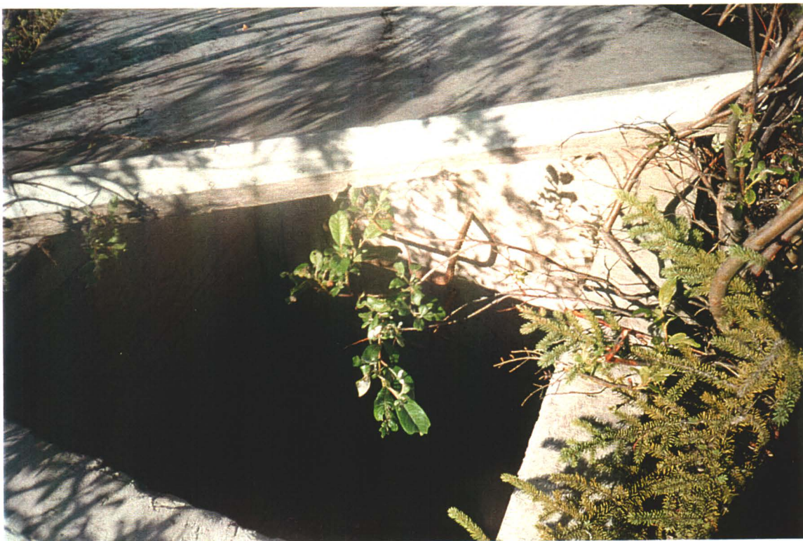
Detail of vault interior.
