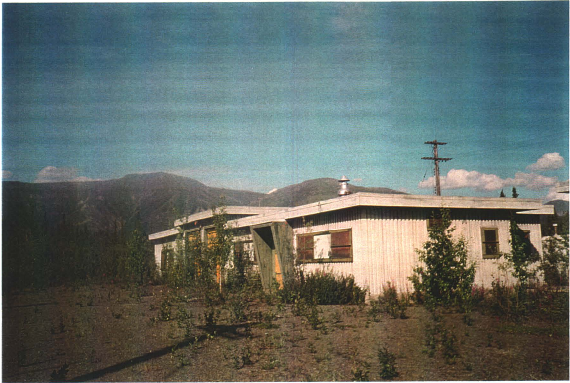
Main building. Front of building, which houses office, shop, generator room, and water supply.
