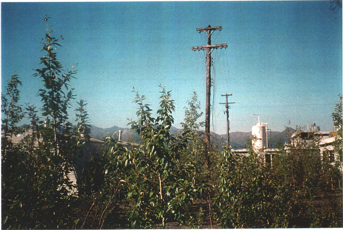
Typical power pole array, both frames. Power disconnected. No pole-mount transformers.
