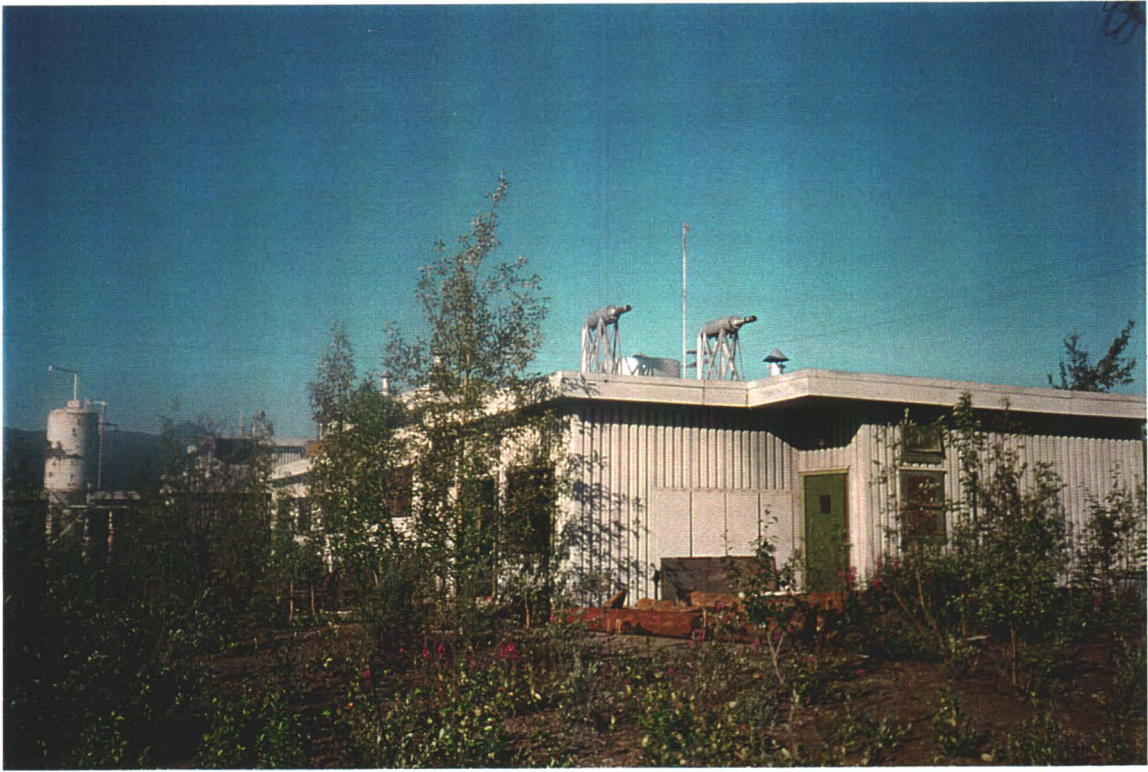
Main Building. View from opposite end.
