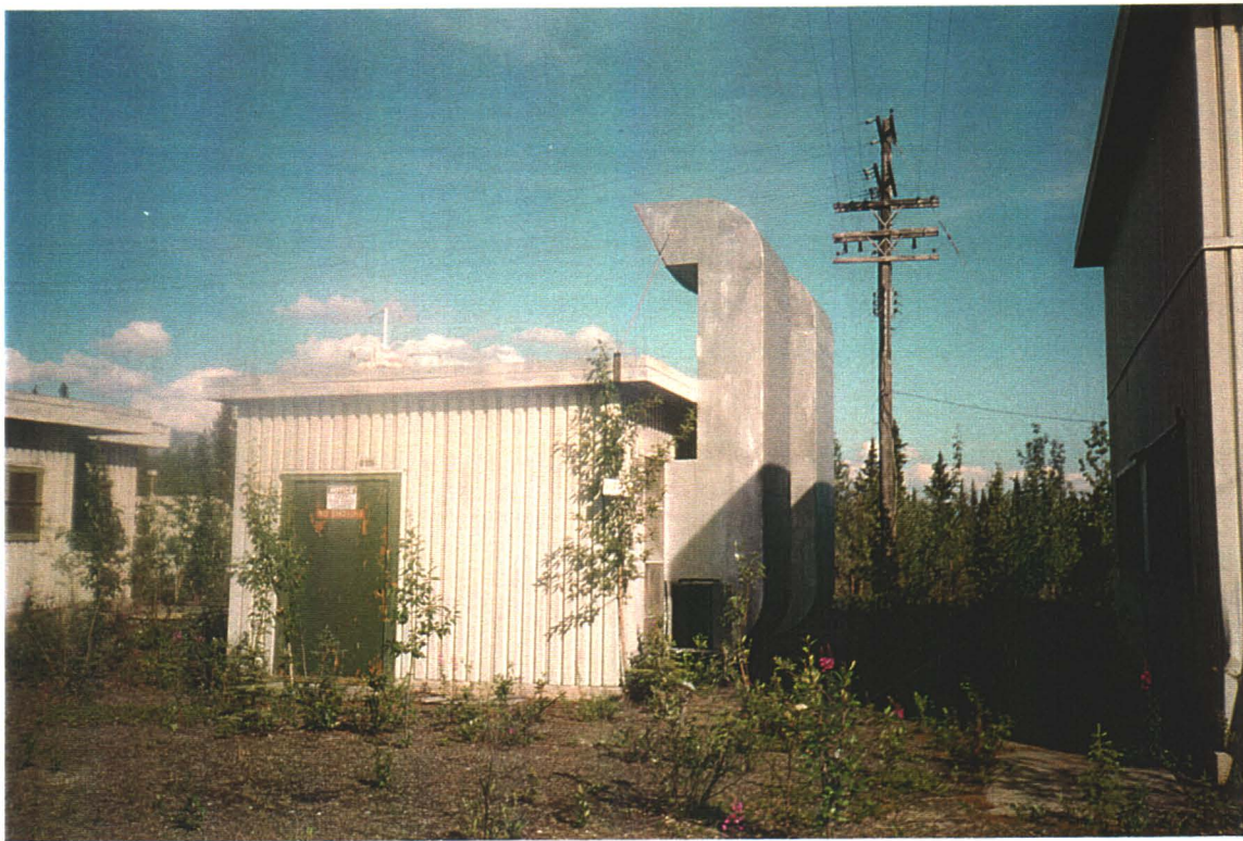
Air Intake Building. Empty, no environmental concern.
