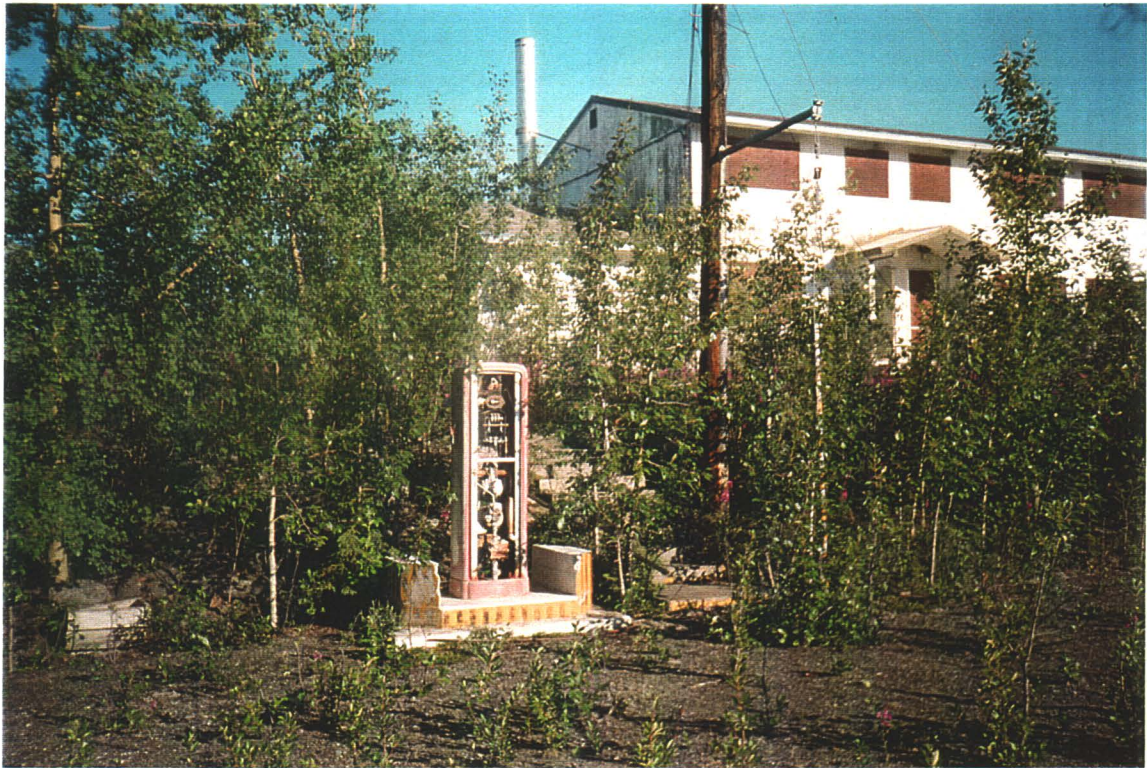
Pump island for vehicle fuel.
