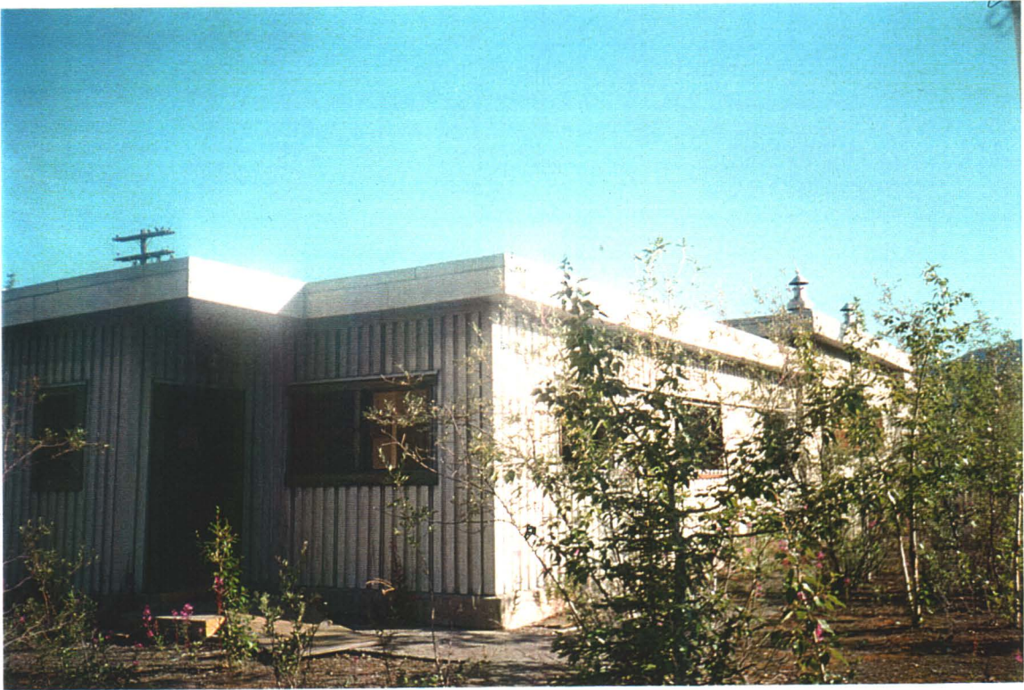
Main Building. Back side. Building is metal frame structure on concrete pad.
