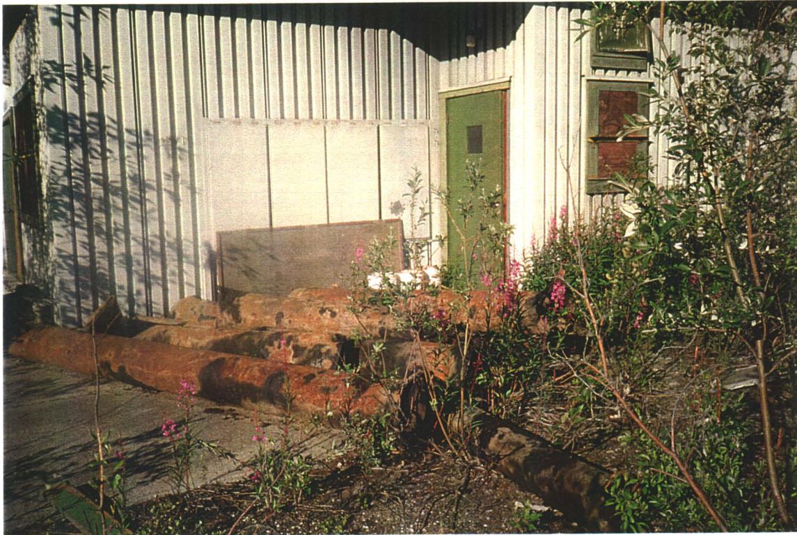
Main Building. Sections of old pipeline stored here. Contain accumulated hydrocarbon/wax deposit.
