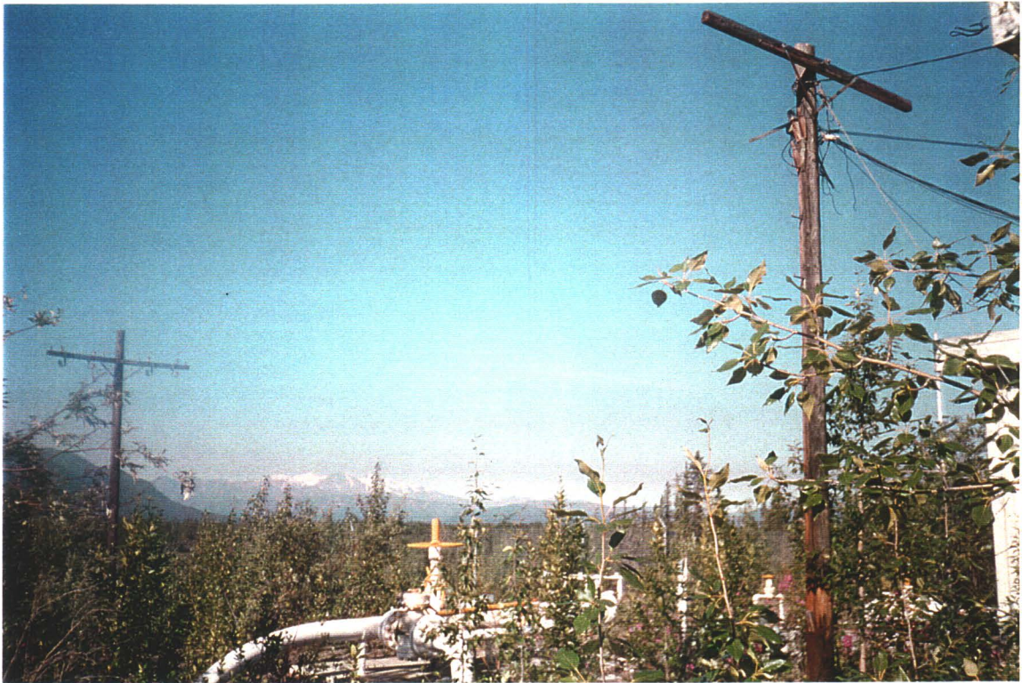
Typical power pole array, both frames. Power disconnected. No pole-mount transformers.
