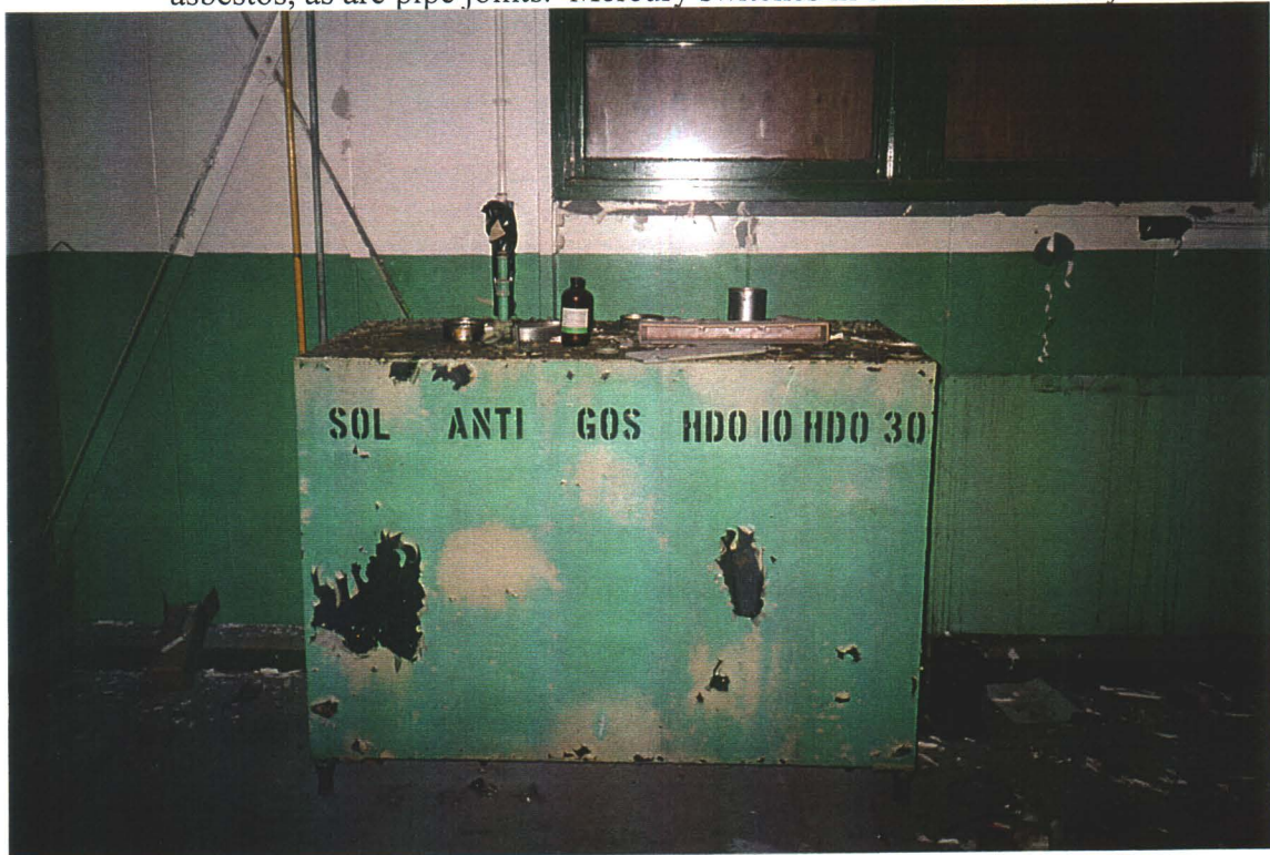
Main Building, Office Room furnace area. Interior walls are asbestos, as are pipe joints. Mercury switches in electrical circuitry.
