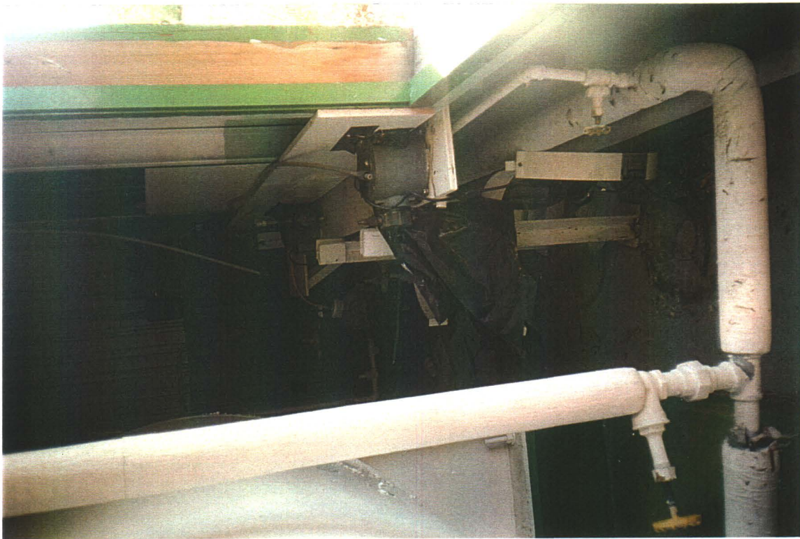
Main Building. Water Storage Room. This room houses a drained water tank and various flow metering devices and pressure system. Asbestos is present in the pipe insulation knuckle connections
