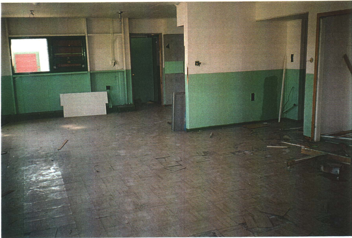
Main Building, Office Room. Note asbestos floor tiles and lead paint on walls. Interior walls are asbestos wallboard.
