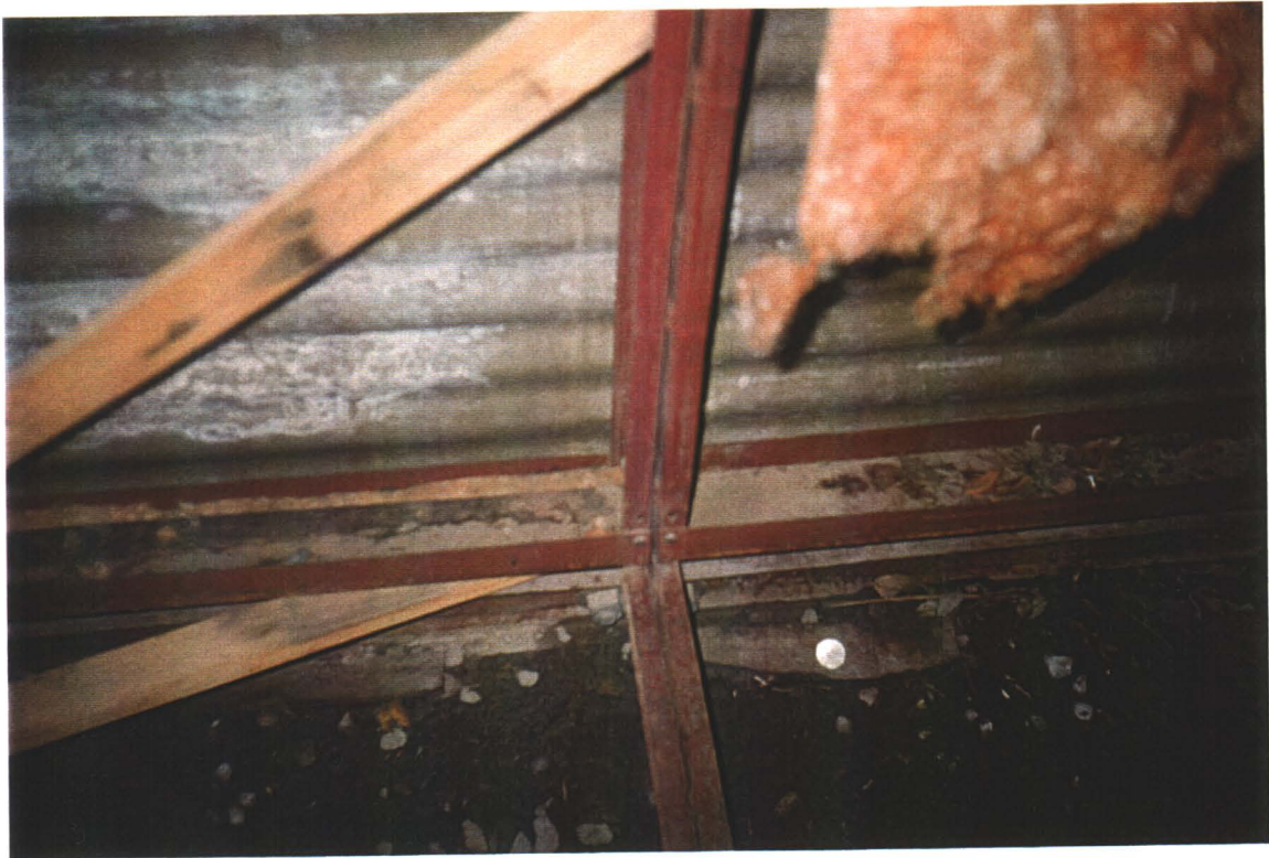
Interior of Quanset. Detail of bolt-together structure.
