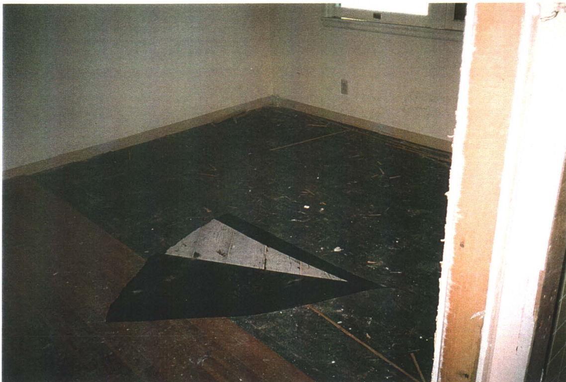
Single Residence. Interior bedroom. No evidence of asbestos on main floor.
