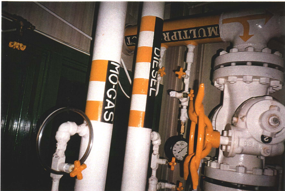
Compressor Room. Details of piping systems. Lines enter from outside, fuel is compressed and lines return to the outside. Lines are currently empty
