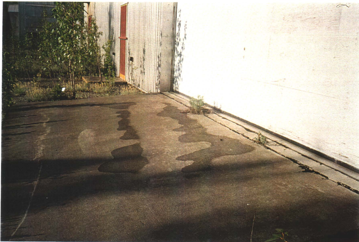
Mechanical Room/Shop. Over-head door, with concrete apron.
