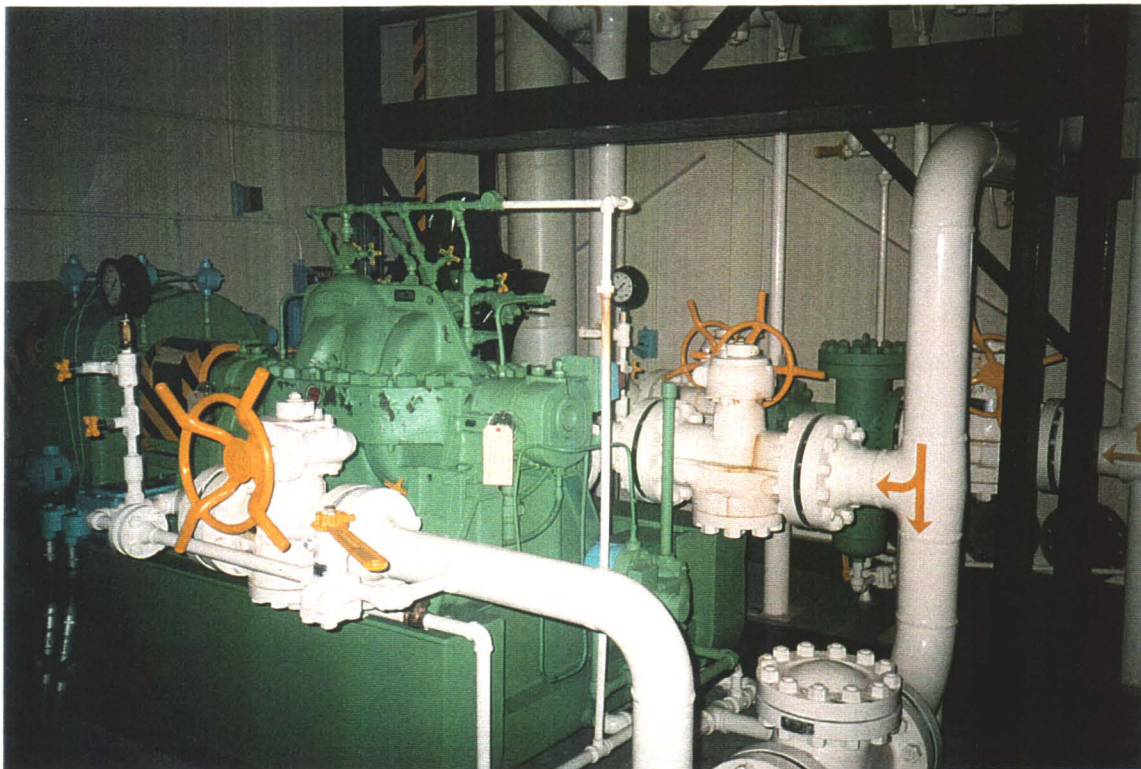
Compressor Room. Two compressor units, both drained and filled (for storage) with P-9 light oil. (note: all lead-based paint in this room)
