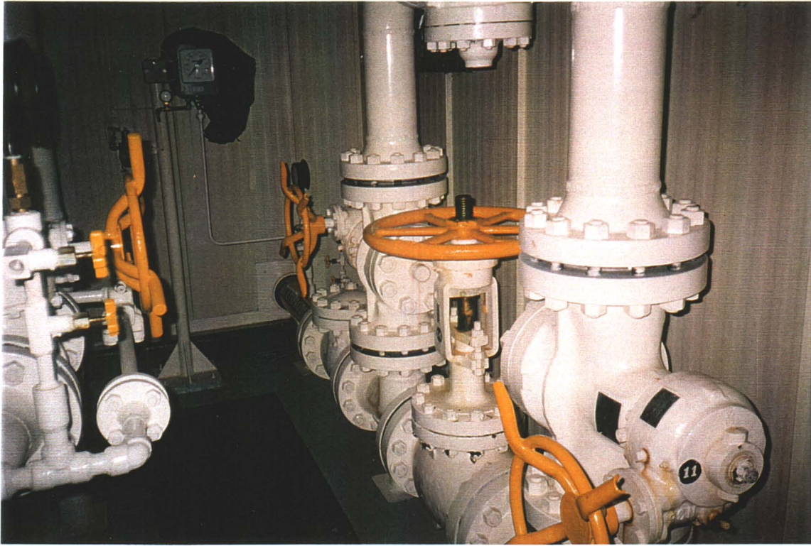
Compressor Room. Details of piping systems. Lines enter from outside, fuel is compressed and lines return to the outside. Lines are currently empty
