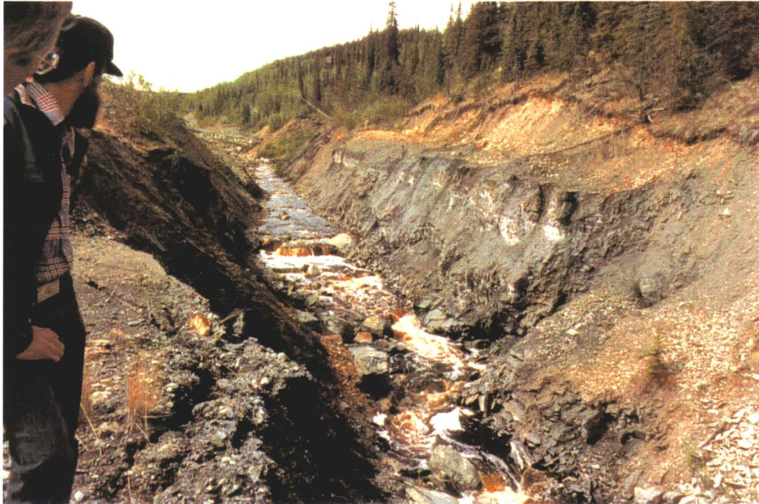
Photo 4: Channel Erosion Downstream of Weirs (1983)
