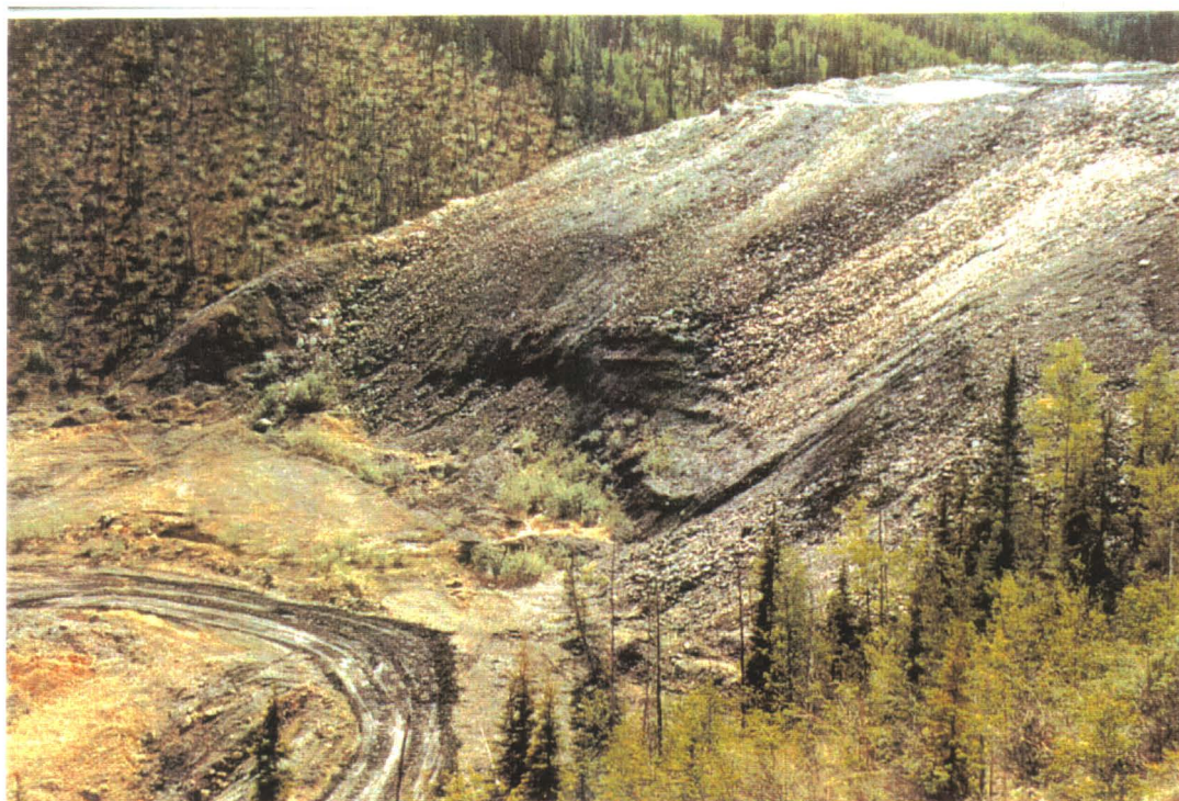
Photo 13: Outlet and Drainage Ditch on North Waste Rock Slope (1988)
