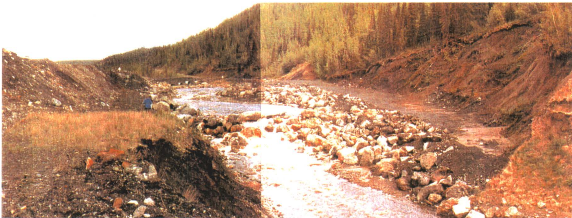
Photos 3 and 4: Channel repairs (1985)
