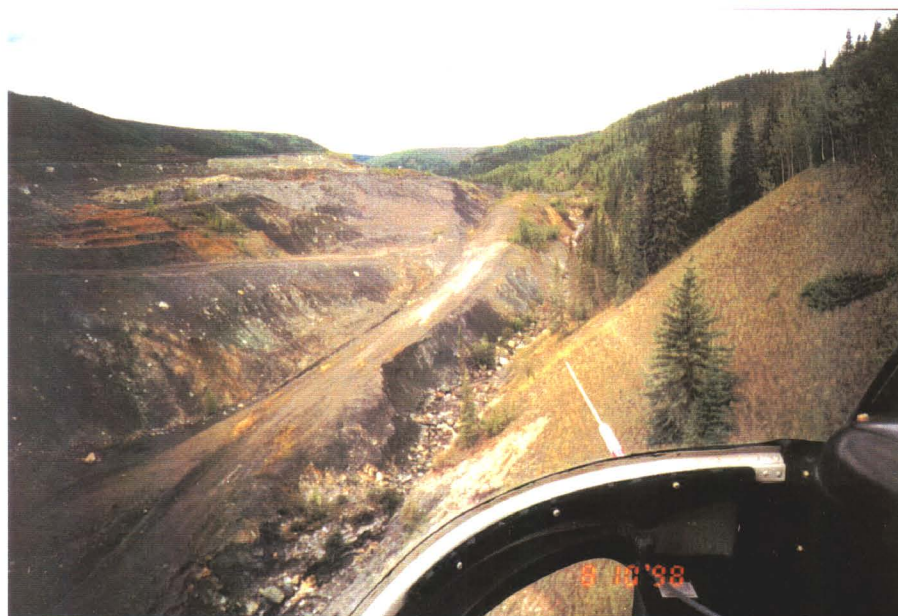
UMA Photo 2-8: Failure Along Access Road Shoulder (1998)
