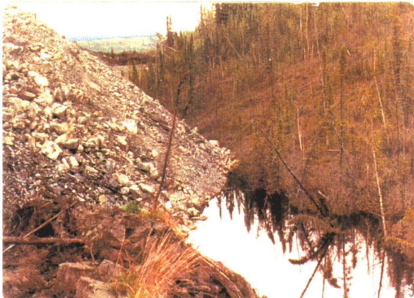
Photo PC-01: View Downstream at Blockage 2 (1975)
