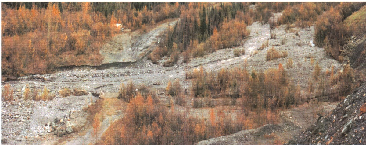
UMA Photo 13-17 and 13-18: Clinton Creek at washed out bridge
