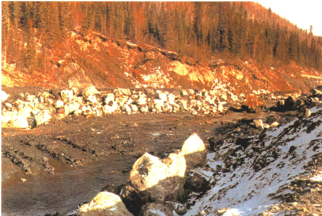
Photo 7: Armouring of North Side of Channel (1983)
