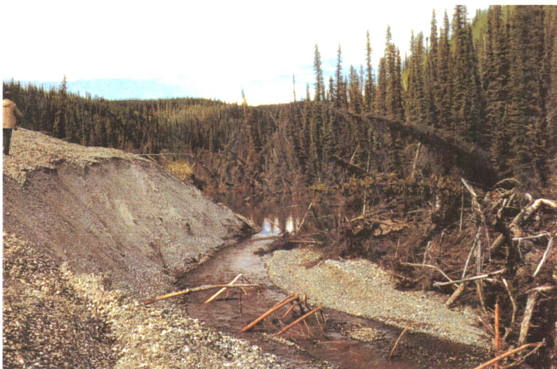
Photo 19: Erosion of Toe of North Lobe and Heaved Valley Floor (1988)
