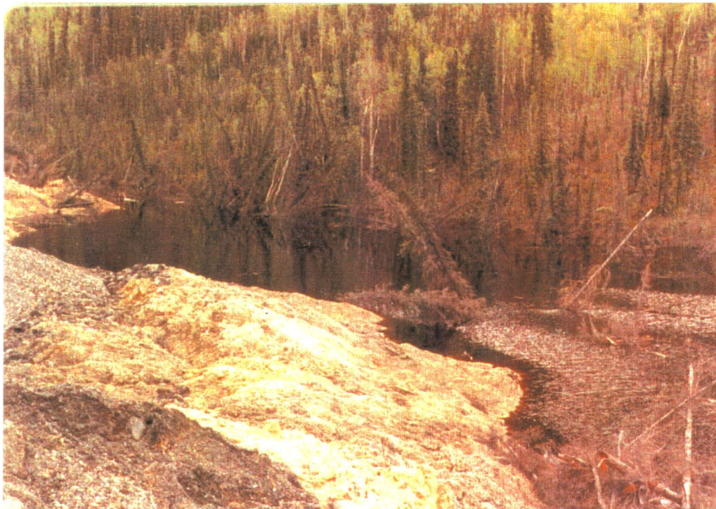
Photo PC-03: Till Up-Thrust at Toe of Failed Waste Rock (1975)
