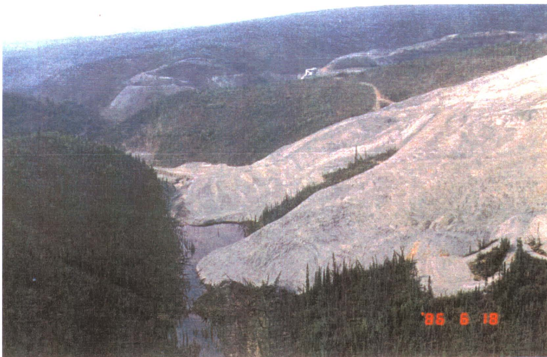
Photo 8: Toe of North Lobe Approaching Valley Slope (1986)
