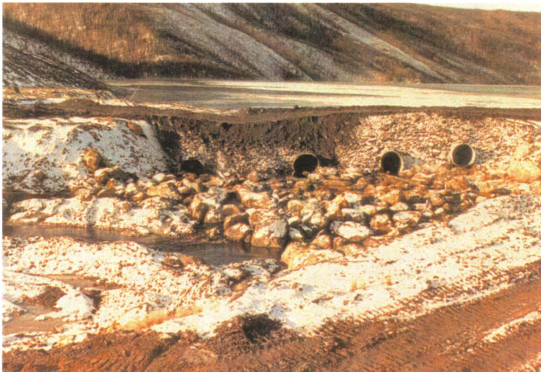
Photo 10: Channel Lining at Culvert Outlets (1983)
