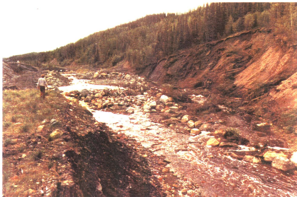
Photo 2: Channel Bypassing Rock Weirs (1984)
