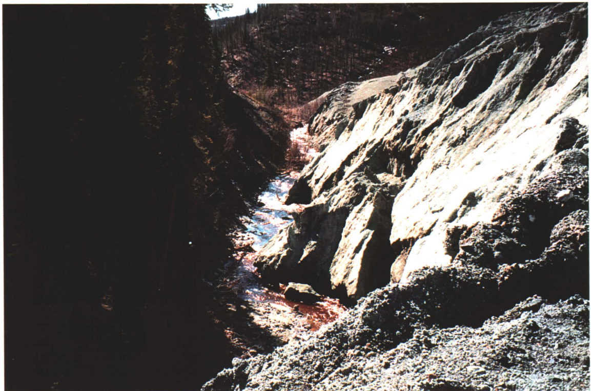
Photo F: Eroding toe of tailings and east bank of Wolverine Creek
