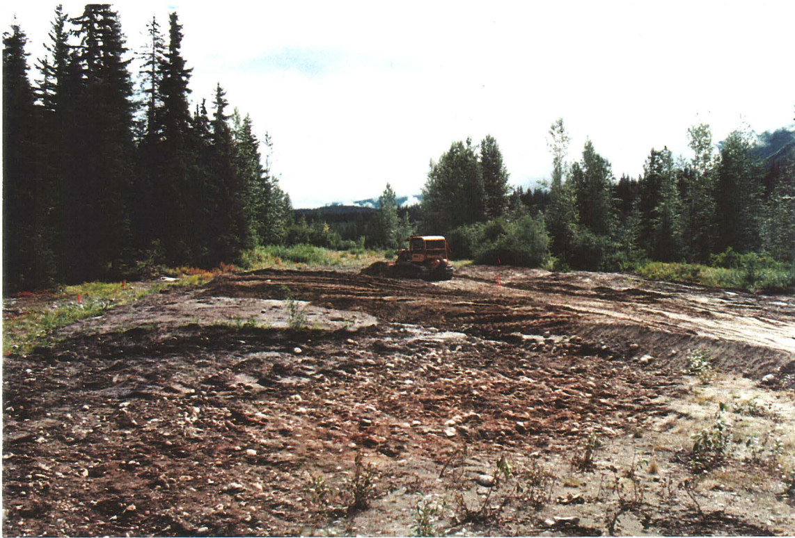
Photograph 2: Excavated area near the Trench at Rainy Hollow looking east
