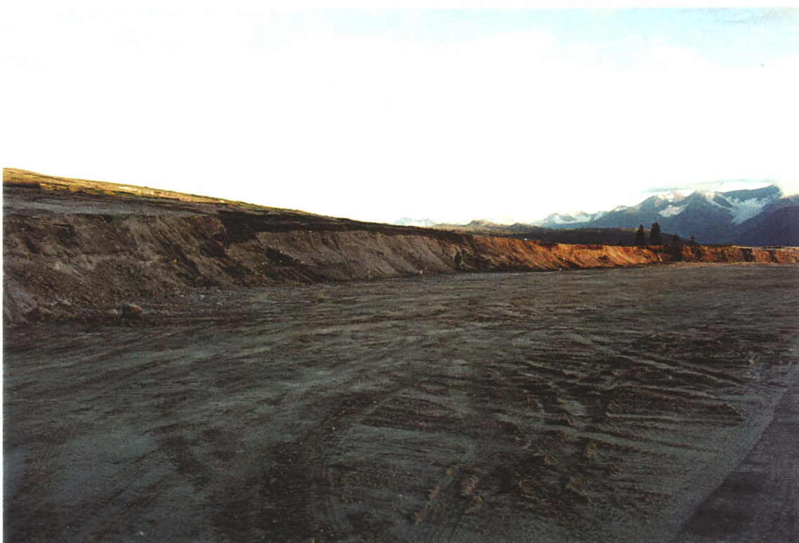
Photograph 4: Gravel borrow area after removal of material and prior to final landscaping
