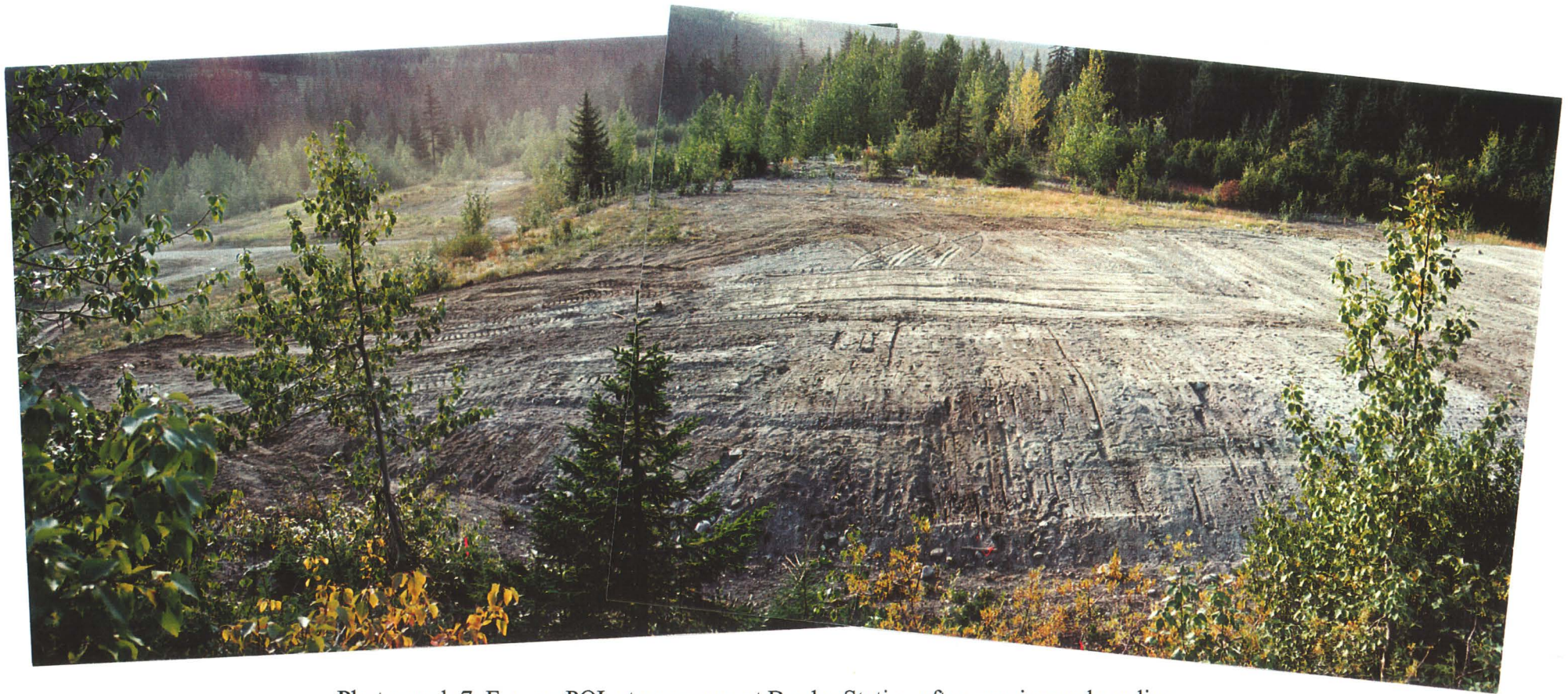
Photograph 7: Former POL storage area at Border Station after capping and grading
