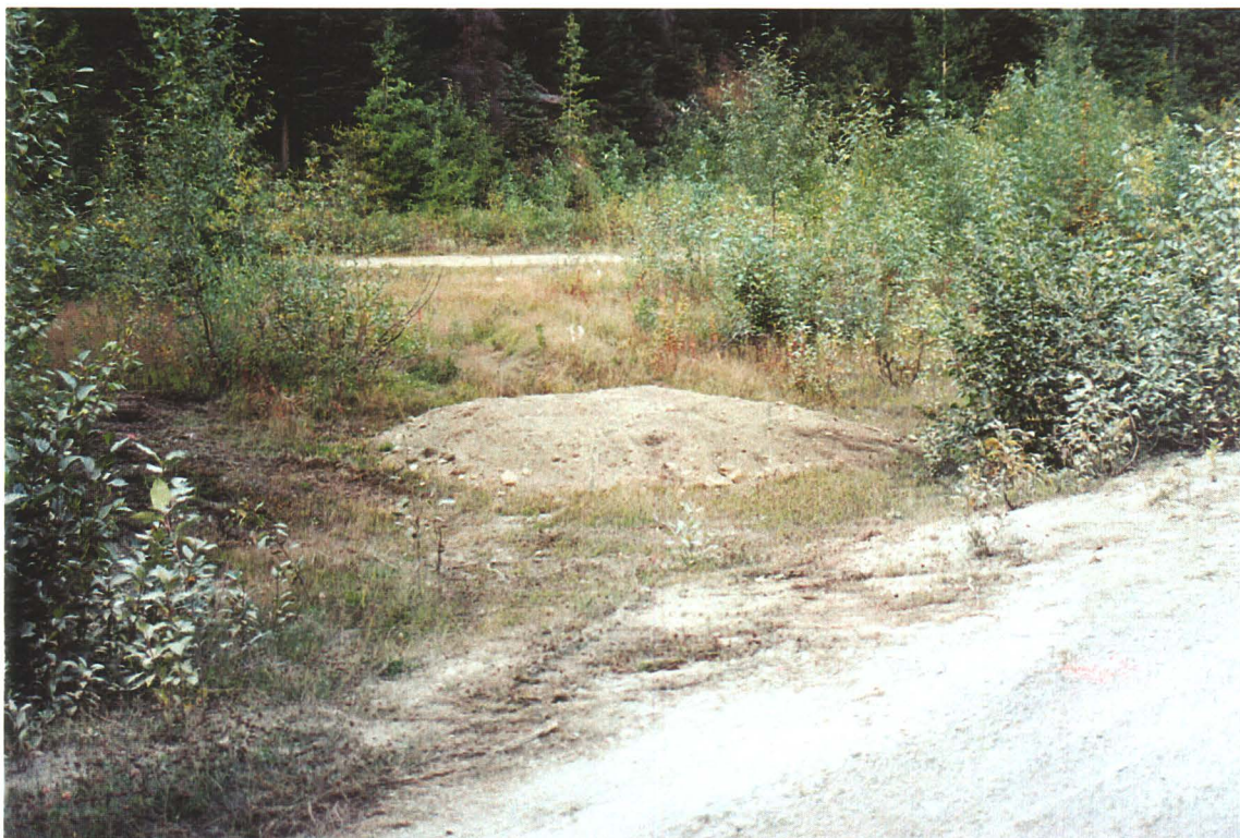
Photograph 3: Depression near the entrance of the road leading to the Temporary Storage Facility (M14) after the excavation of DDT contaminated soil and capping with gravel
