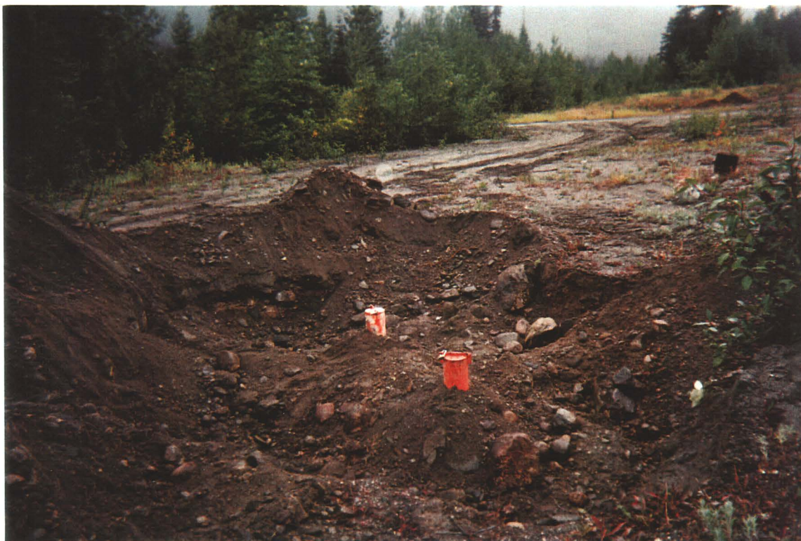
Photograph 9: Monitoring wells after modification for burial
