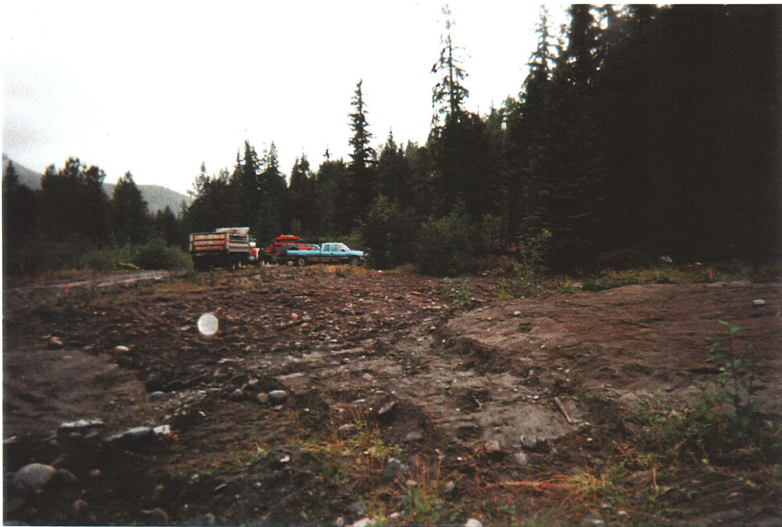
Photograph 2a: Excavated area near the Trench at Rainy Hollow looking north
