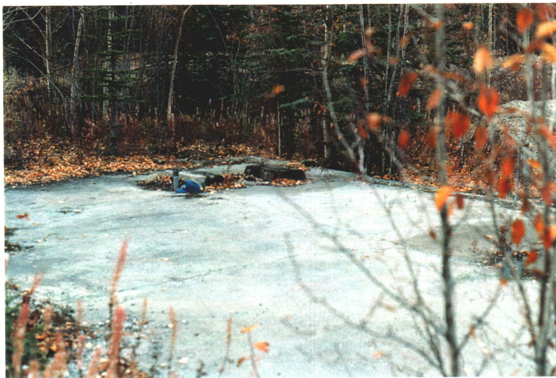
Slab foundation of generator building.
