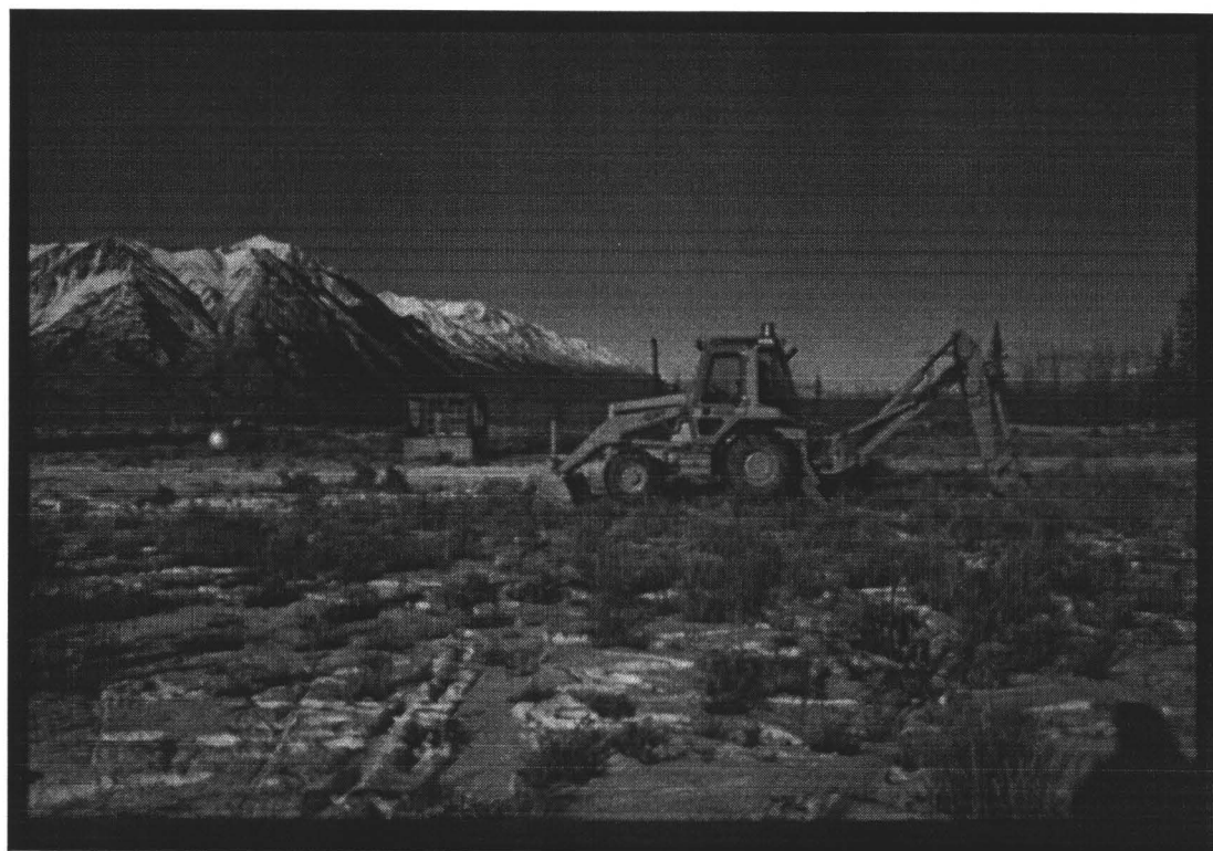
Photograph 8: GPR Site #2 from northwest corner looking northeast at Testpit #1.
