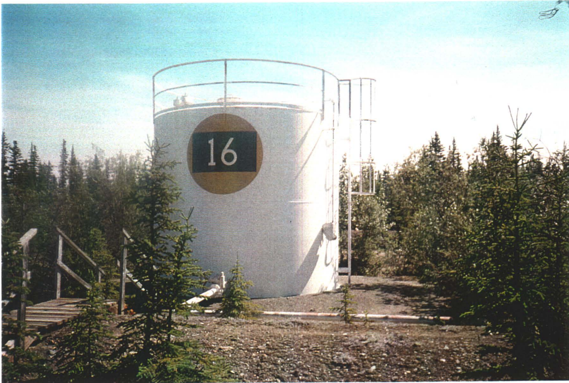
300 barrel tank, cleaned and inspected March 18, 1968
