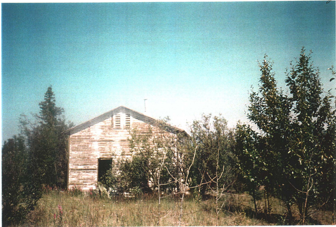
Pump House building. Exterior
