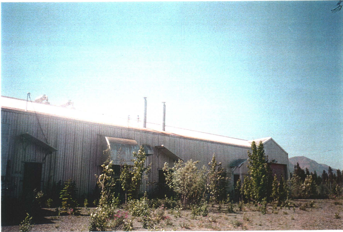
Front of main building. Note stainless steel ventilation structures, and asbestos-filled Generator Room stacks.
