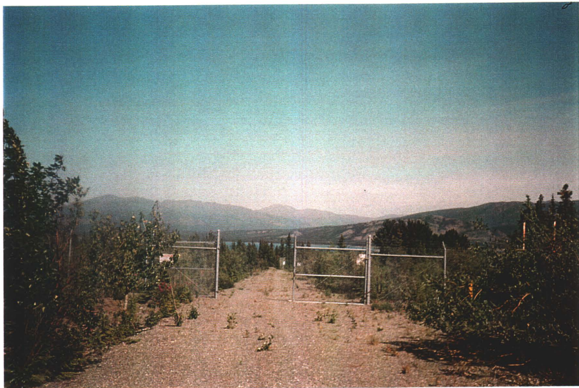
Location of two underground storage tanks and former pump island to the right of main gate.
