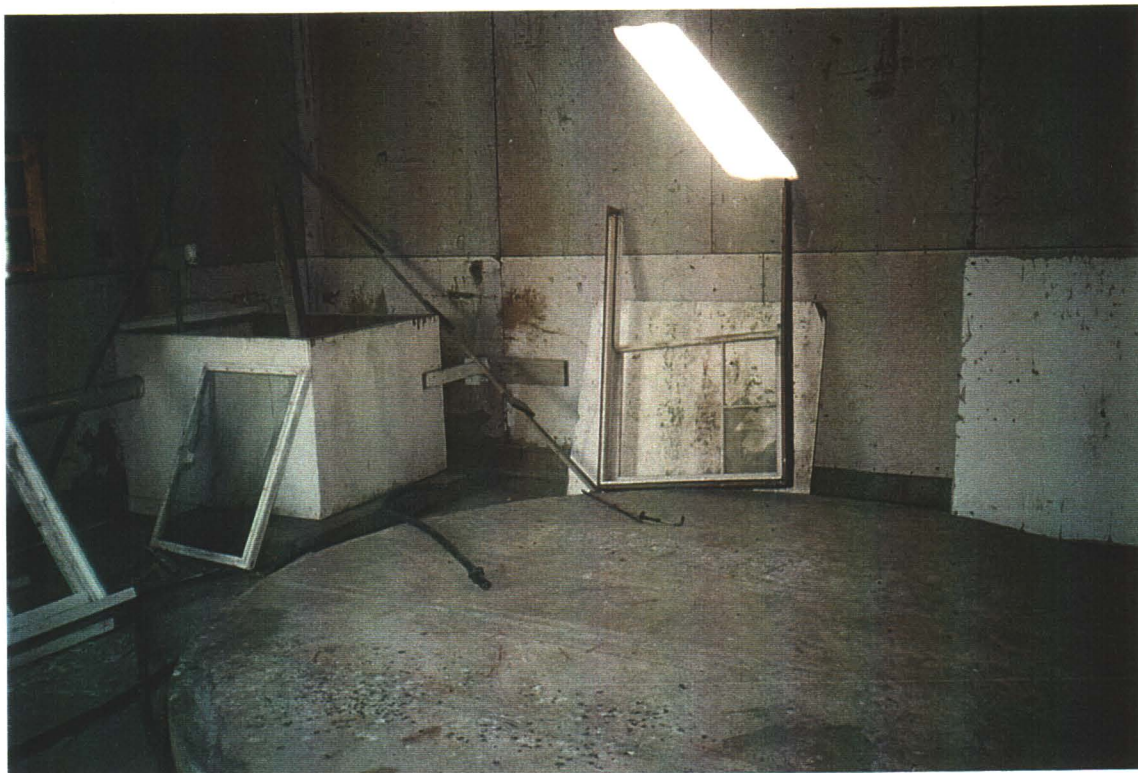
Pumphouse Building interior. Note significant concrete pad structure.
