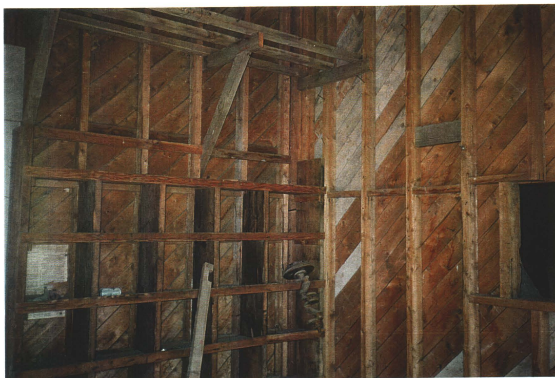
Pump House interior. Detail of wooden siding.
