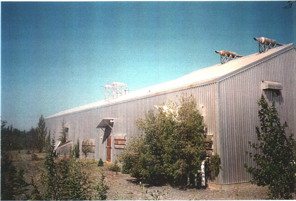
Main Building. Pipeline entry/exit lines.
