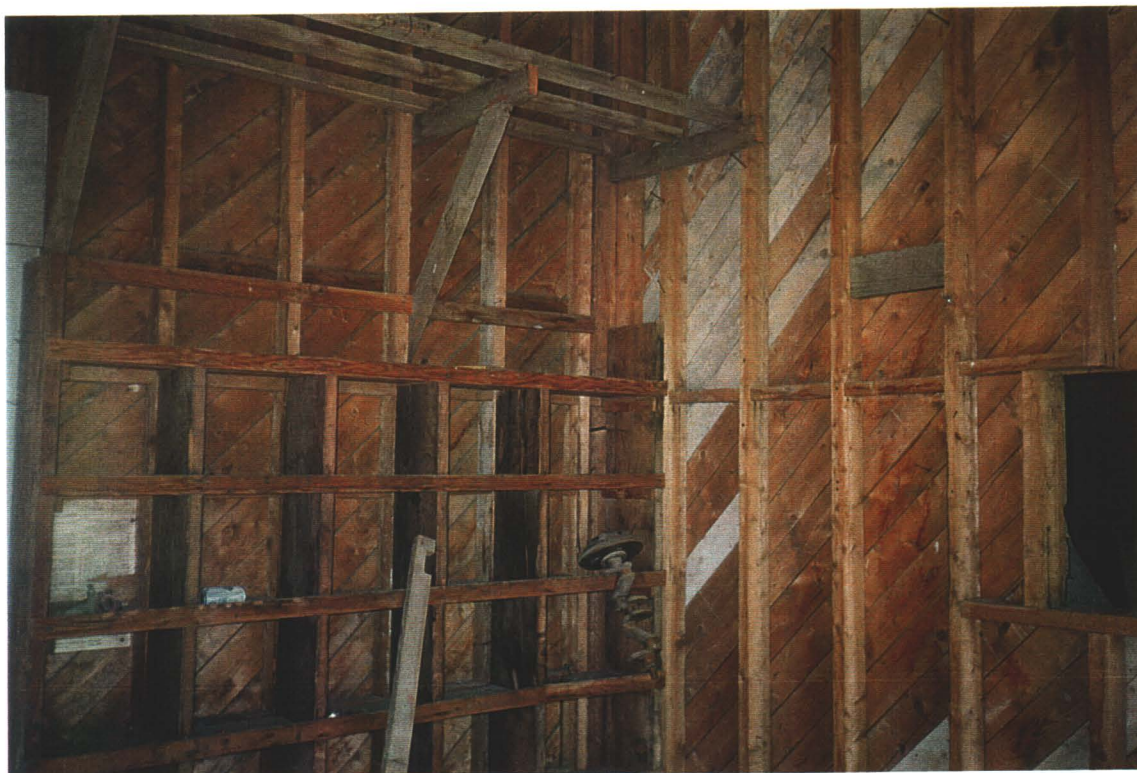
Pump House interior. Detail of wooden siding.
