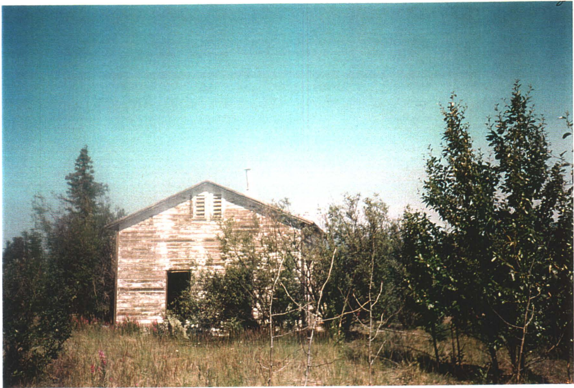
Pump House building. Exterior
