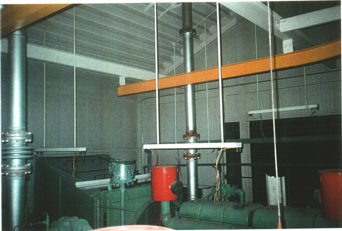
Engine Room. Typical building metal siding/roof structure.
