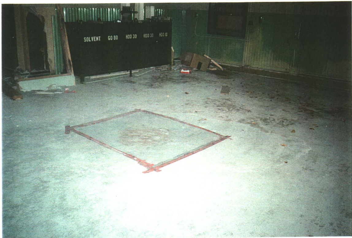
Mechanical Room/Shop. Concrete floor, with sealed sump.
