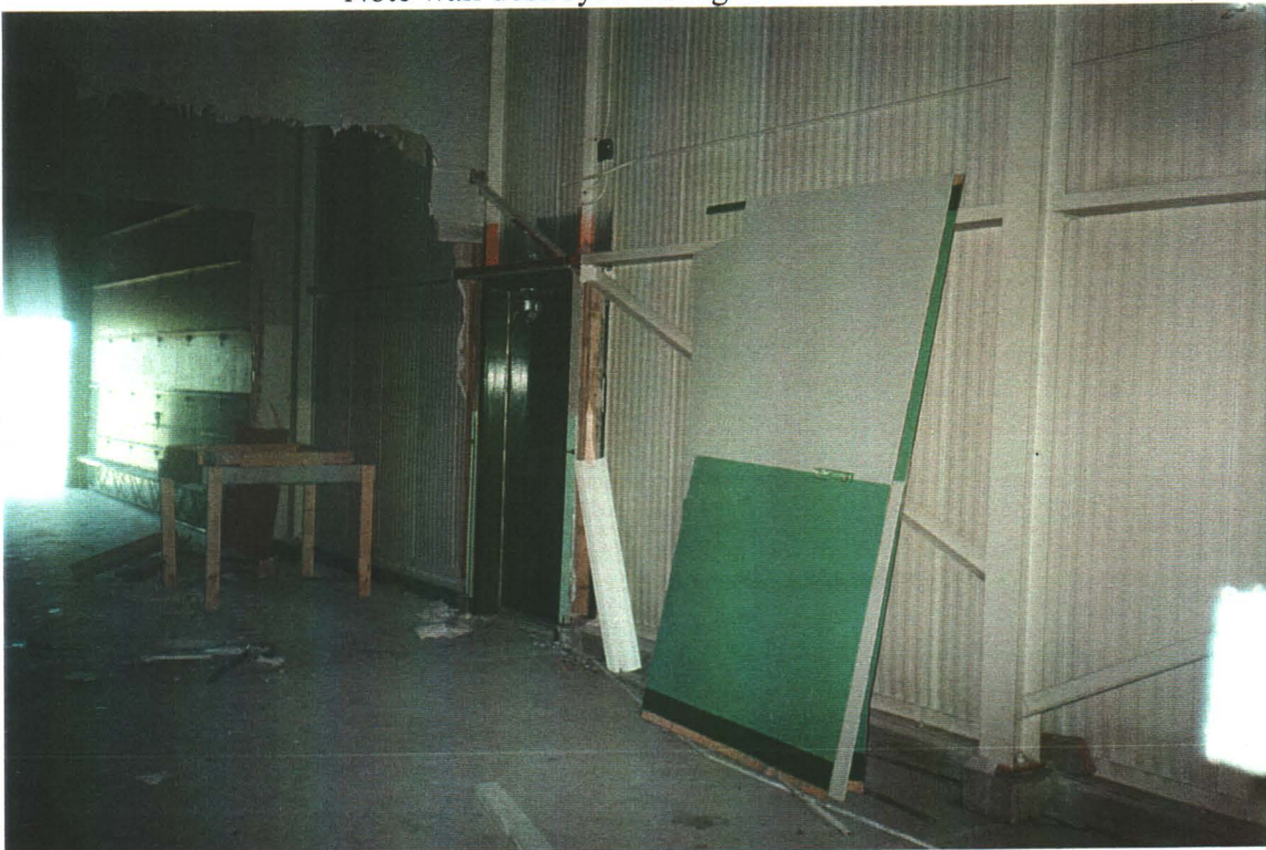
Store Room. Former location of cold storage lockers. Note wall destroyed during locker removal
