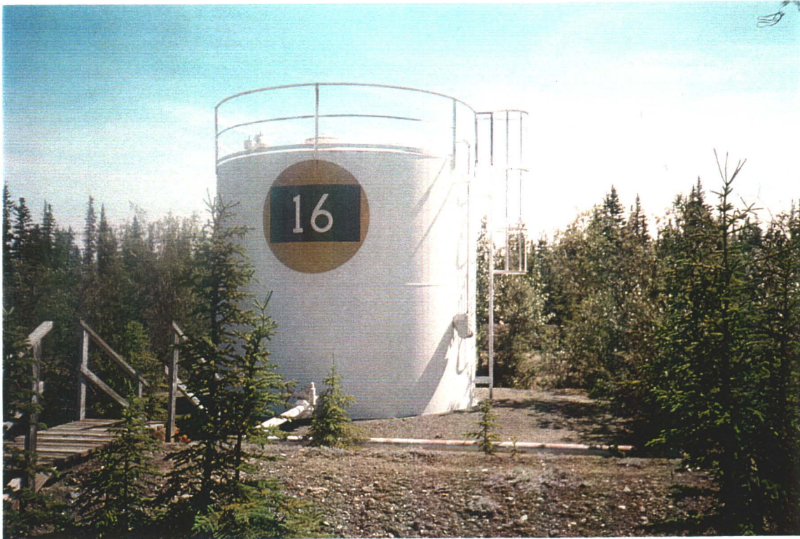
300 barrel tank, cleaned and inspected March 18, 1968
