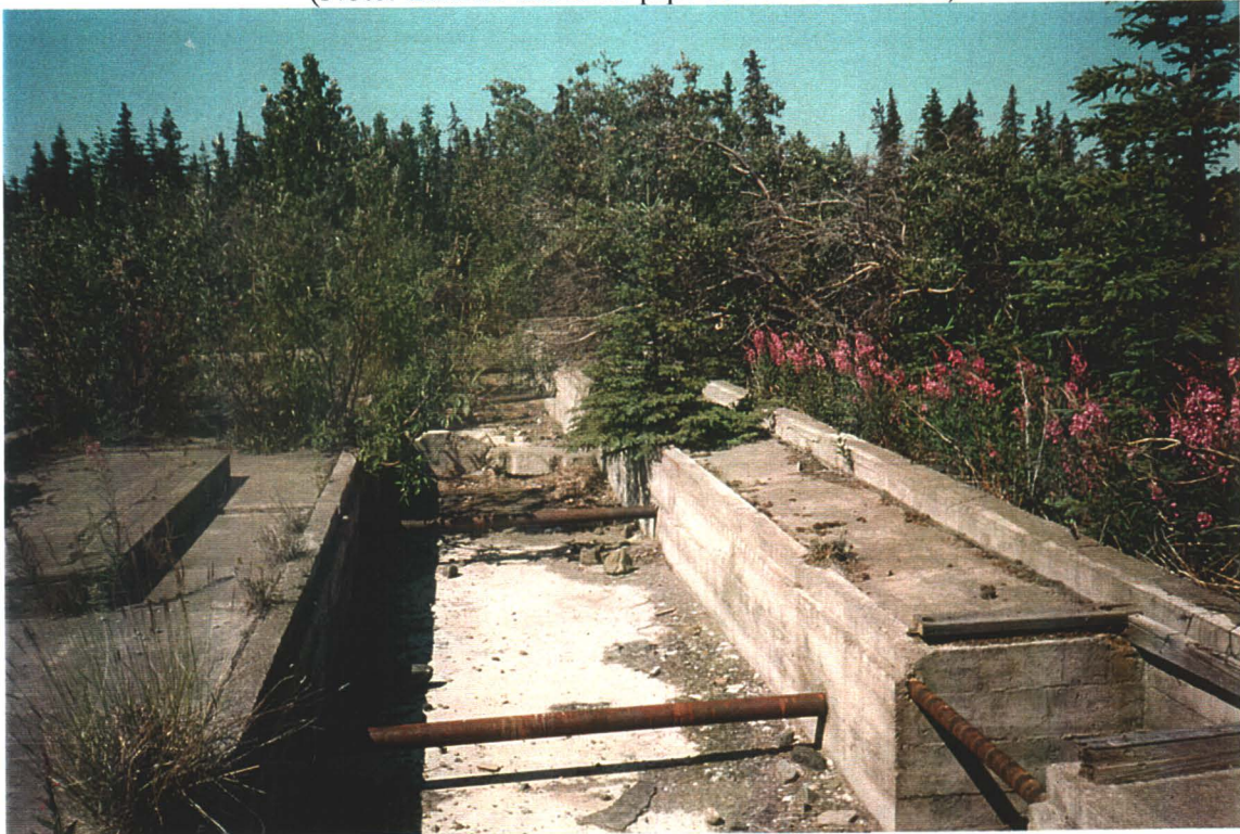
Typical services pit at each trailer stall (one of six). (Note: transite asbestos pipe sewer connection)
