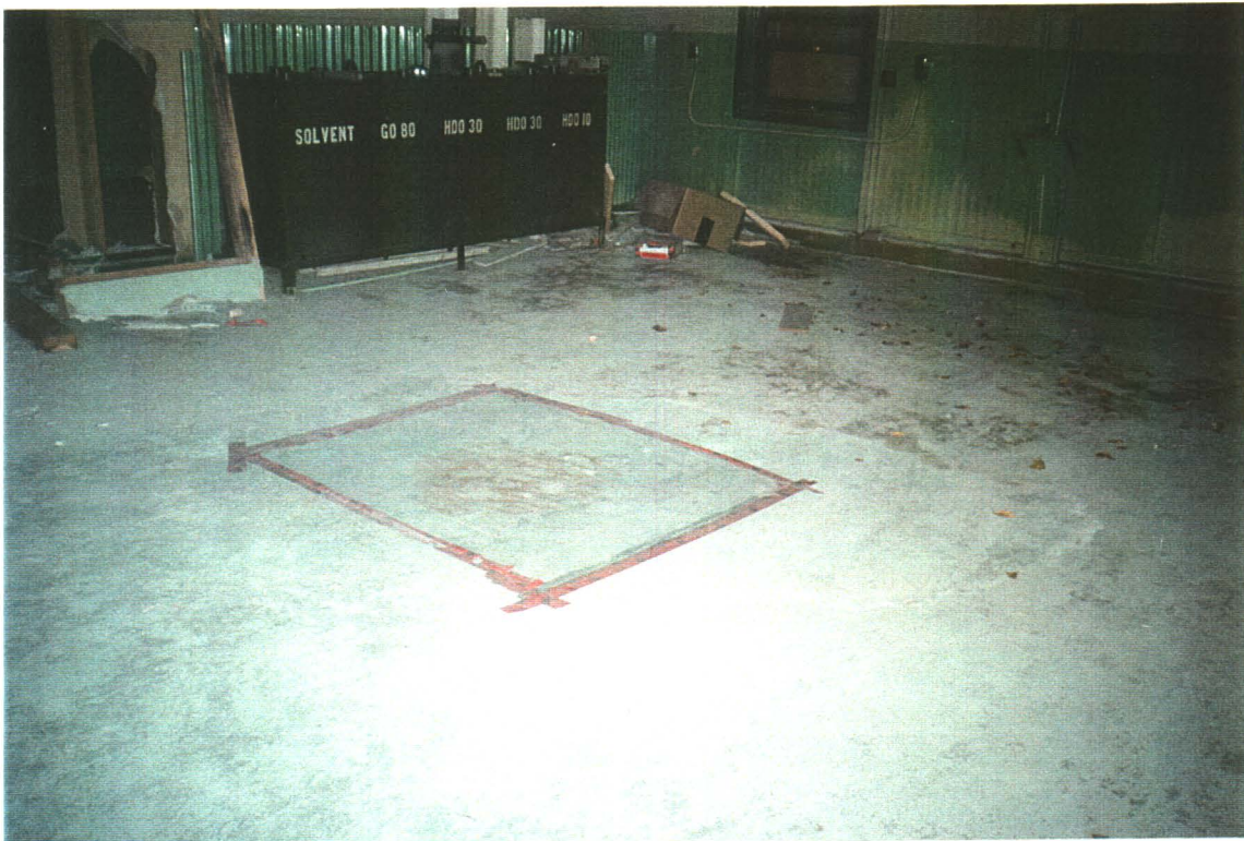
Mechanical Room/Shop. Concrete floor, with sealed sump.
