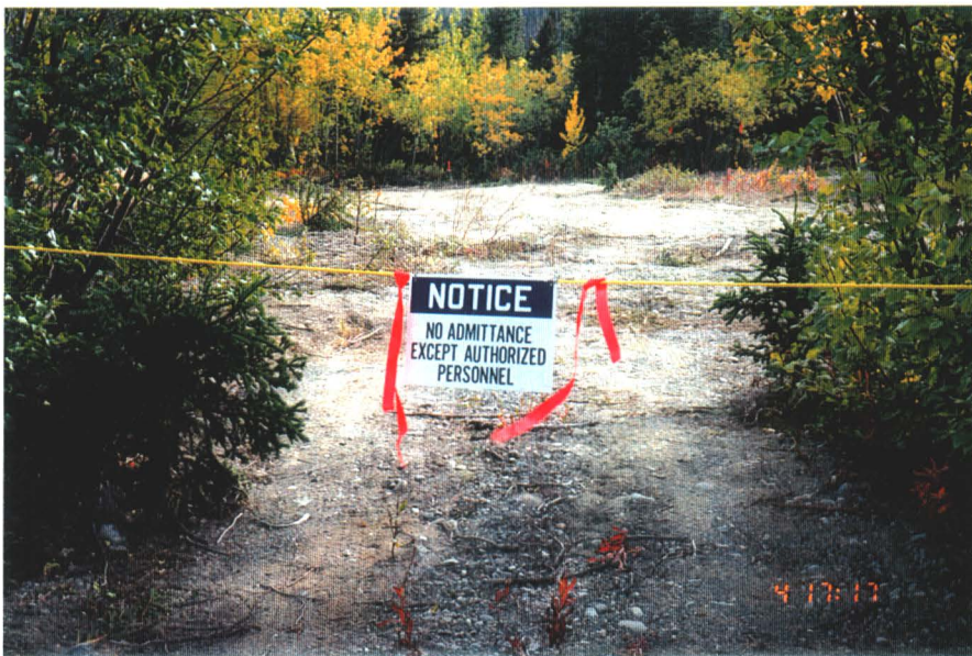
Plate 11 Perimeter was marked with nylon rope and sign
