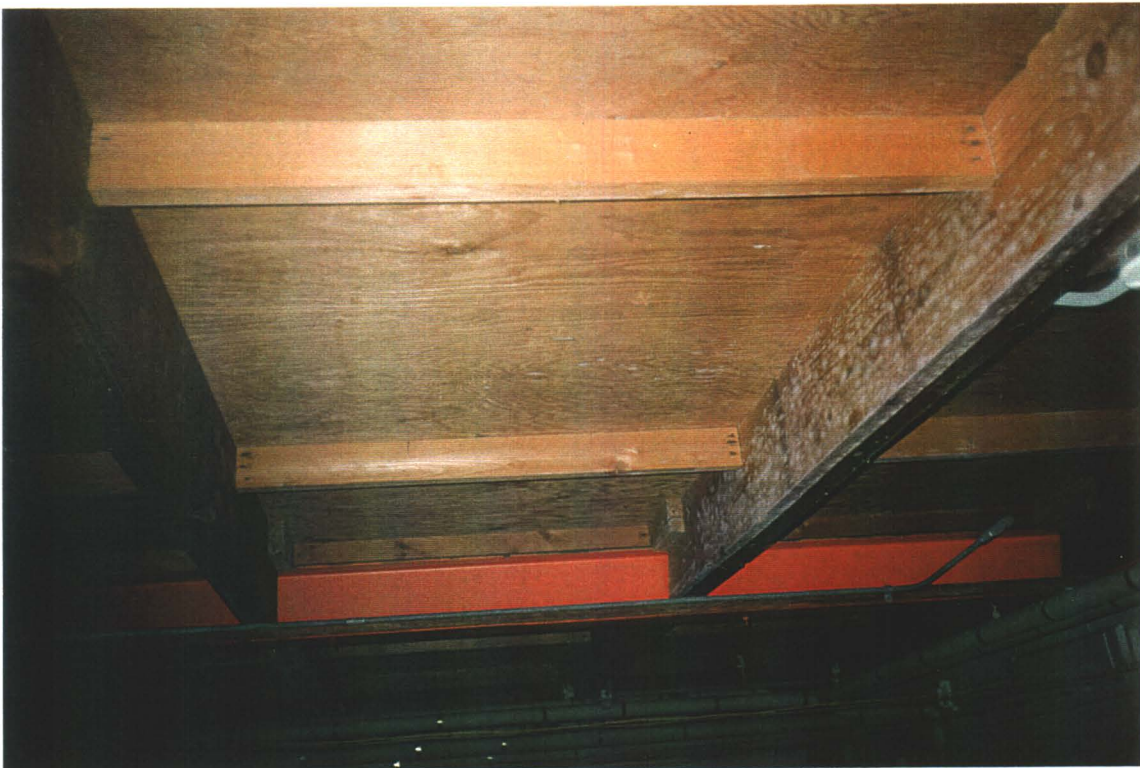
Multi-family Dwelling, basement. Note heavy beam floor system.
