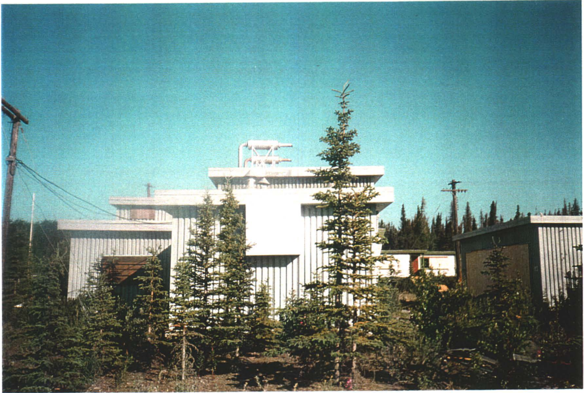
Compressor Building (high building), from back.
