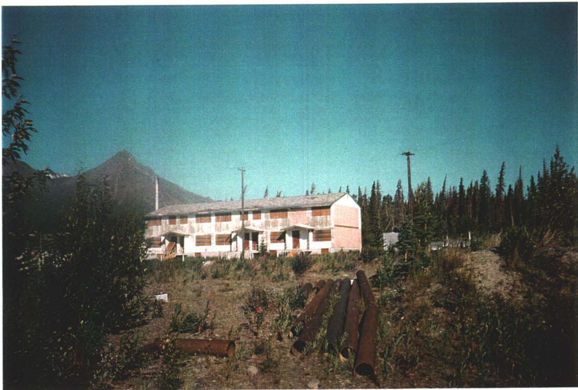
Multi-family Residence, exterior view.
