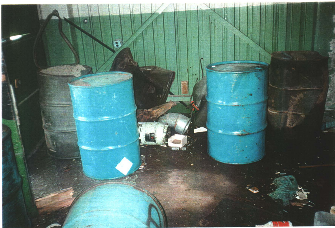
Main Building, Shop. Debris in shop, including several empty containers, one full of new oil.
