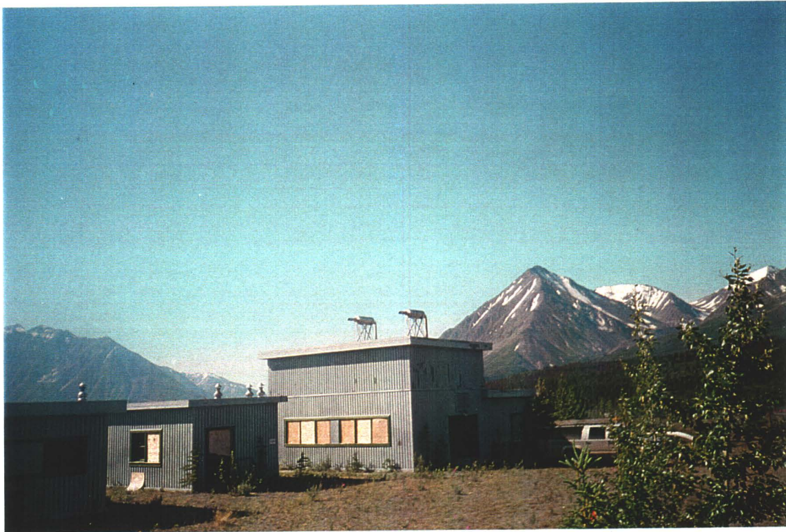
Compressor Building (high building), from front.
