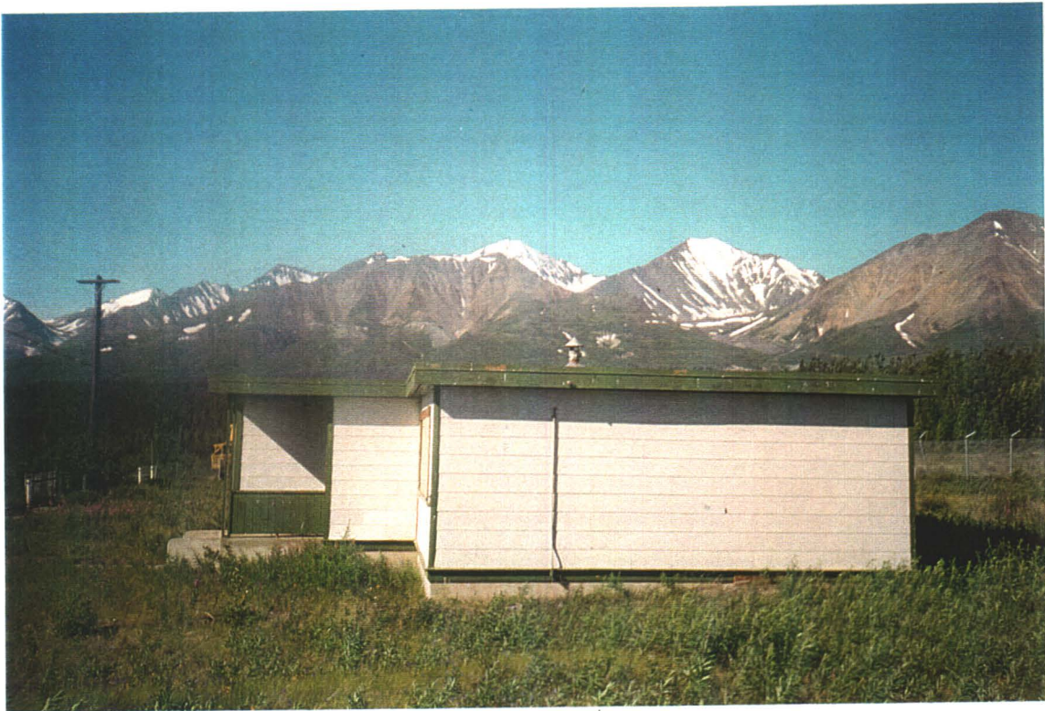
Single Residence, exterior front.
