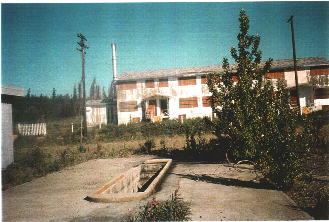
Boiler Room at left side of Multi-family Residence. Steam lines lead to this residence and facility buildings. Wooden siding, coated with lead-based paint.
