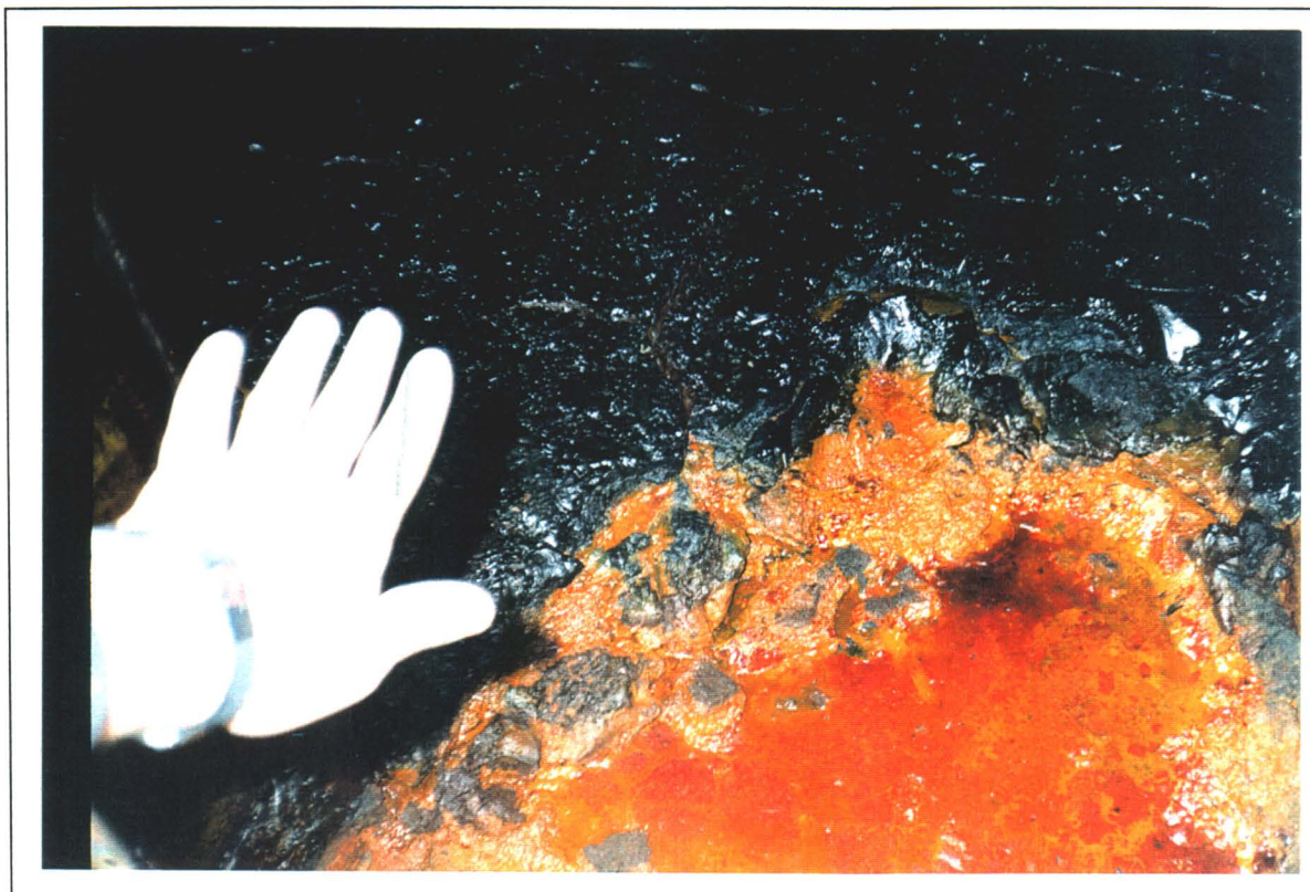
PHOTOGRAPH 8: Crude oil tars inside POL tank
