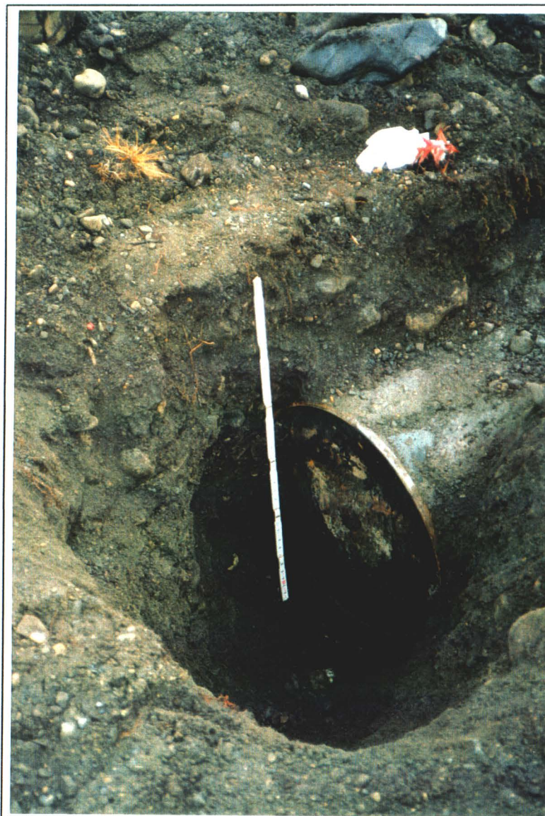
PHOTOGRAPH 10: Exposed west end of underground storage tank.
