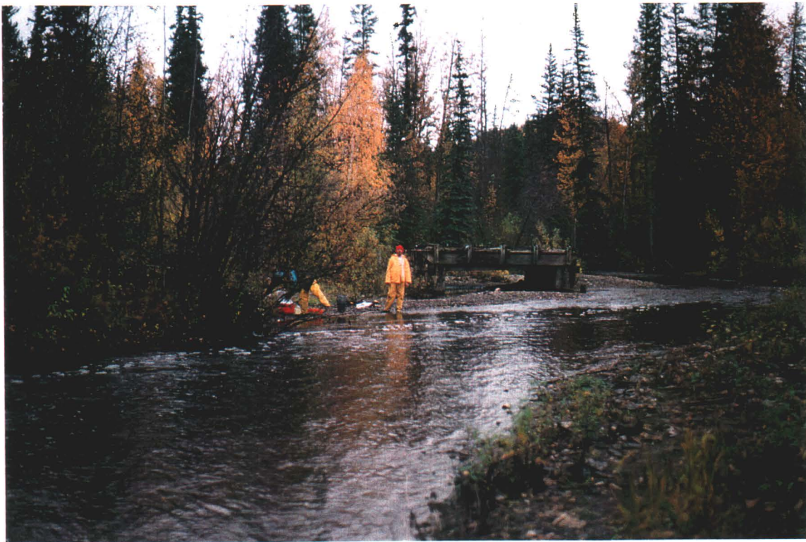
Photograph 4.3: Zone 6 looking downstream towards remnants of bridge and ford crossing to town site.
