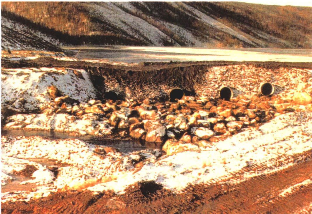
Photo 10: Channel Lining at Culvert Outlets (1983)
