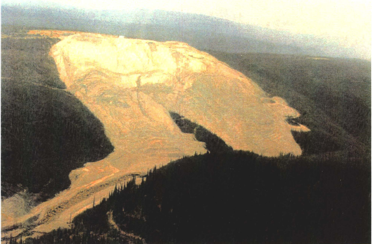
Photo 8: Failed North Lobe Near Valley Slope (1986)
