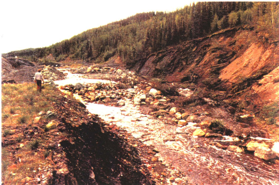
Photo 2: Channel Bypassing Rock Weirs (1984)
