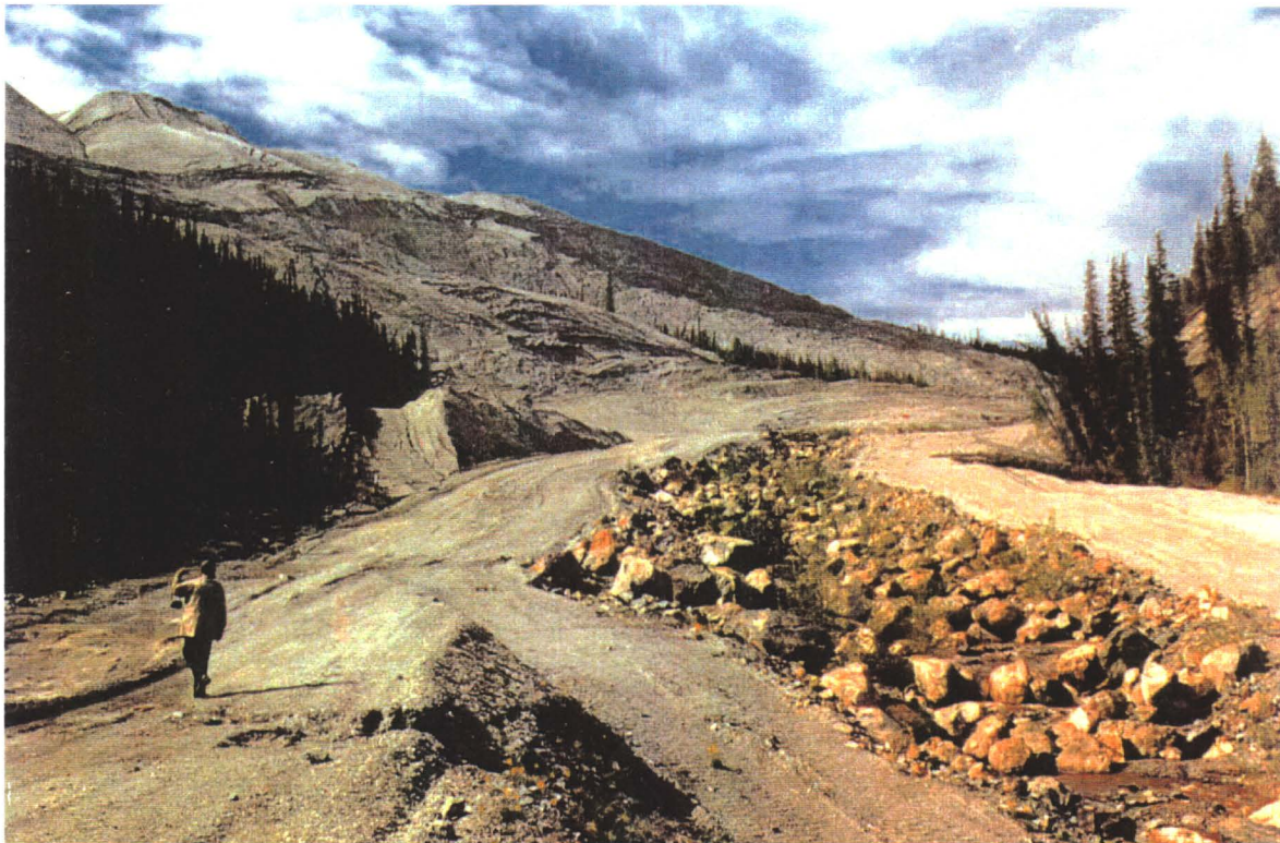
Photo 22: Armoring of Wolverine Creek Channel Downstream of the South Lobe
