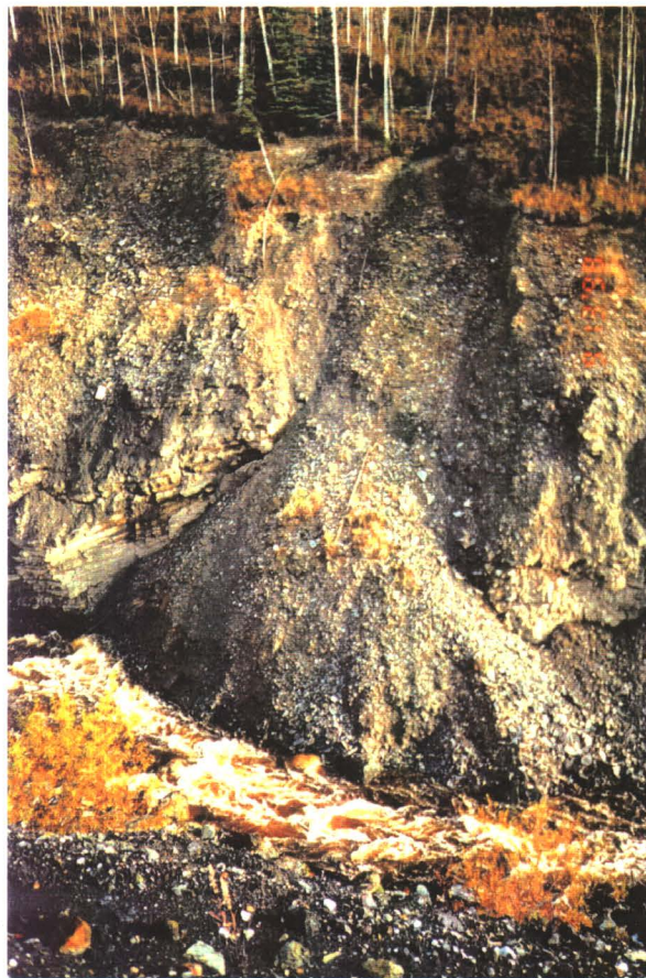
UMA Photo 7-6: Sloughed Till in Channel From Localized Bank Failure (1998)
