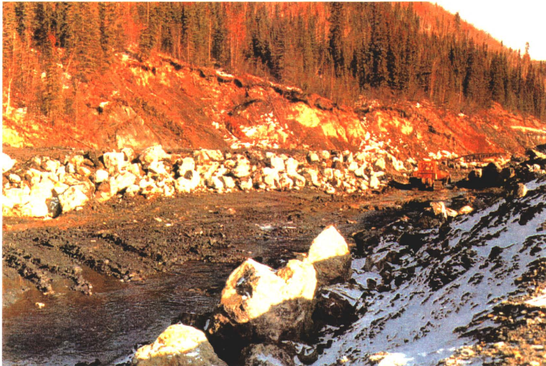
Photo 7: Armouring of North Side of Channel (1983)
