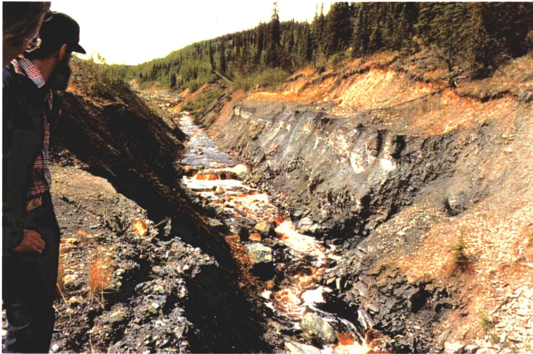
Photo 4: Channel Erosion Downstream of Weirs (1983)
