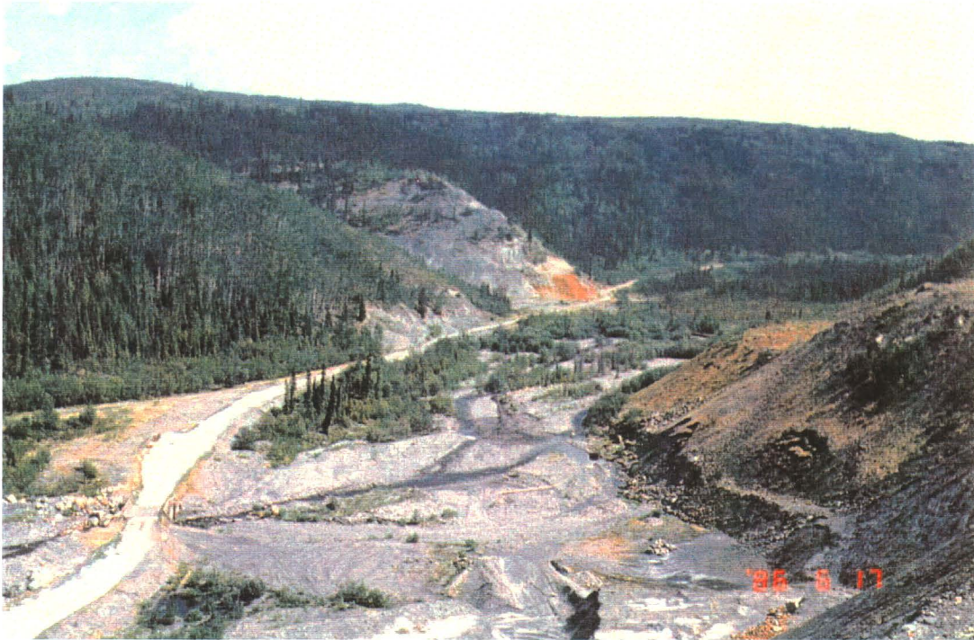
Photo 7: Clinton Creek Bridge Crossing (1986)
