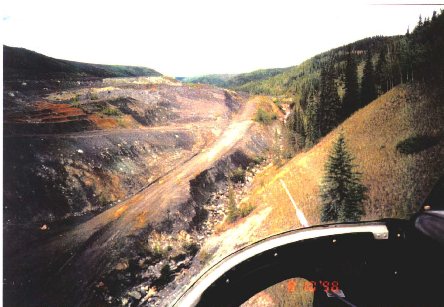
UMA Photo 2-8: Failure Along Access Road Shoulder (1998)
