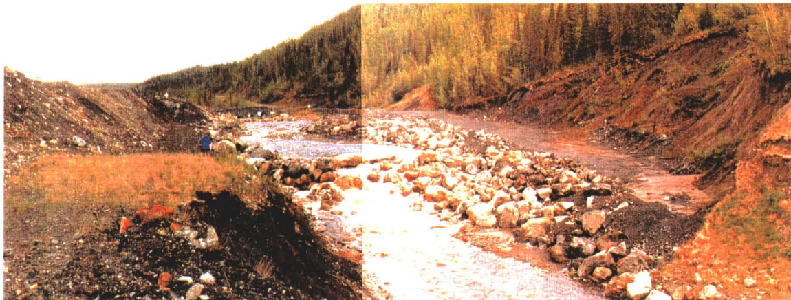
Photos 3 and 4: Channel repairs (1985)
