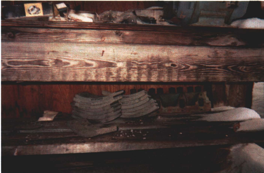
Photograph 17: Asbestos brake pads stored in maintenance building.
