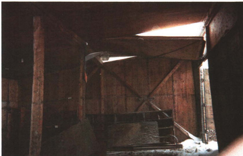
Photograph 6: Section of roof on maintenance shed that is in danger of collapse as weight of snow increases
