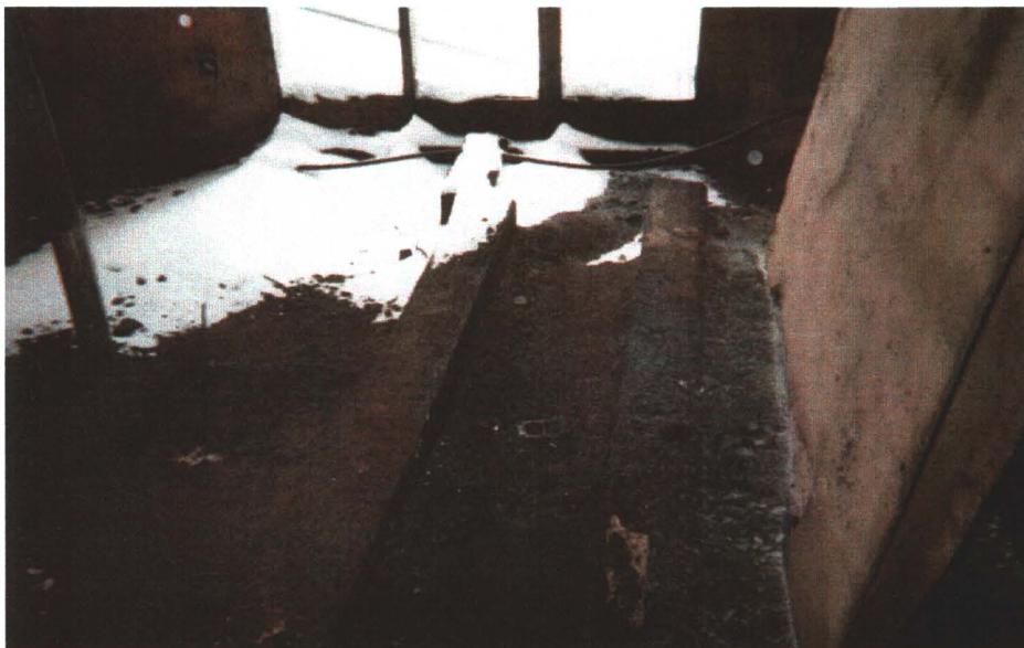
Photograph 8: Stained soil on floor of generator part of maintenance shed (Site 2 sample)
