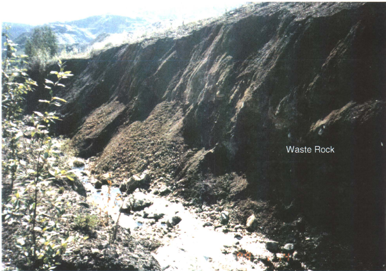
UMA Photo 14-11A Waste Rock Slumping at Sec A-AA
