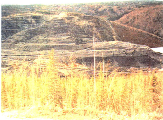
Waste Rock Dump (1977). Note Cracks in Upper and Lower Portions
