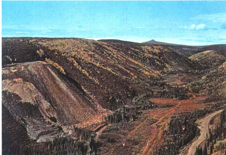
Waste Rock Dump in About 1970 (View Upstream)
