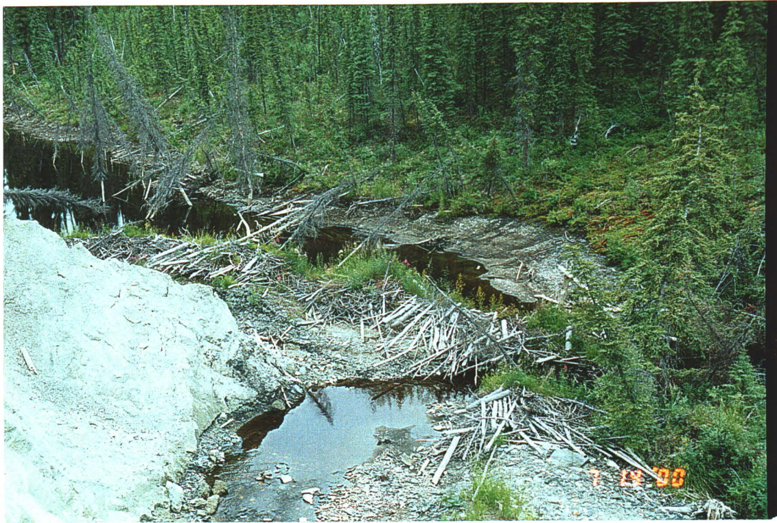
Photo 9: View of the beaver dam located at the upstream edge of the south tailings pile, uplifted by ongoing ground movements.
