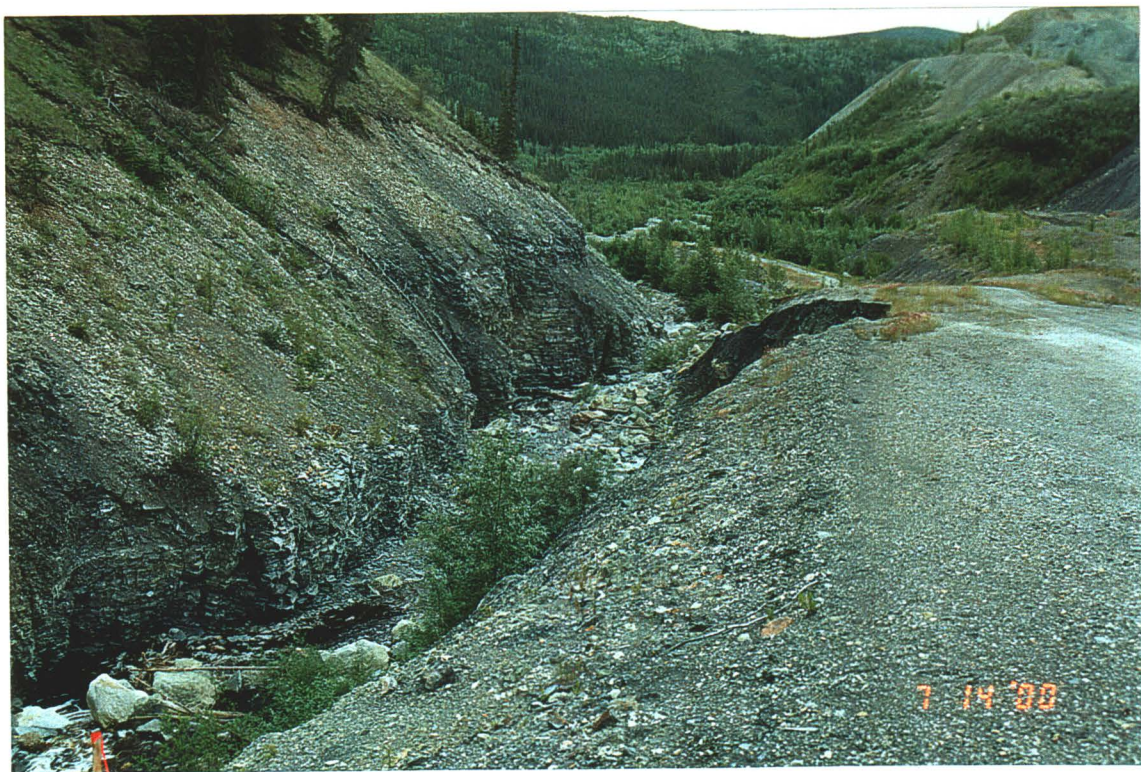
Photo 6: View of the downstream segment of the Clinton Creek channel. Note ongoing erosion of both channel banks.
