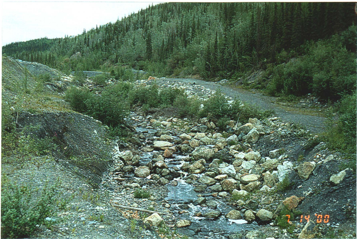
Photo 5: View of former rock weir and increased lateral erosion of both channel banks.
