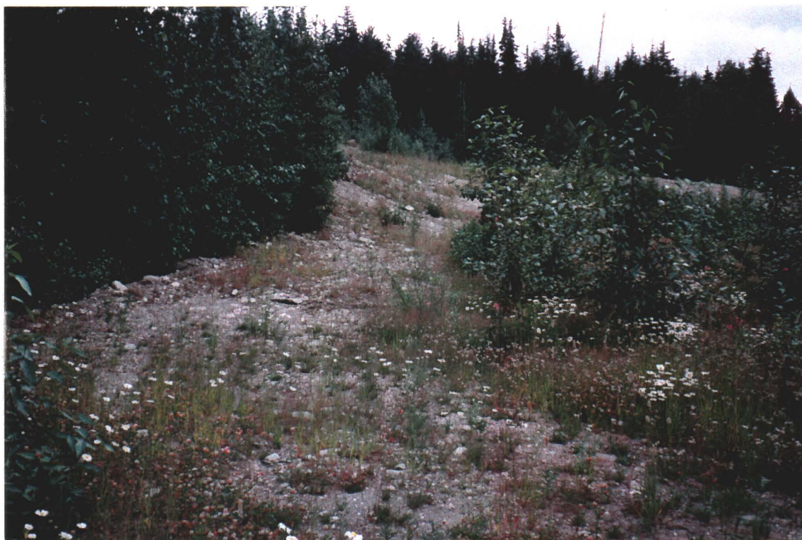
Photograph 9: Looking east along access road constructed for delivering gravel to the former POL storage area
