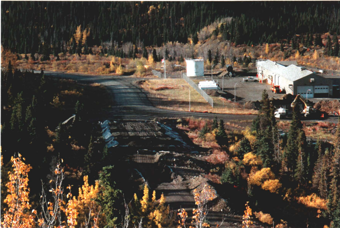
Photograph 6.6: View of the Temporary Containment Cell from Haines Highway prior to covering it with a polyethylene liner.
