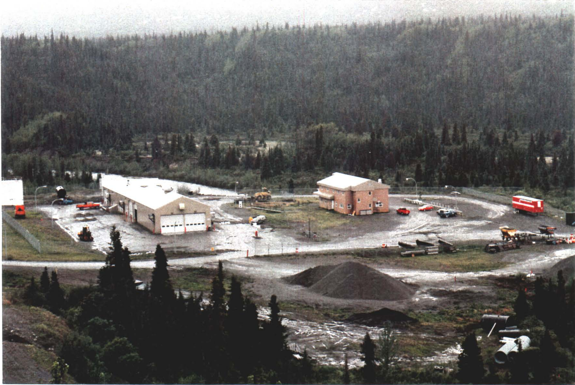
Photograph 2-2: Blanchard Maintenance Camp looking west from the Haines Highway.
