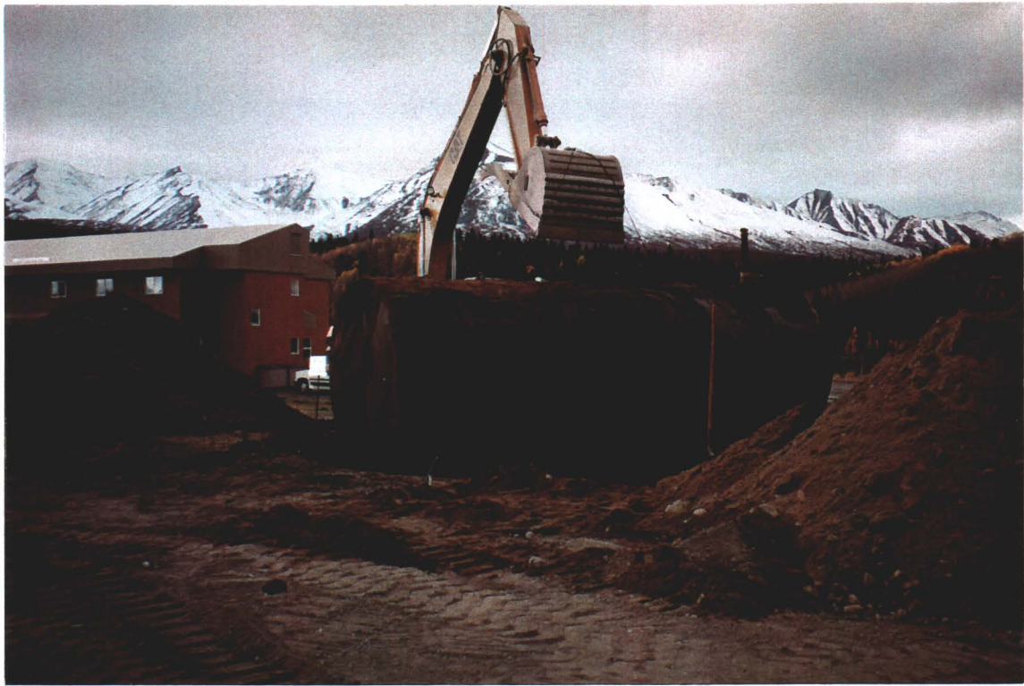
Photograph 6.9: Excavation of Underground Storage Tank northwest of the Maintenance Building
