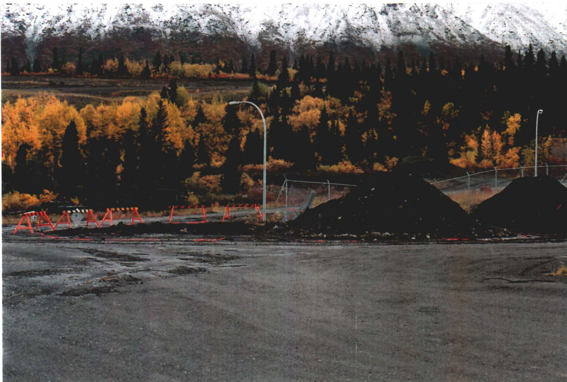
Photograph 6.2: Uncontaminated overburden removed from burn pit stockpiled to the side of the excavation for future backfilling use
