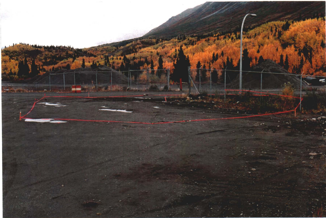
Photograph 6.1: Demarcated of the Burn Pit prior to excavation
