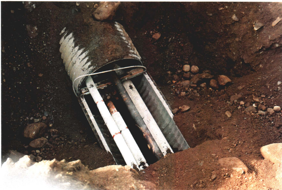
Photograph 3.12: A metal utilidor encountered at a depth of 2 m in TP99-45 with a section of the cover removed.
