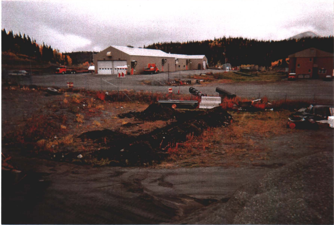
Photograph 6.7: Trench excavated on the north side of the site to enable the removal of 200 mm diameter culvert
