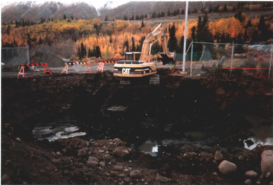
Photograph 6.3: Excavation of the burn pit and surrounding area. Note the heavily stained soils in the immediate vicinity of the former burn pit location (center of the photograph).
