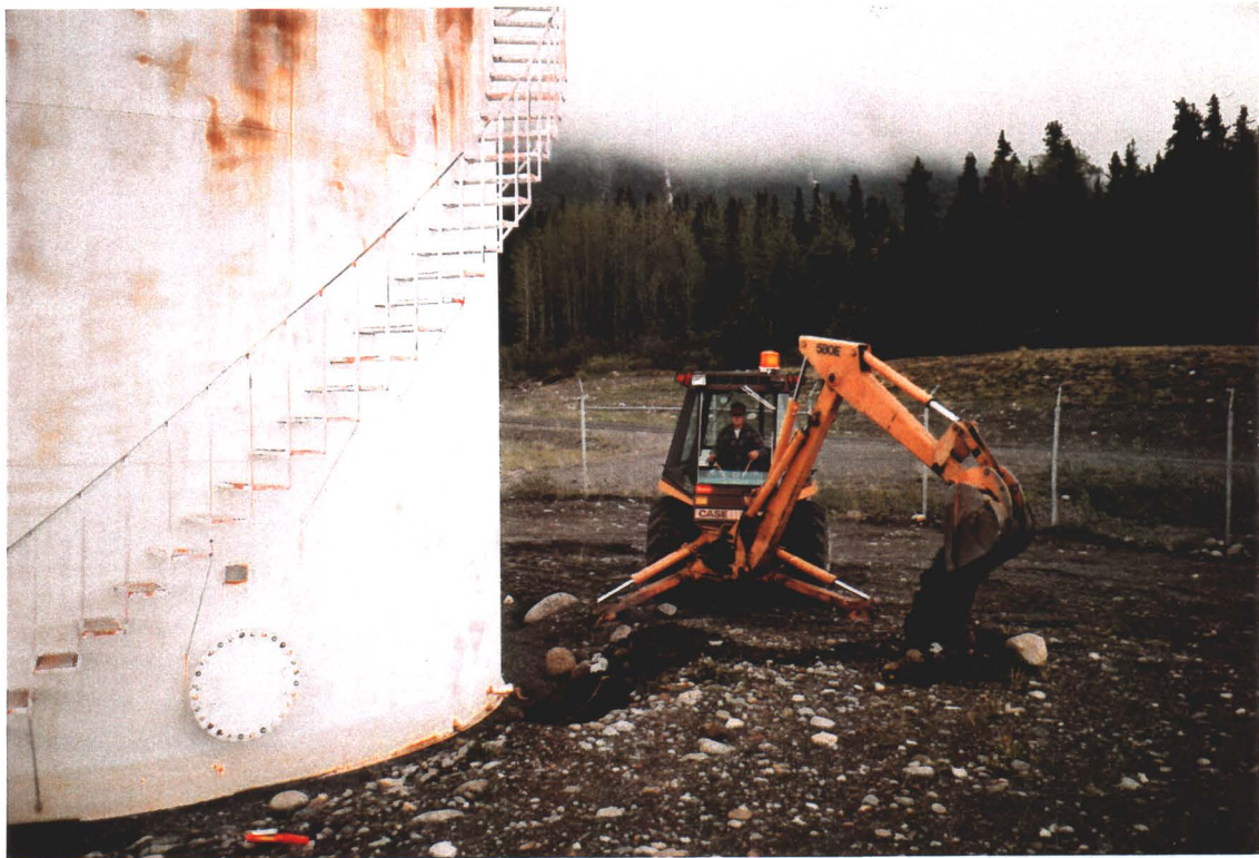
Photograph 3.3: Excavating a test pit near the empty large above ground storage tank (AST) located south of the maintenance building
