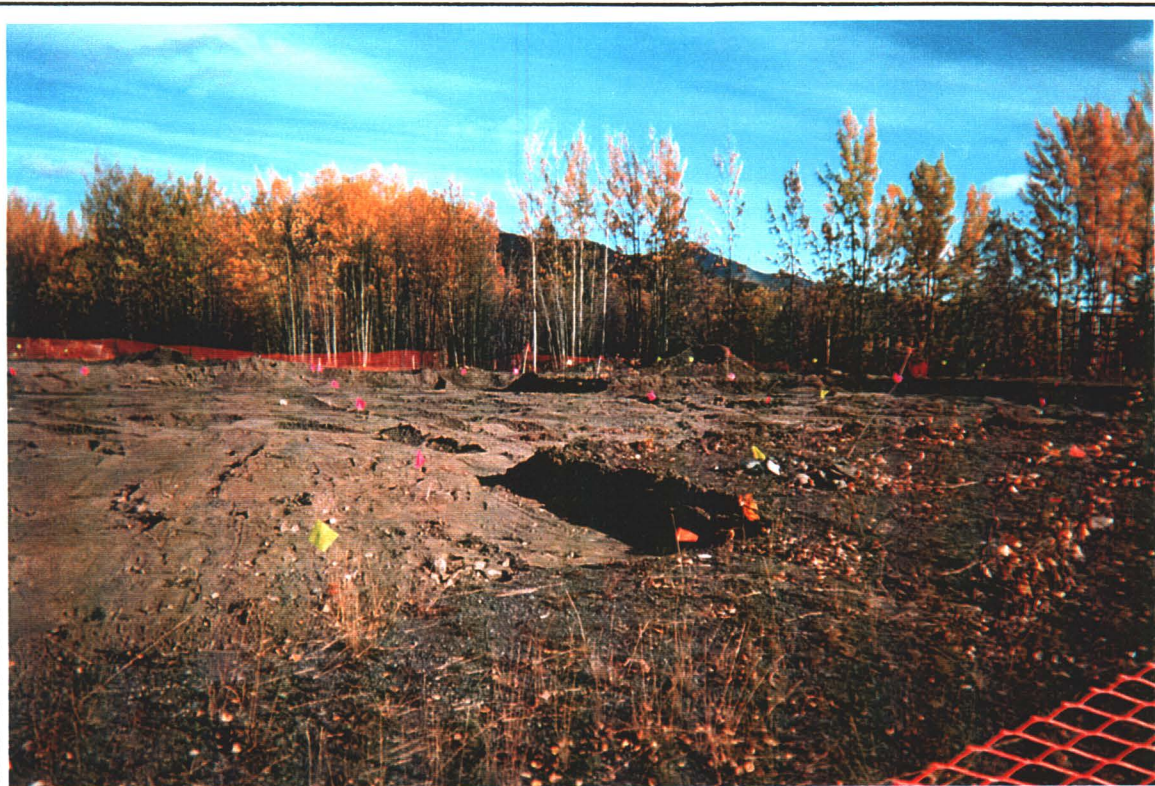
PHOTO 3: Main excavation. Pink and yellow survey flags mark sampling locations.
