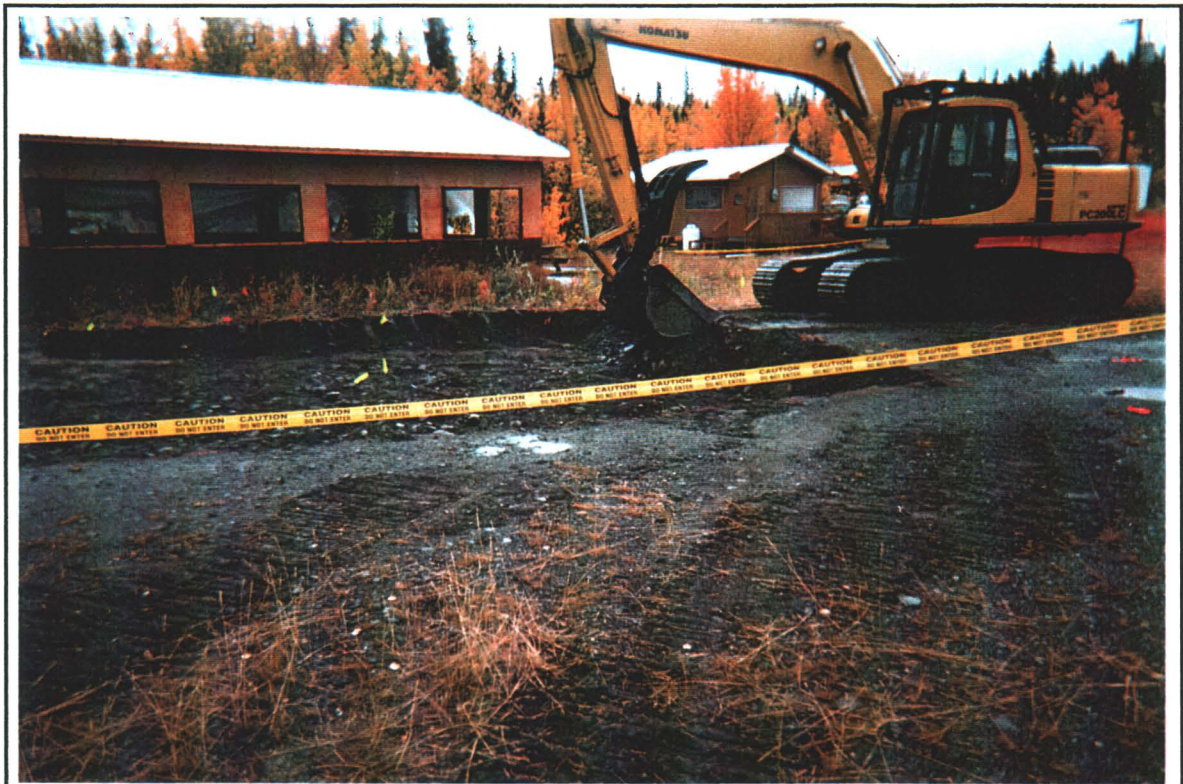
PHOTO 1: Remediation of small area south of the assembly hall.
