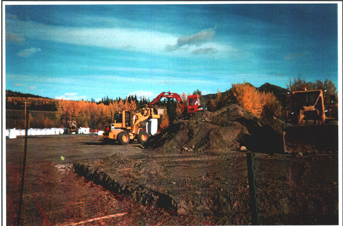
PHOTO 2: Soil bagging operation. Trench in foreground delineates area to be excavated.
