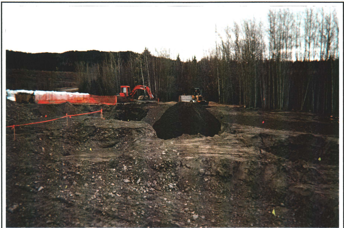
PHOTO 8: Backfill being pushed into southeast corner of excavation. Excavation advanced to 2.5m depth in some of the cells in this area.
