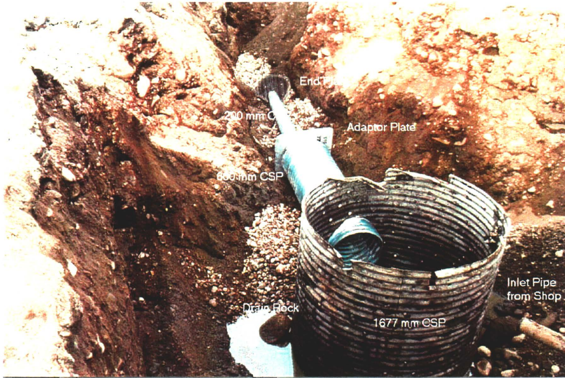
Photo 3: Looking north during infiltration gallery installation. Note influent pipe from shop in front right.
