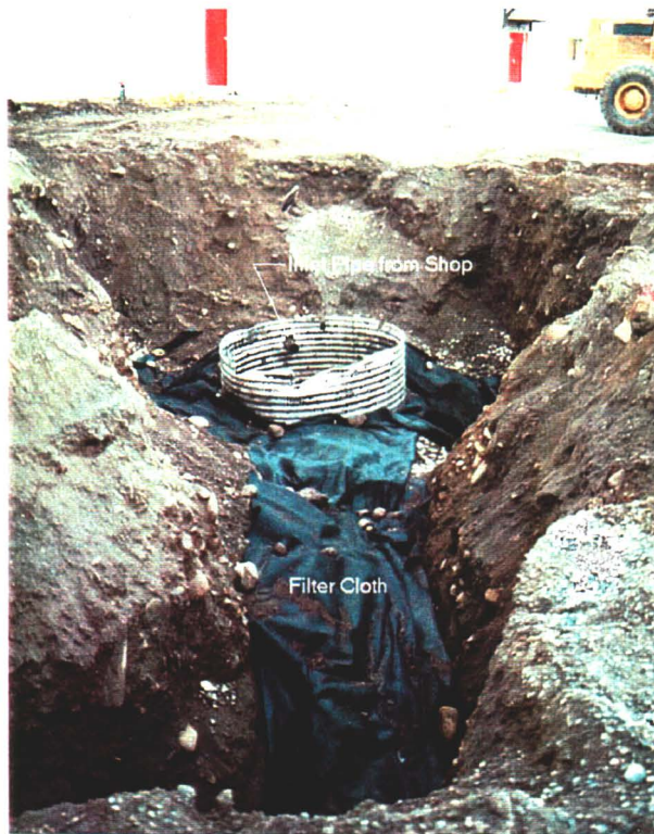
Photo 3: Looking north during infiltration gallery installation. Note influent pipe from shop in front right.
