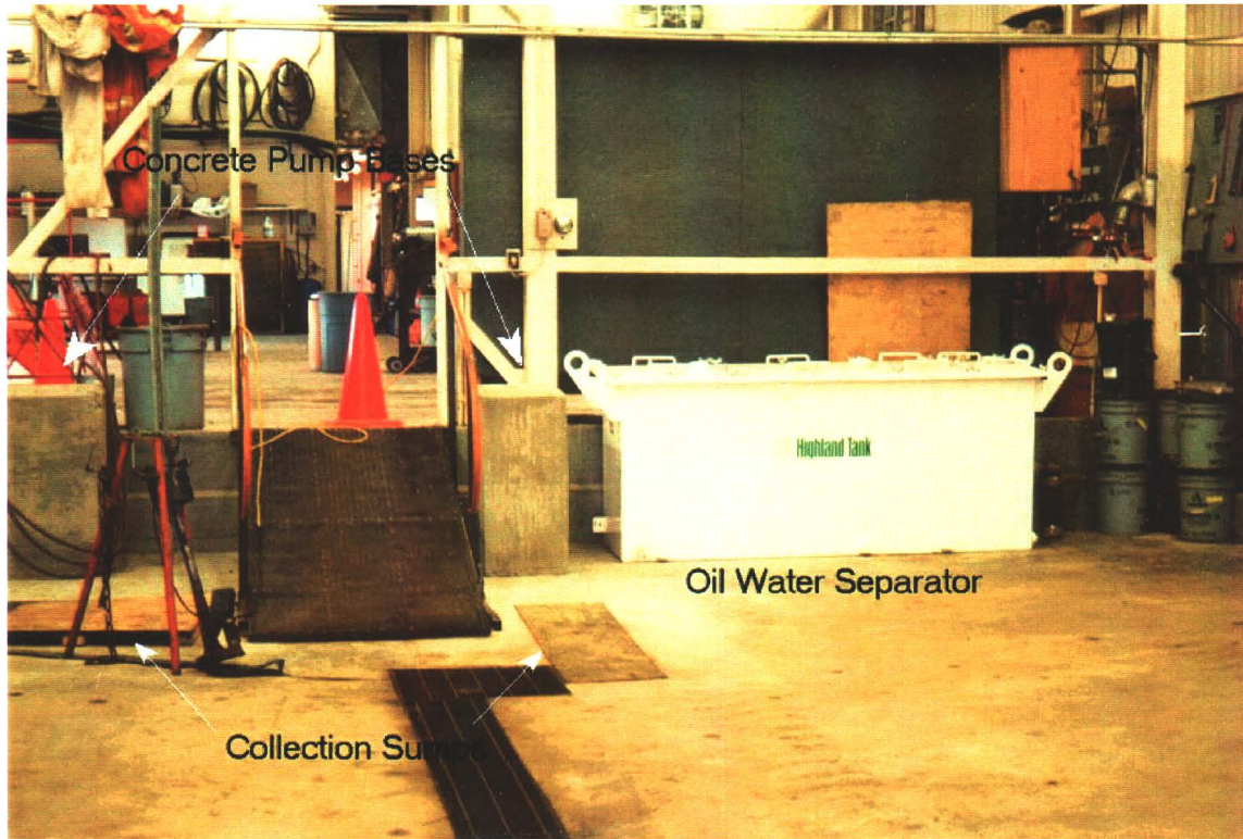
Photo 1: Concrete work, floor drains and oil water separator (not commissioned).
