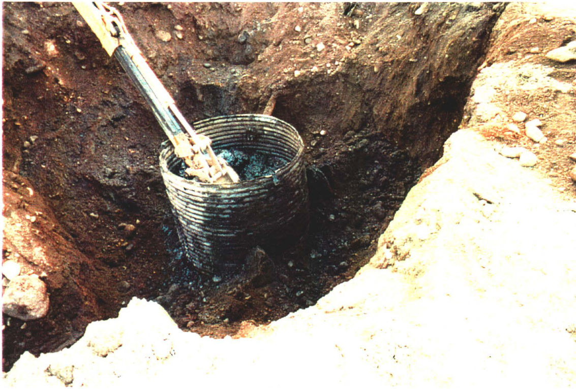
Photo 2: Excavation of hydrocarbon impacted material from the seepage pit location.
