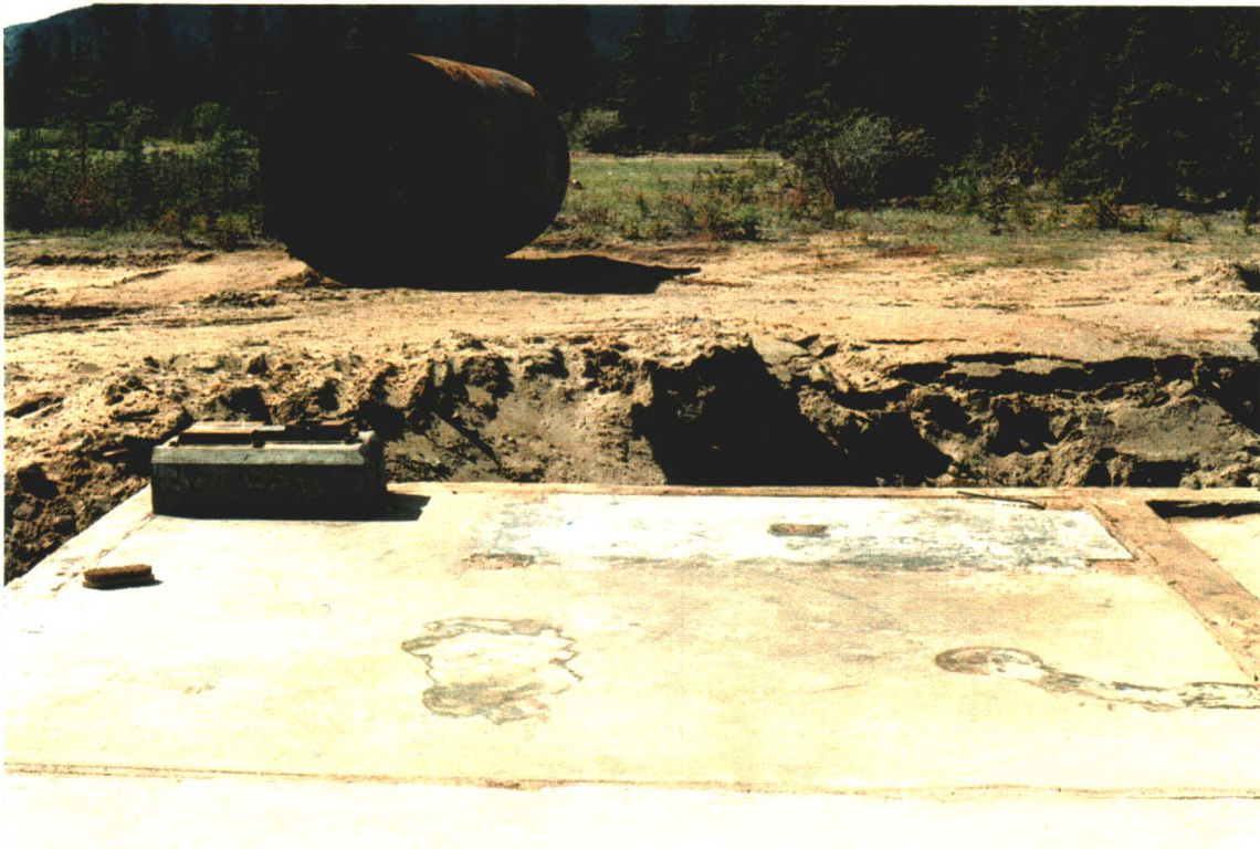
Photograph IV-6: Pit and tank after removal of the powerhouse diesel tank.
