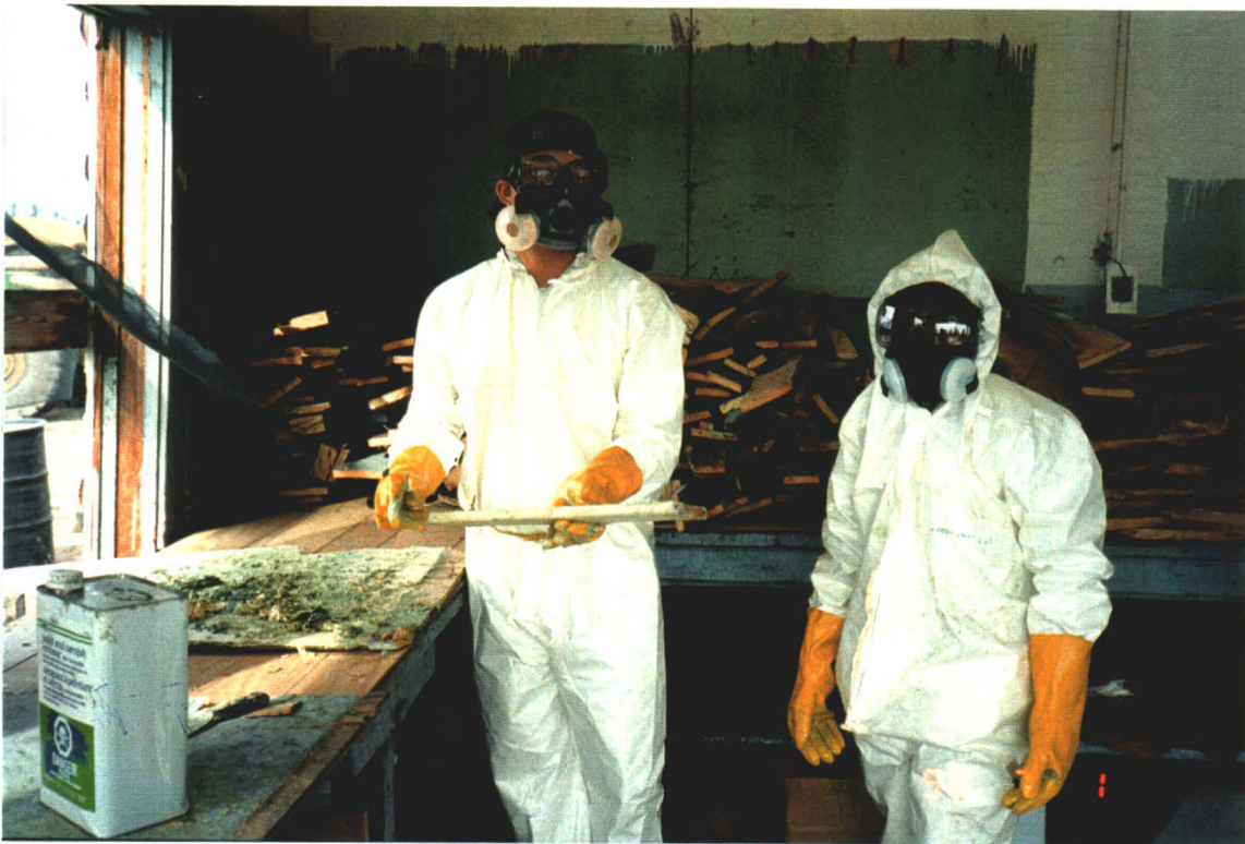
Photograph IV-4: Powerhouse wooden plank during chemical paint stripping.
