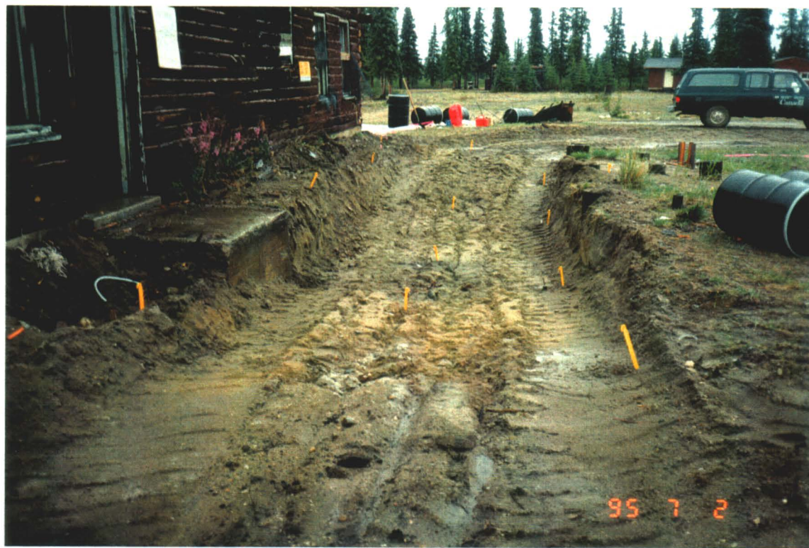
Photograph III-5: Excavated area at AA108 and AA115, the powerhouse south stain after removal of DCC-I contaminated soil.
