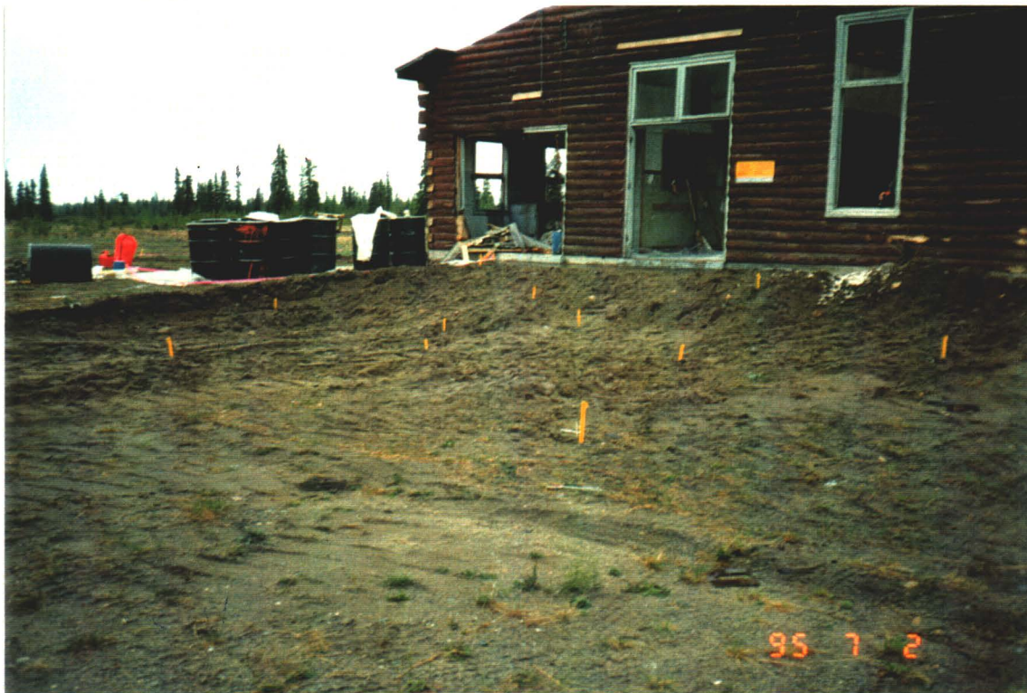
Photograph III-3: Excavated area at AA101, the powerhouse east stain, after removal of DCC-I contaminated soil.
