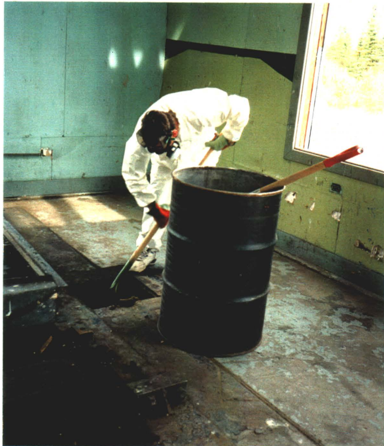
Photograph IV-2: Powerhouse generator sump soil excavation and containment in barrels.
