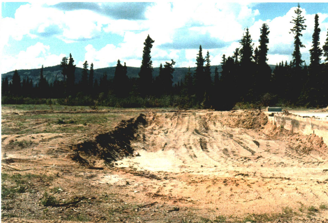
Photograph IV-8: Graded trench after removal of soil from around the powerhouse concrete pad.
