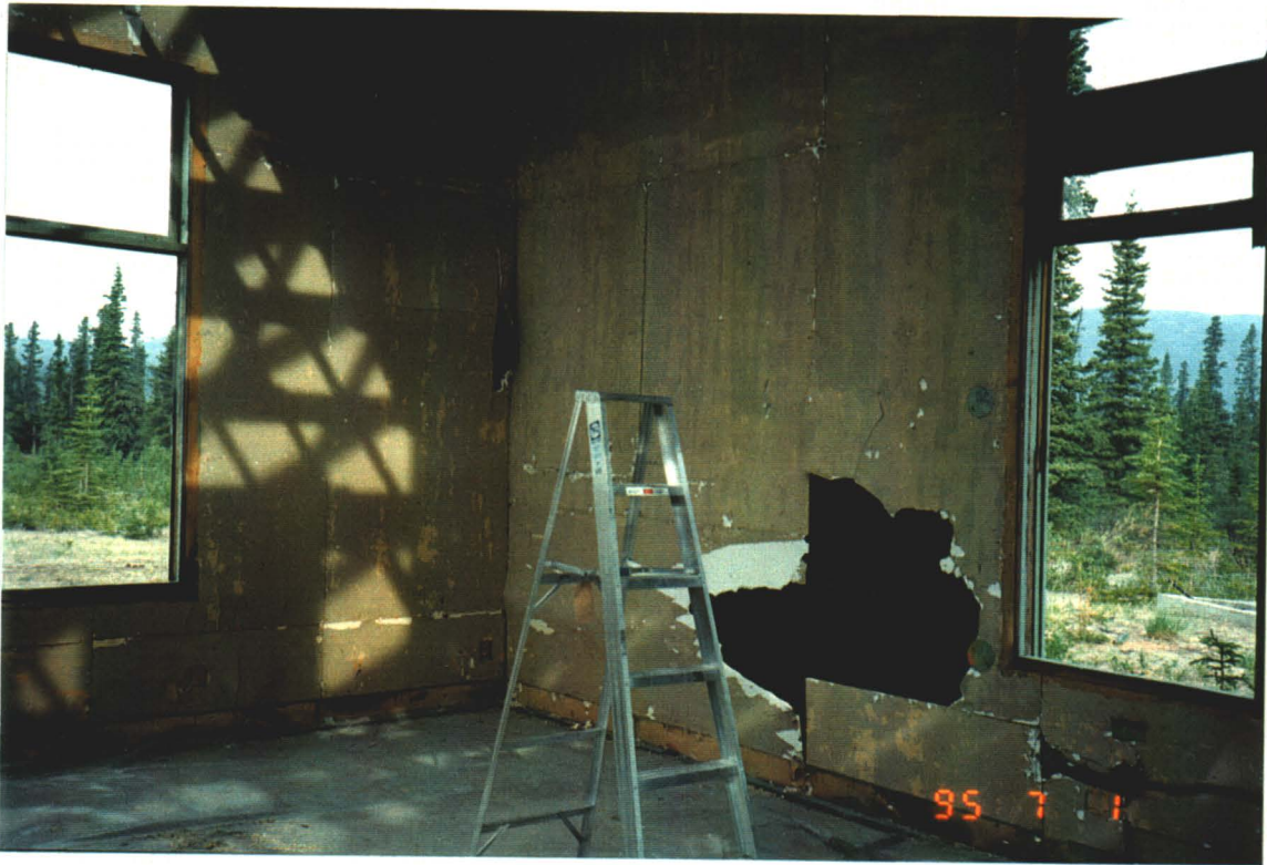
Photograph IV-3: Powerhouse walls after physical paint stripping.
