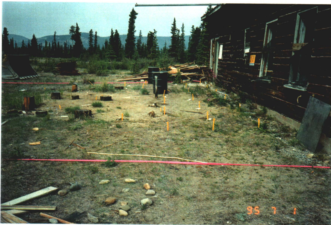
Photograph III-4: Delineation and demarcation of contaminated area at AA108 and AA115 the powerhouse south stain.
