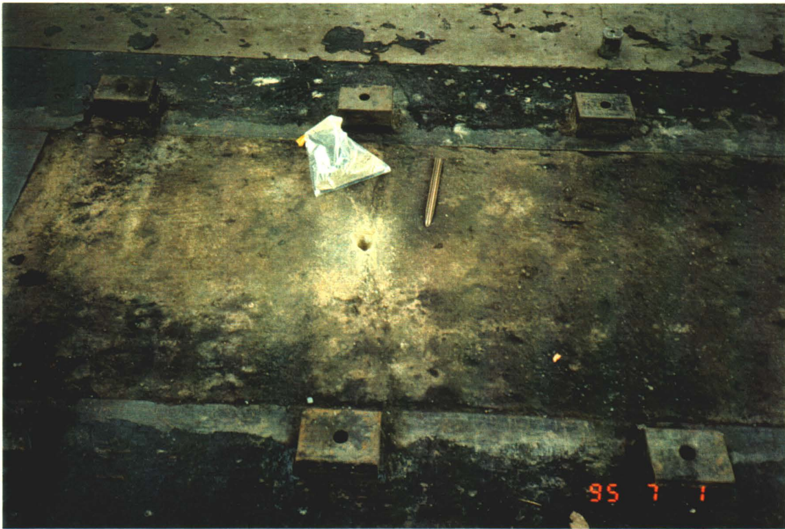
Photograph IV-5: Concrete sample removed from the powerhouse generator foundations.
