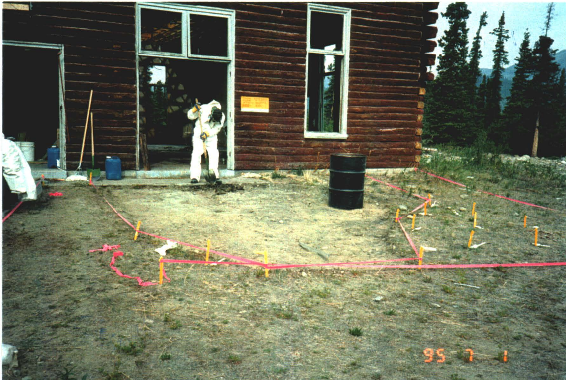
Photograph III-2: Excavation and barrel containment of DCC-II/CCME R/P PCB-contaminated soils at AA101, the powerhouse east stain.
