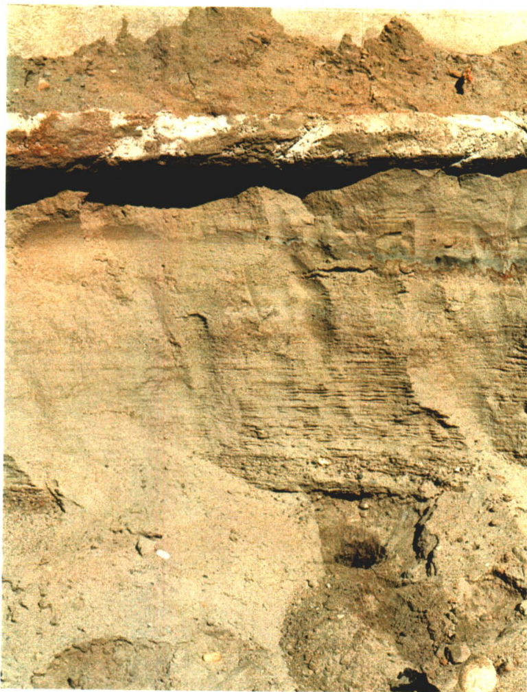
Photograph IV-8: Graded trench after removal of soil from around the powerhouse concrete pad.
