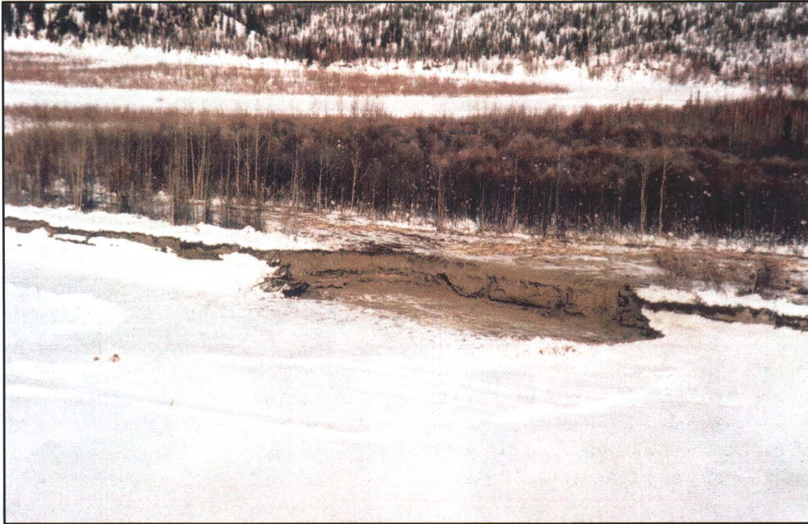
Photograph 4.1: Area view of the Peel-Caribou Staging Area looking north, after project completion in March 2002
