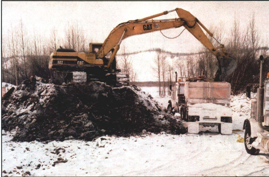
Photograph 2.11: Loading contaminated soils and debris into Seacan containers
