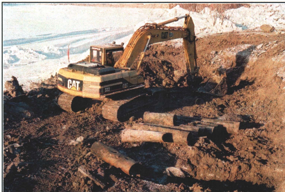
Photograph 2.10: Drill casings excavated from the waste pit and the excavator
