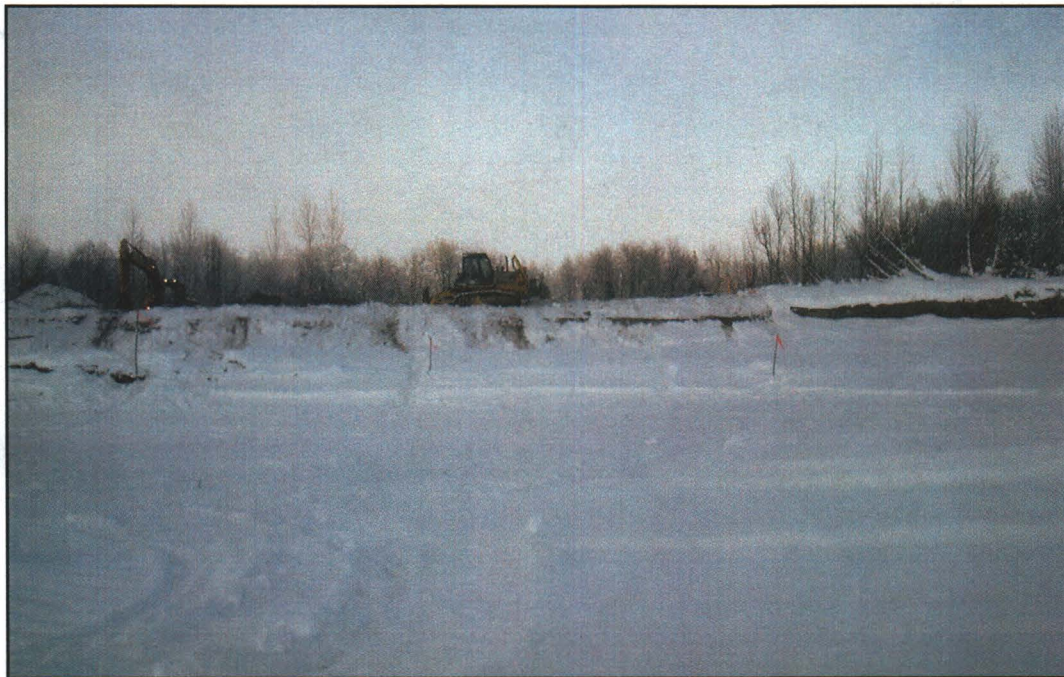
Photograph 2.4: Removing snow cover from the waste site as viewed from the frozen river
