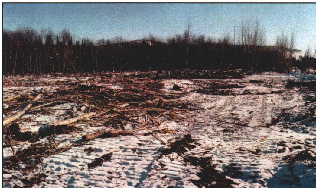
Photograph 2.19: Stockpile area after project completion
