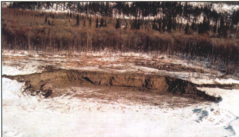
Photograph 2.18: Waste Pit after removal of all debris and contaminated soil
