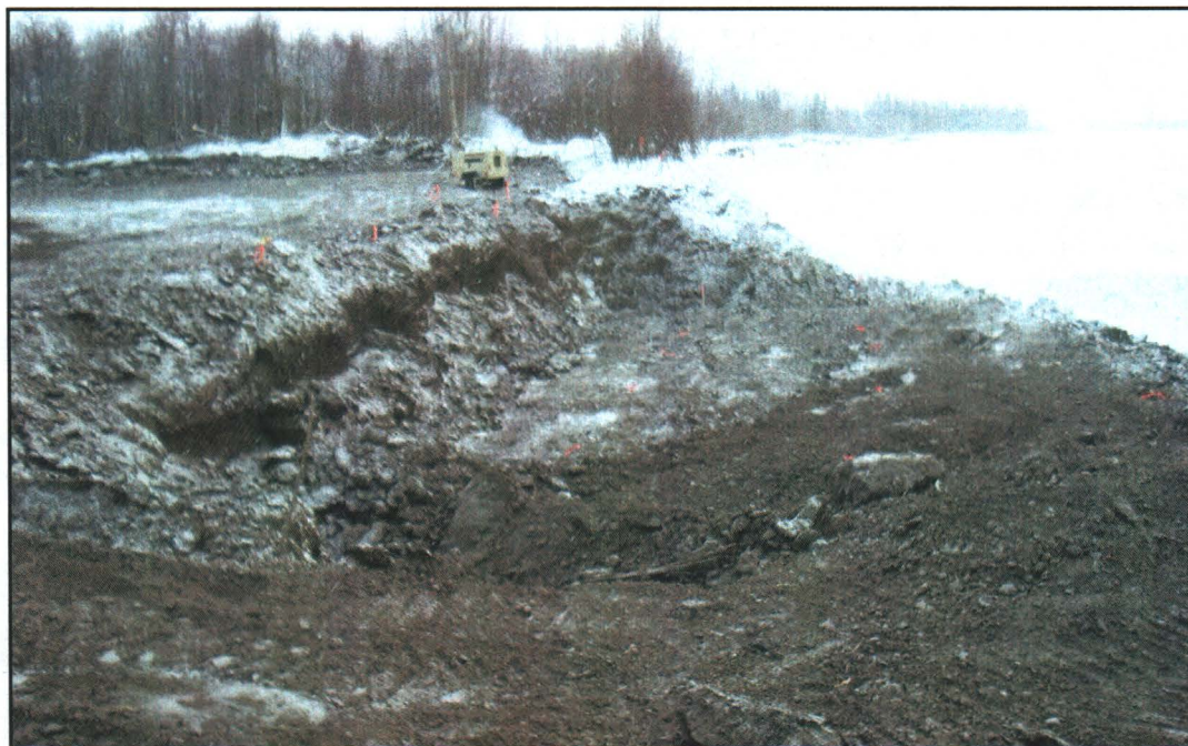
Photograph 2.7: Waste pit after removal of overburden from the contaminated zone
