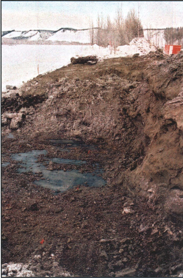
Photograph 2.8: Waste pit after excavation of contaminated soils
