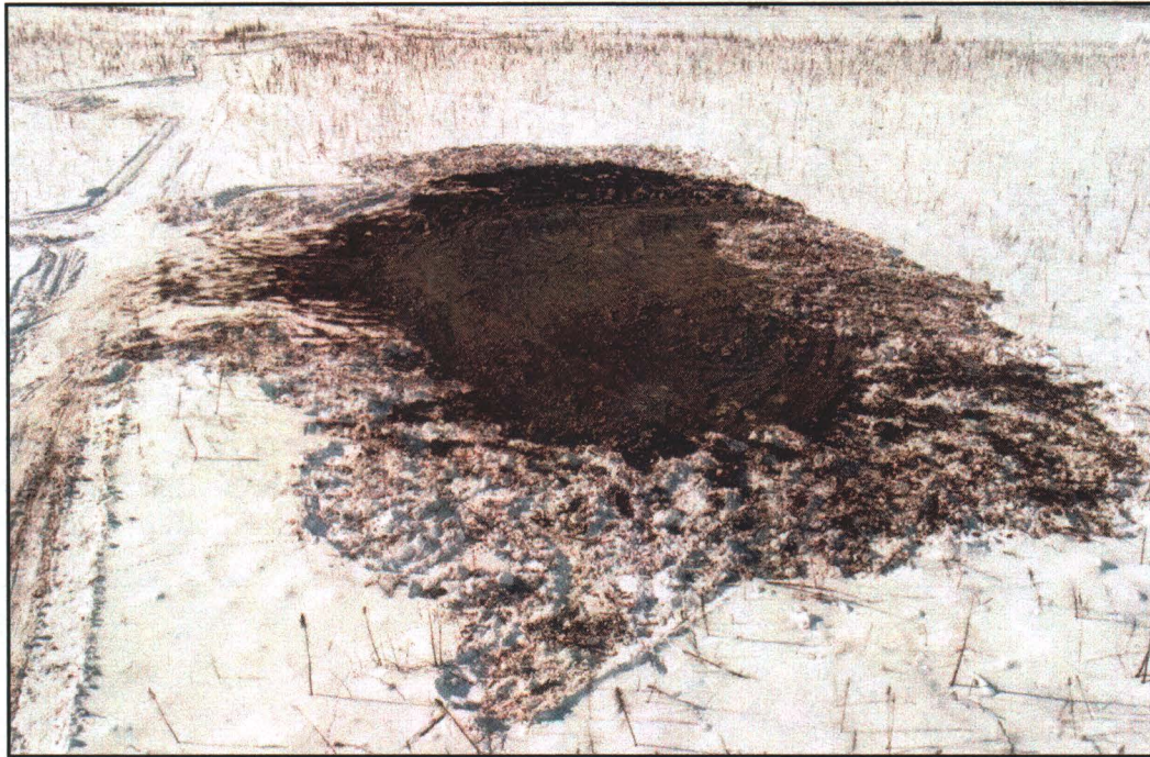
Photograph 2.16: Aerial view of the new landfill after burial of non-contaminated debris and site re-contouring.
