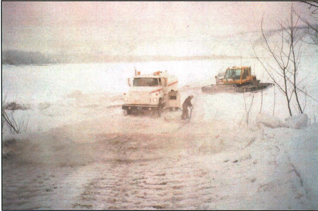
Photograph 2.1: Water truck and Challenger working on the access road near the waste site
