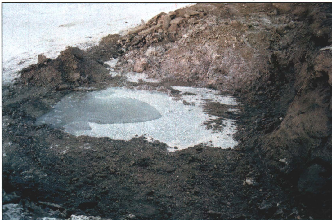
Photograph 2.17: Small pool generated after excavation at the contaminated zone
