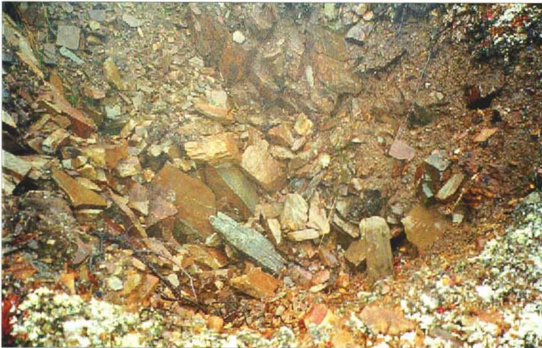
Photo 49-1 : Vanguard. Shaft #2 has collapsed 1m below surface, the timber post in the bottom right hand corner is all that marks the location. (Azimuth 110°)
