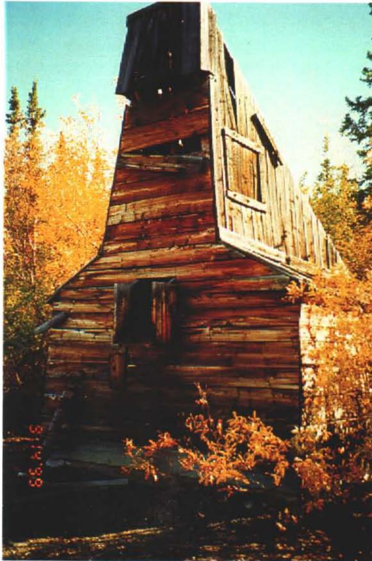
Photo 61-4: Wood framed headframe (61A).
