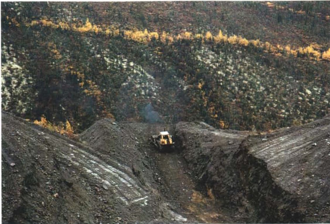
Photo 55-1: Bulldozer working at Runer site.
