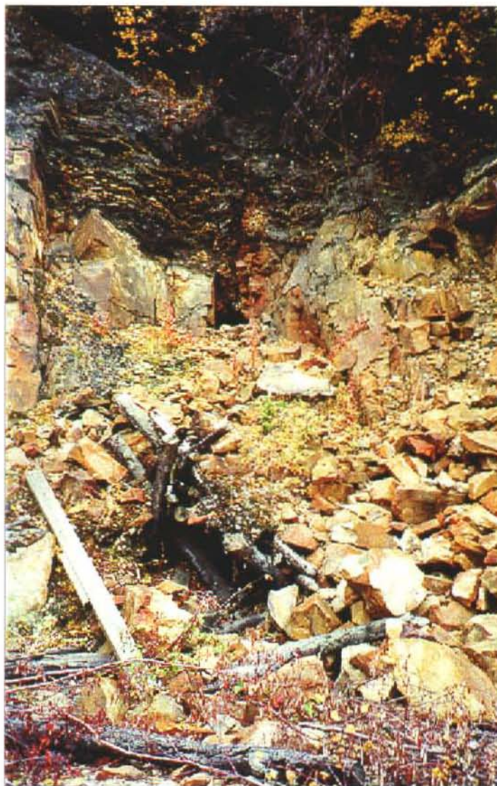
Photo 66-1 : Moon. The first 10m of the portal structure into the Moon adit has collapsed. (Azimuth 216°)
