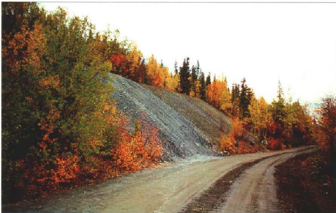
Photo 54-5: View of east side of Hogan waste rock dump. Highly acidic material appears in a zone that is light grey in color.
