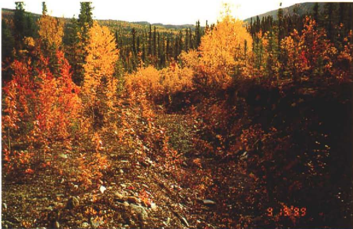
Photo 62-1: Partially overgrown trench adjacent to road.
