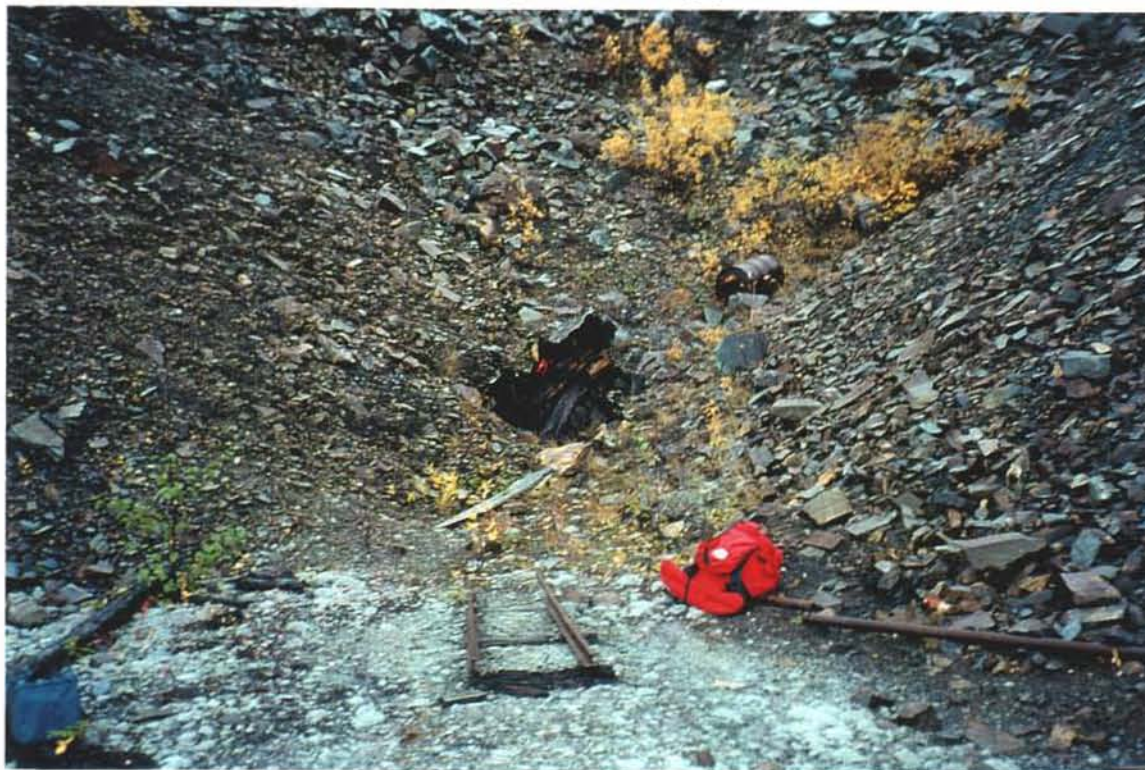
Photo 49-4 : Vanguard. The pile of broken logs and sheet metal marks the entrance to the Vanguard Adit. The first 30m of the adit have collapsed. (Azimuth 290°)
