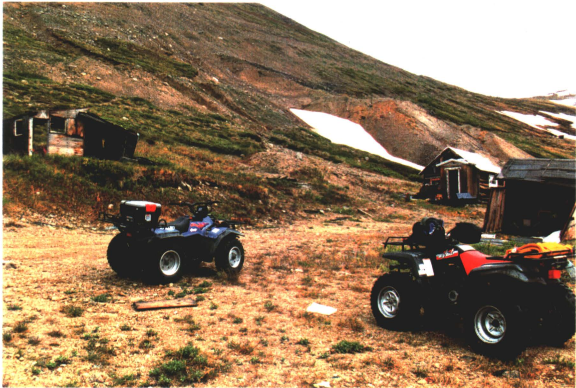
MINE EXPLORATION BUILDINGS (ADIT IN BACKGROUND BEHIND SNOW)
