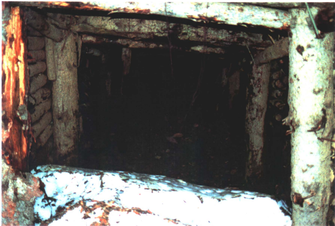
INTERIOR OF LOWER ADIT
