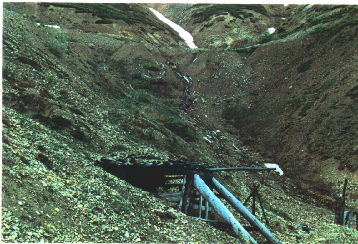
LOWER ADIT LOOKING UPSLOPE (NOTE WASTE IN GULLY FROM UPPER ADIT)
