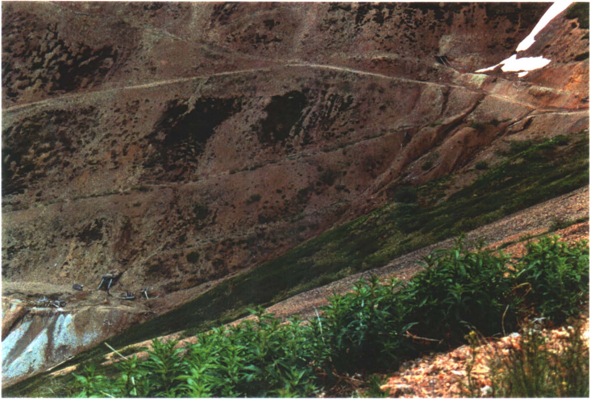
UPPER AND LOWER ADITS AND WASTE DUMPS (NOTE EROSION)
