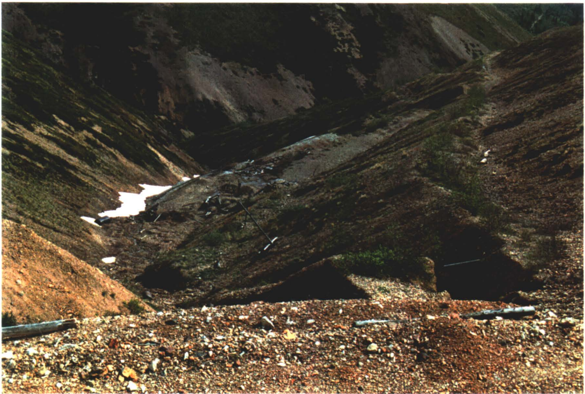
LOWER WASTE ROCK DUMP AND EROSION IN GULLY
