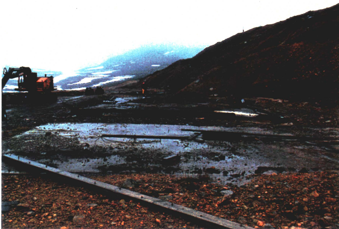
3. MILL FOUNDATIONS AND EXCAVATOR
