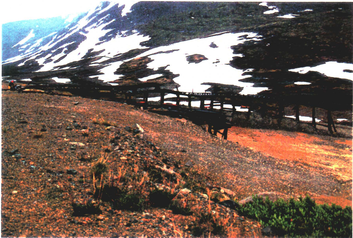
7. TRESTLE INTO WASTE DUMP
