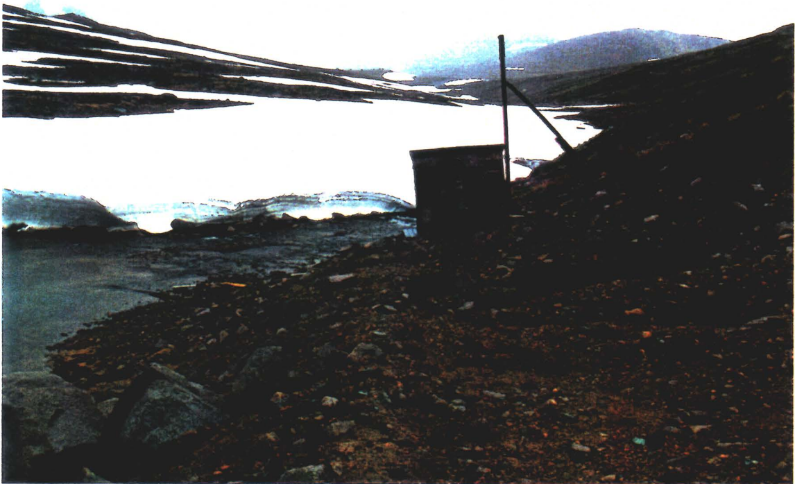
10. PUMPHOUSE ON BANK OF BIG THING CREEK
