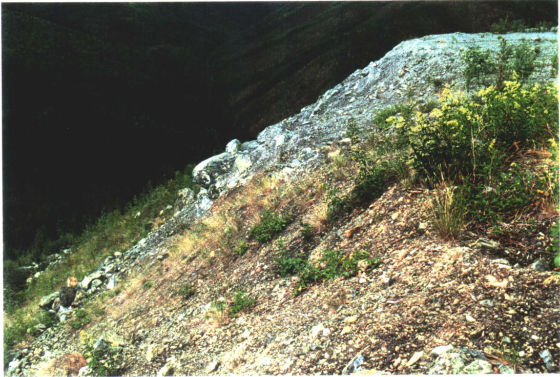
WASTE ROCK DUMP
