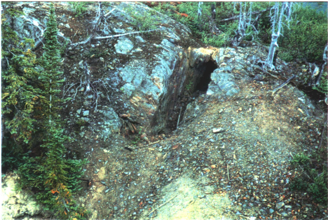
CLOSE-UP VIEW OF ADIT
