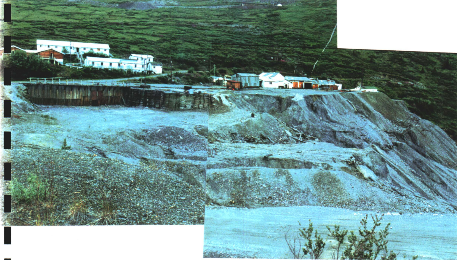
LEVEL 700 SITE WITH WASTE DUMP IN FOREGROUND
