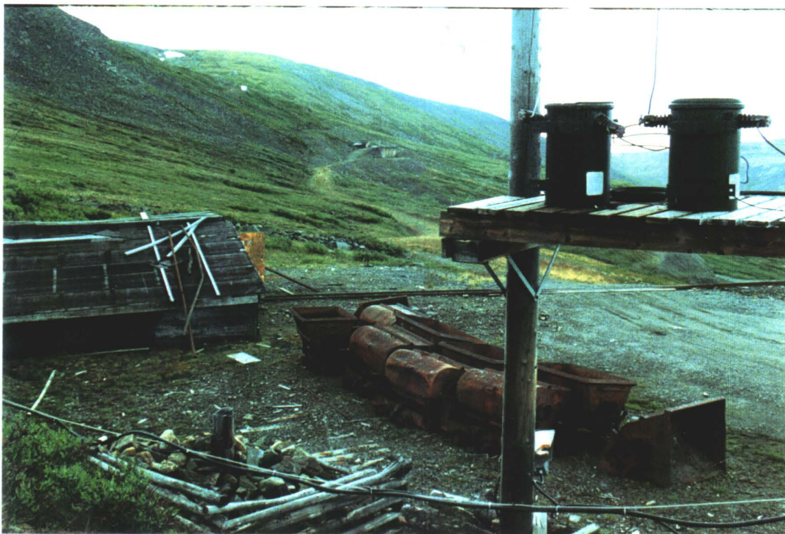
ORE CARS, TRANSFORMERS, AND ADIT BUILDING AT LEVEL 200
