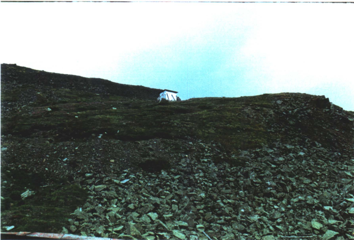
STRUCTURE ABOVE LEVEL 150 (POSSIBLY A VENTILATION SHAFT)
