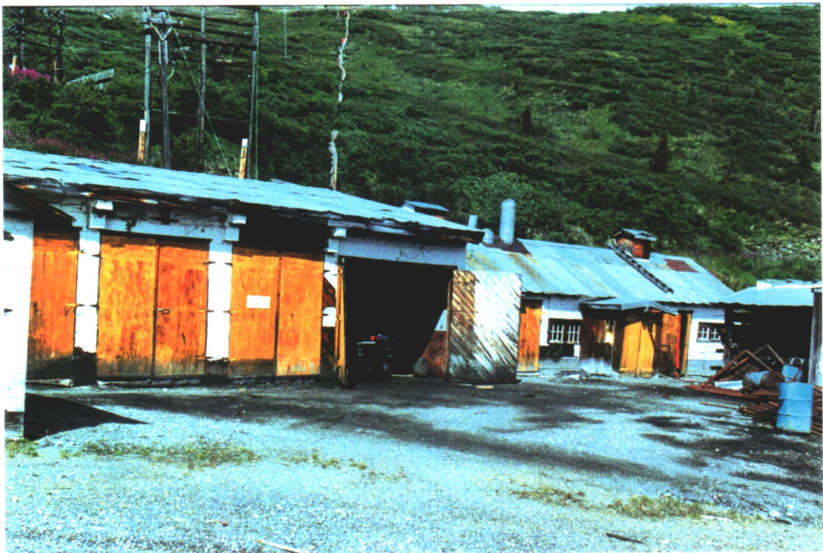
4 BAY GARAGE AND GENERATOR BUILDING (AT RIGHT)
