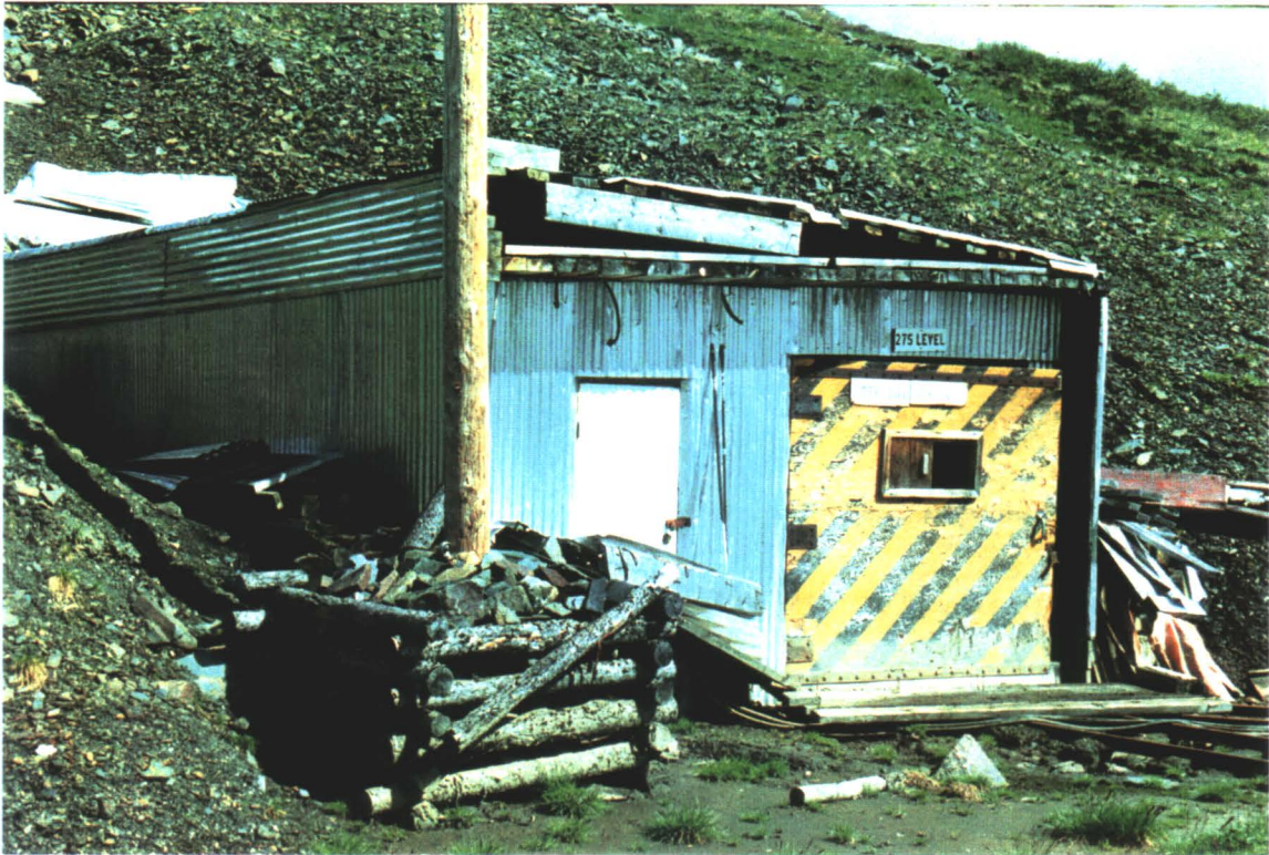
ADIT BUILDING AT ENTRANCE TO LEVEL 275
