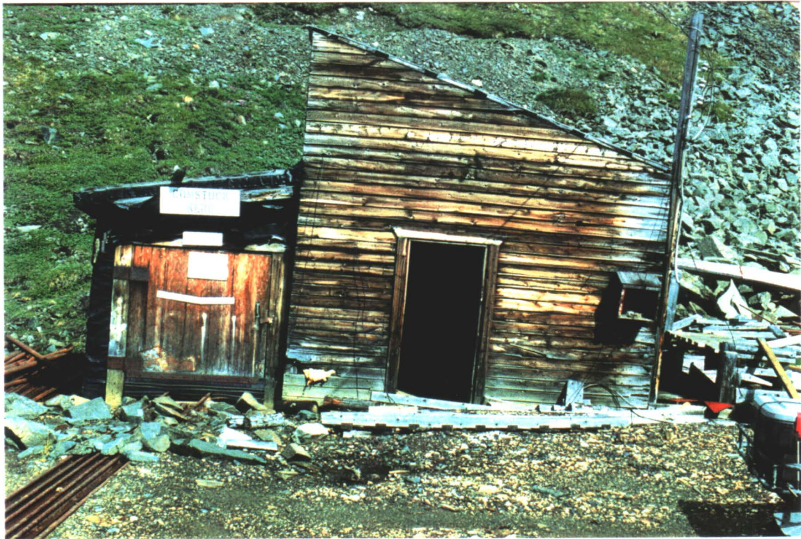
ADIT BUILDING AT LEVEL 150
