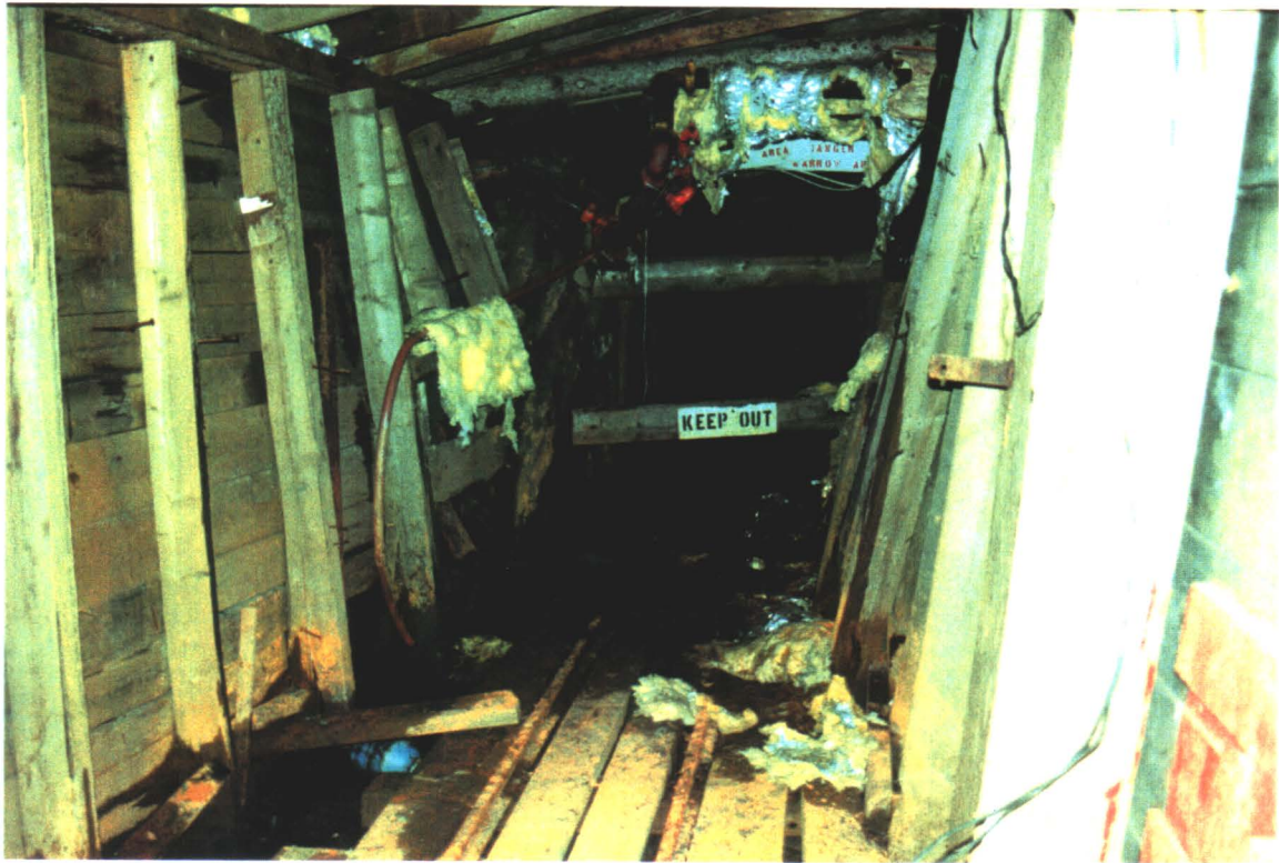
INTERIOR OF ADIT AT LEVEL 150
