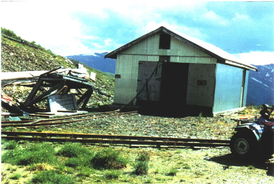
GARAGE WITH ELECTRICAL SWITCHING EQUIPMENT AT LEVEL 275
