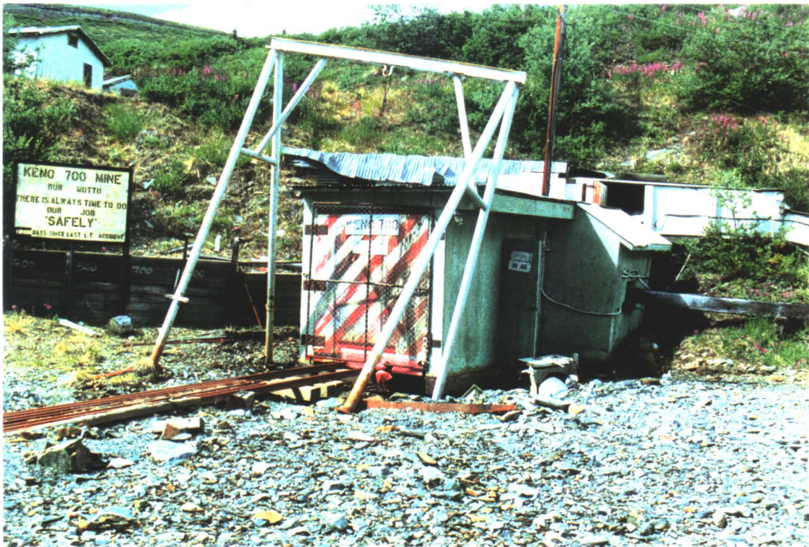
ENTRANCE TO ADIT AT LEVEL 700
