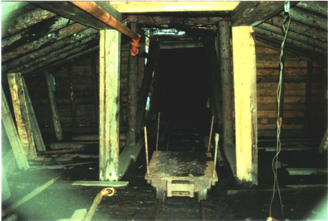
INTERIOR OF ADIT LEVEL 200
