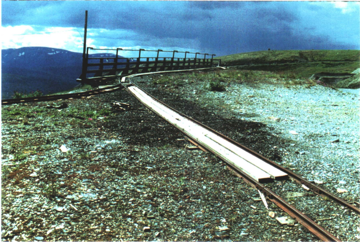
RAIL TO LOADOUT AT LEVEL 275
