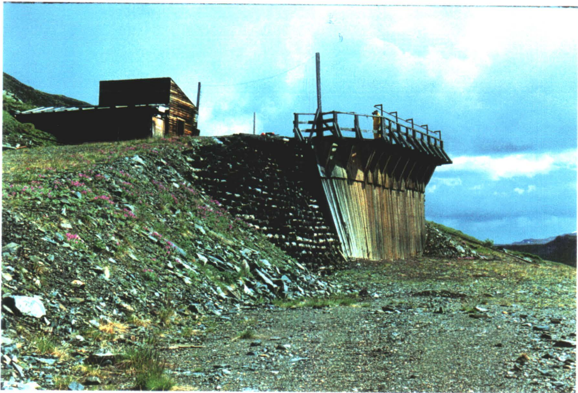
LOADOUT AND ADIT BUILDING AT LEVEL 150
