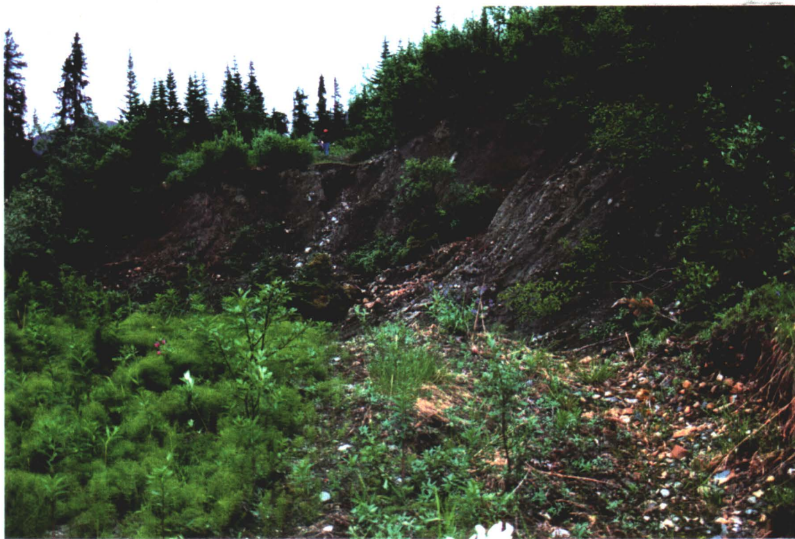
17. SLOPE FAILURE ACROSS ROAD
