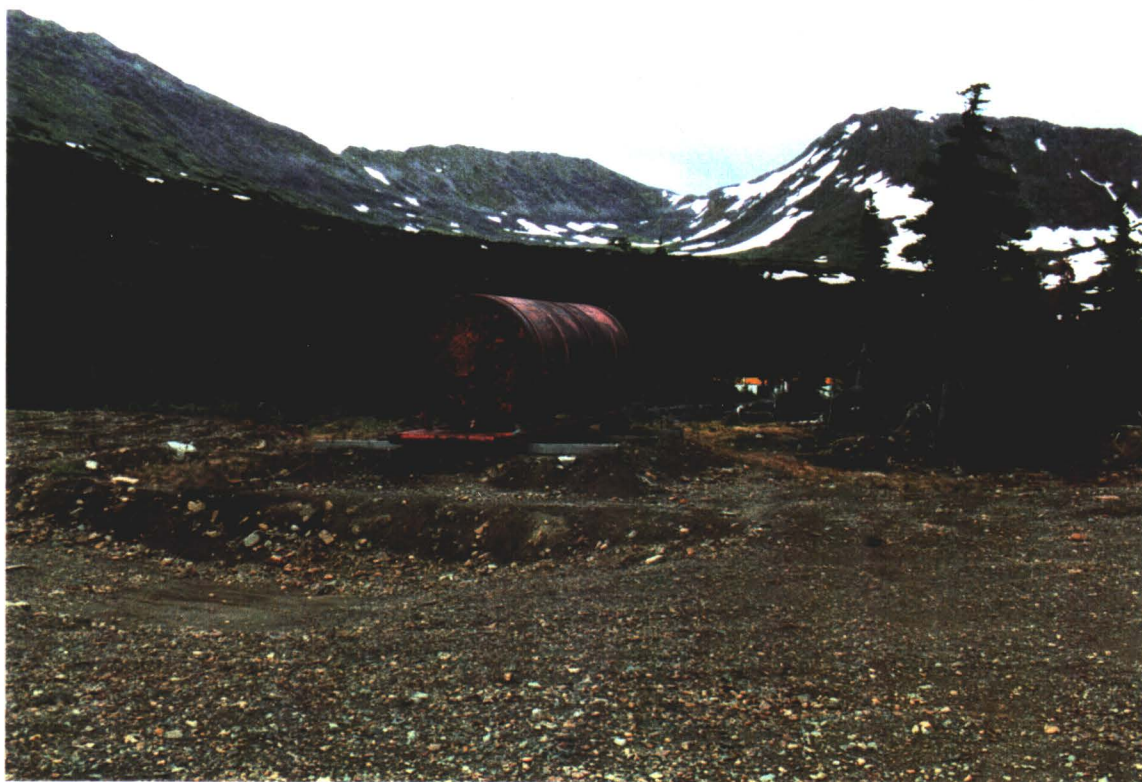
8. FUEL STORAGE TANK ON SKID FRAME
