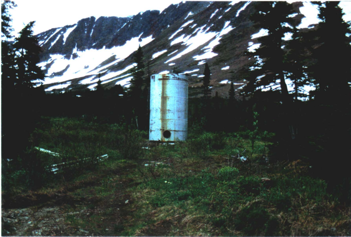
9. VERTICAL FUEL STORAGE TANK
