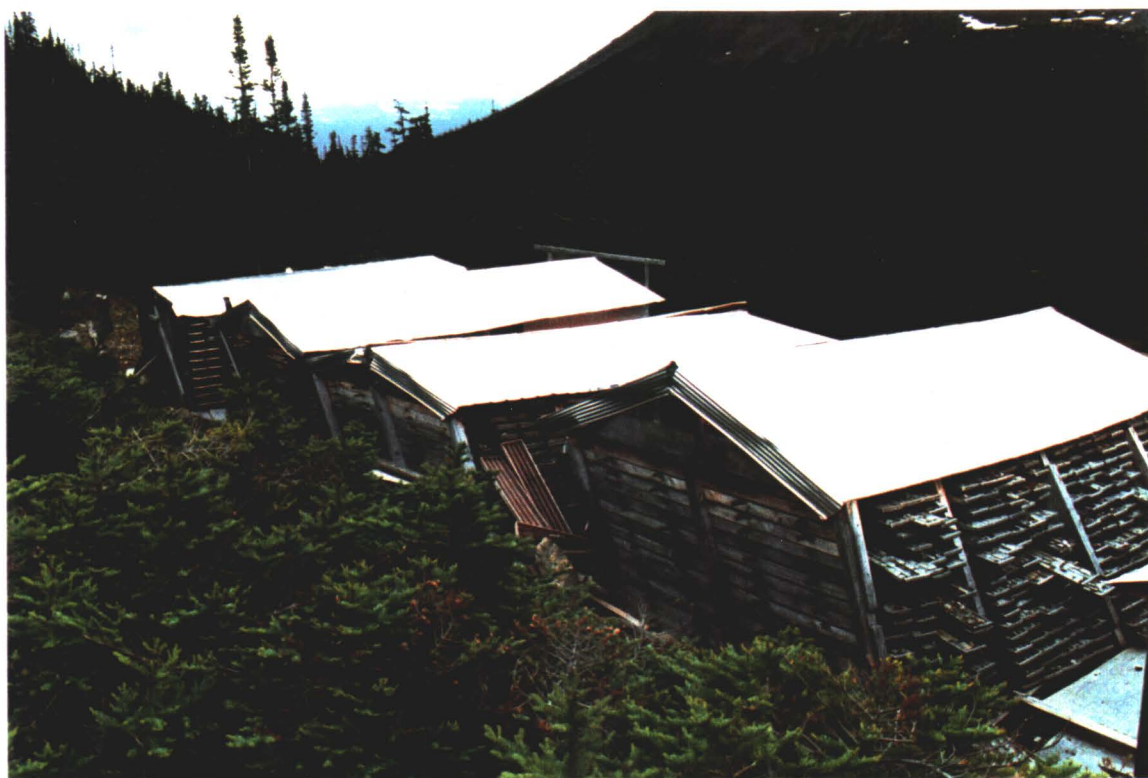
12. CORE STORAGE SHEDS
