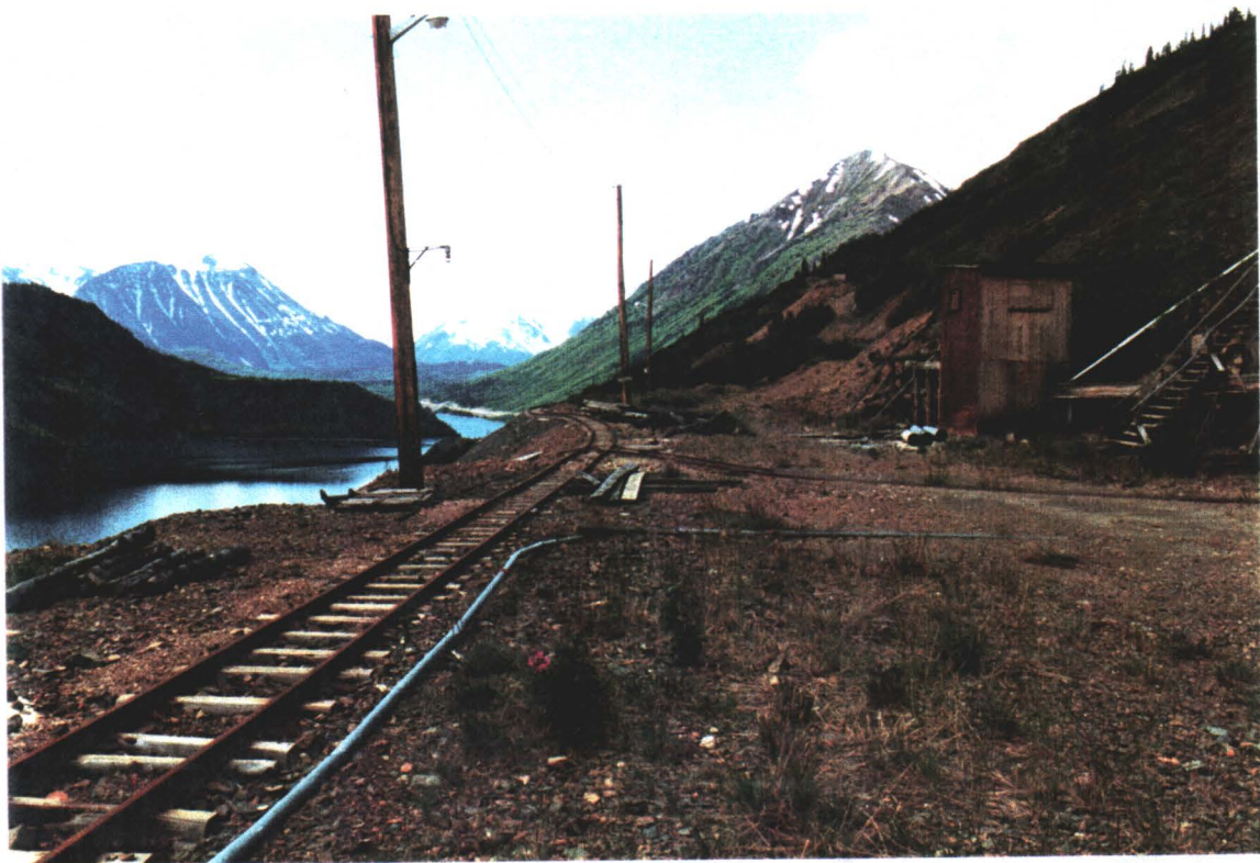
ADIT #2 FACING SOUTH
