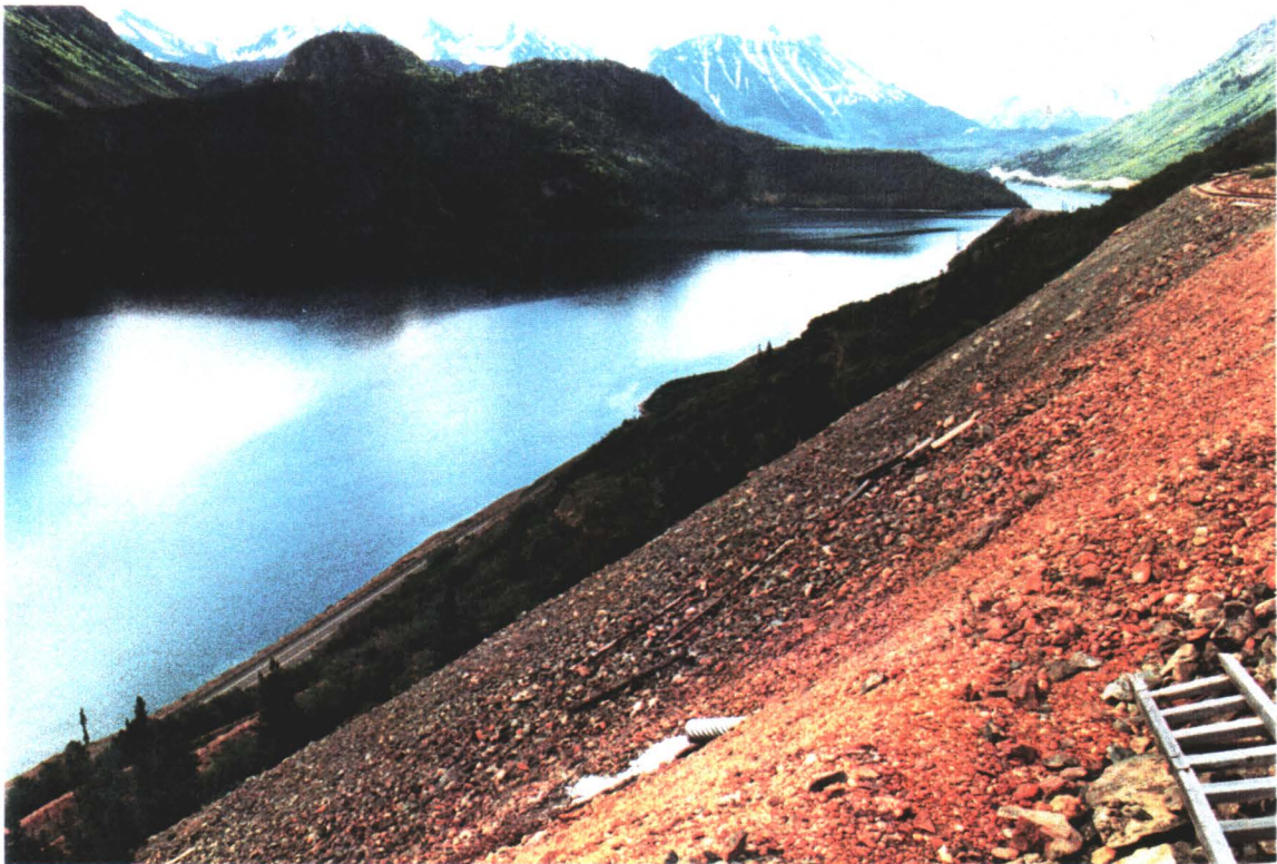
DRAINAGE OUTLET ON WASTE ROCK SLOPE
