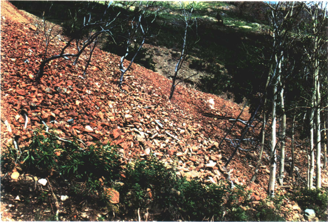
DEAD VEGETATION AT TOE OF WASTE ROCK
