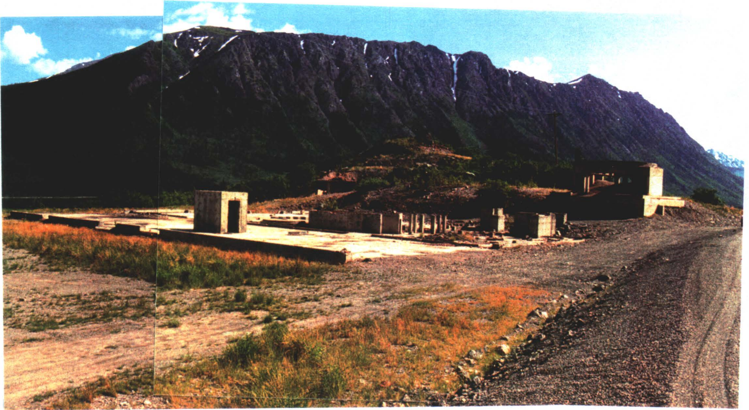
FOUNDATION OF MILL SITE
