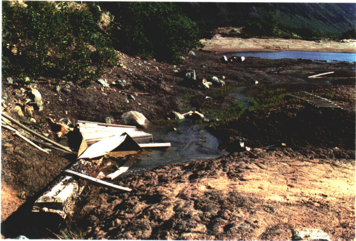
SEEPAGE UPSLOPE OF TAILINGS
