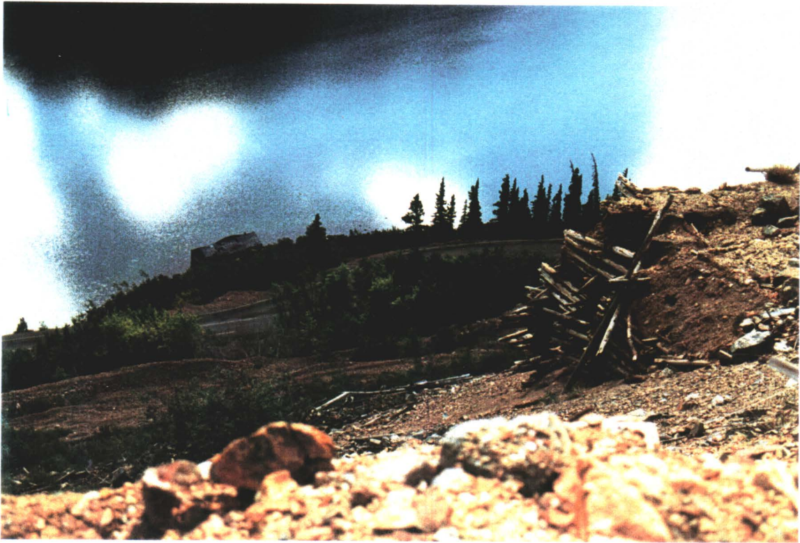
DOWNSLOPE OF LOADING STRUCTURE. NOTE DETERIORATING RETAINED WASTE ROCK
