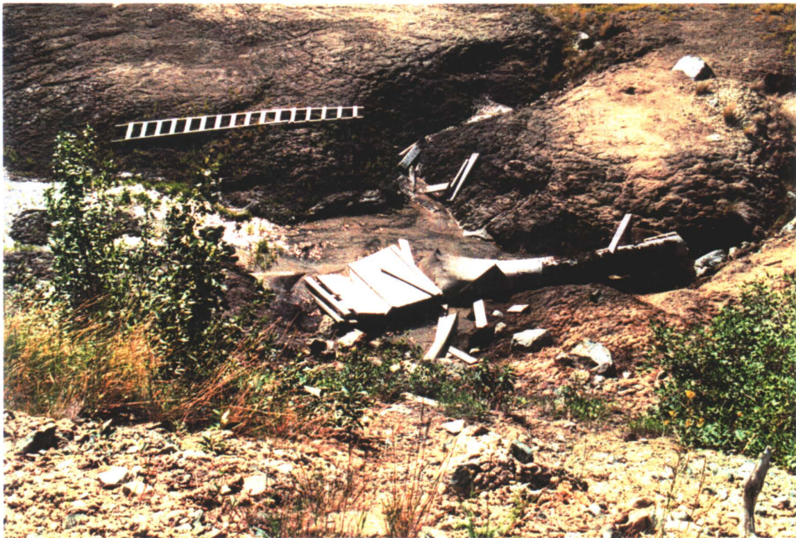
INLET TO DRAINAGE PIPE
