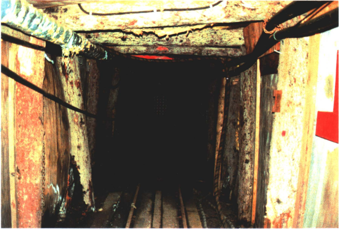
INTERIOR OF ADIT #2
