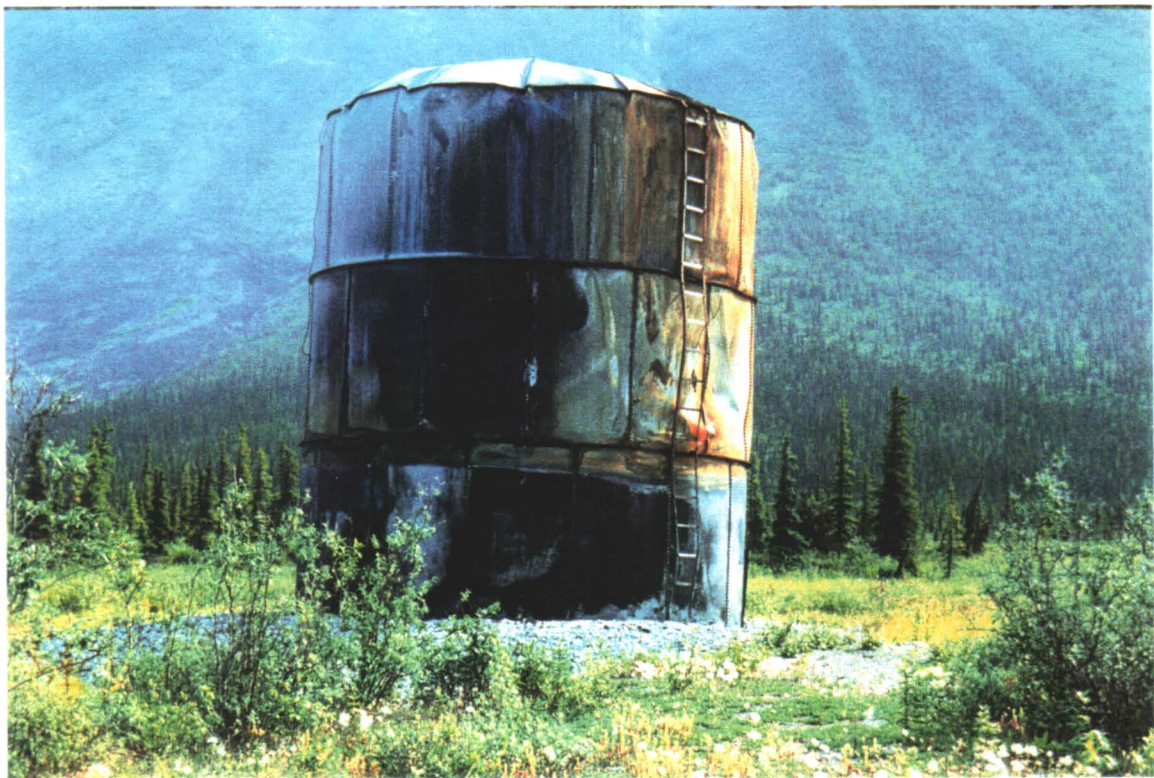
EMPTY FUEL STORAGE TANK
