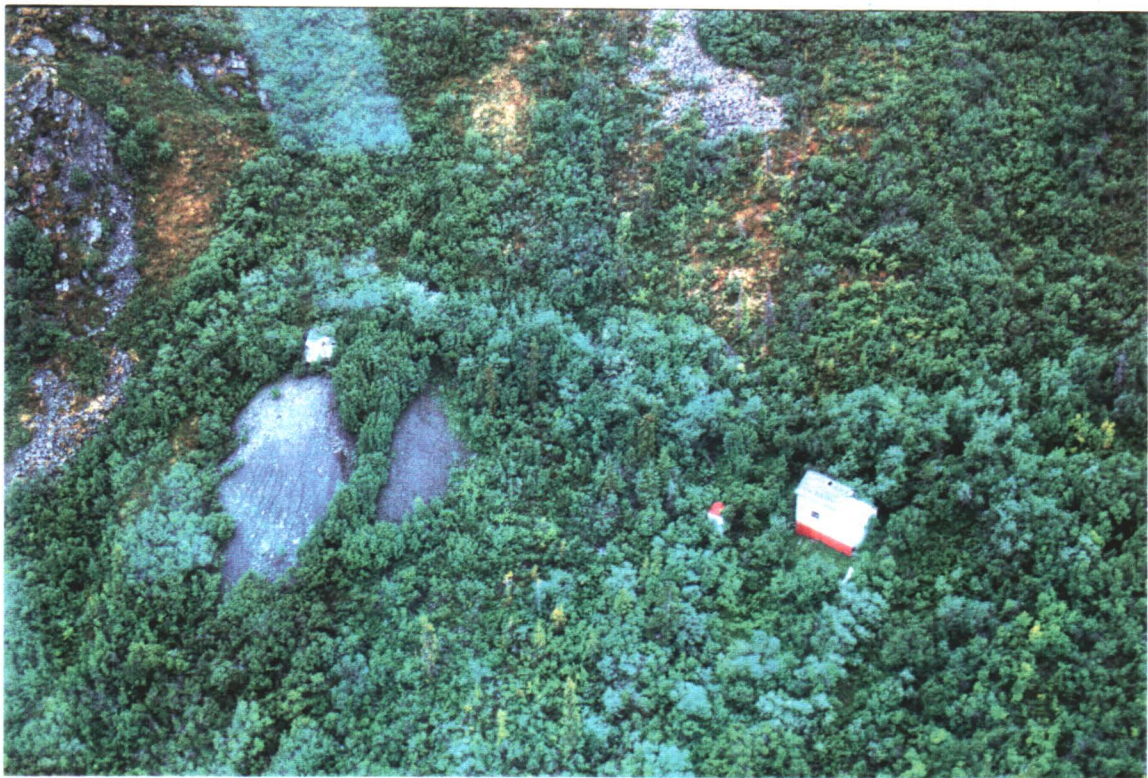
SITE WITH WASTE ROCK DUMP BELOW UPPER SITE
