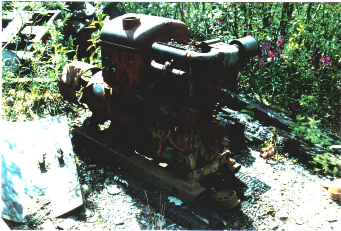
ELECTRICAL GENERATOR AND SURROUNDING DEBRIS
