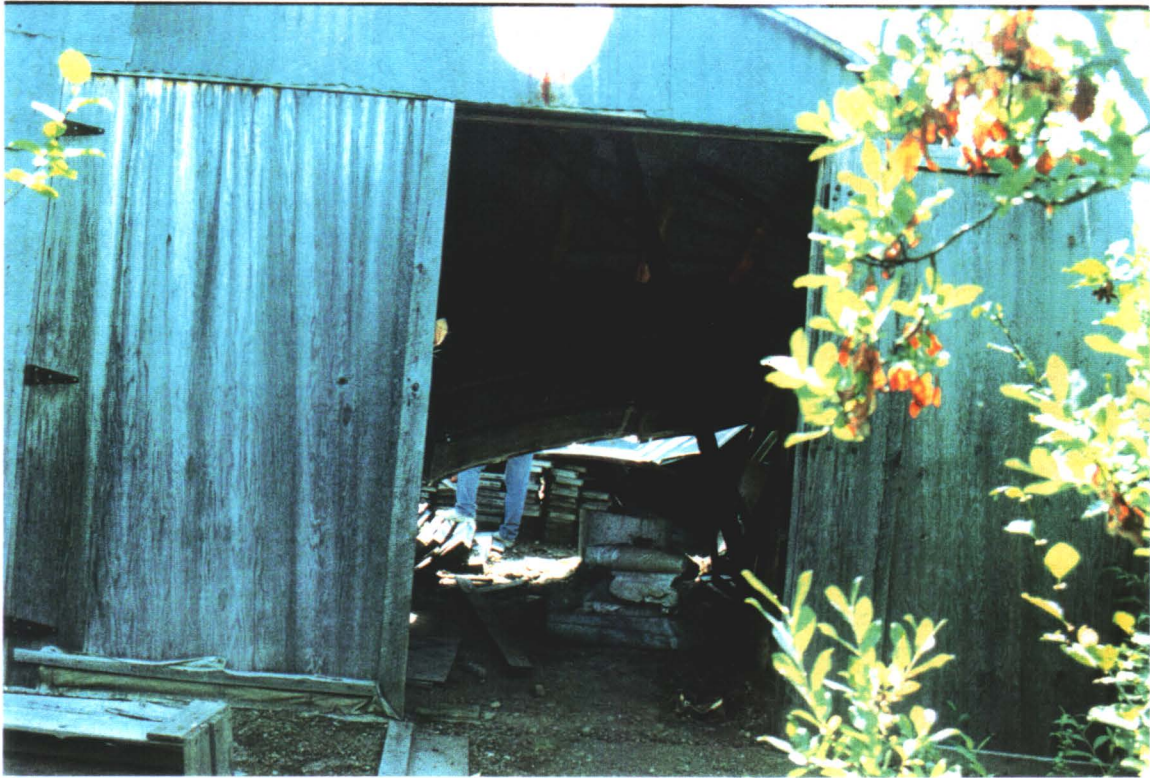
METAL CLAD QUONSET. NOTE ROCK CORE.
