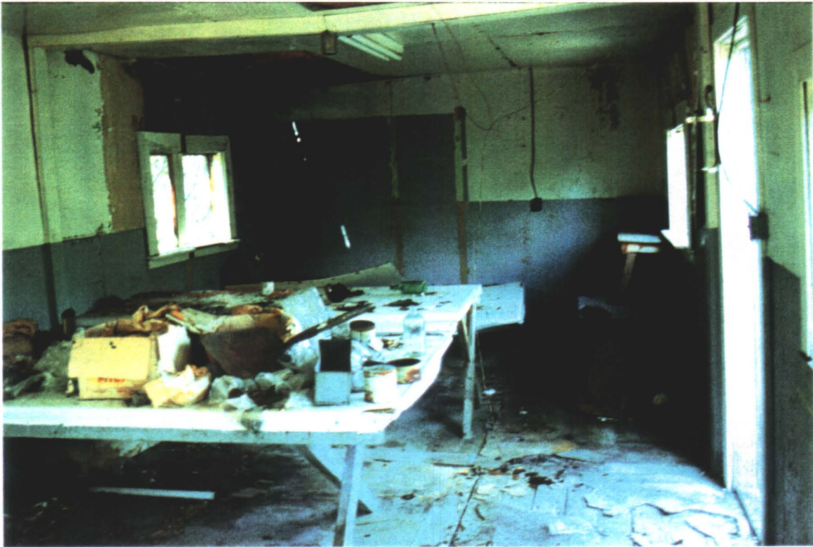
INTERIOR OF OFFICE BUILDING
