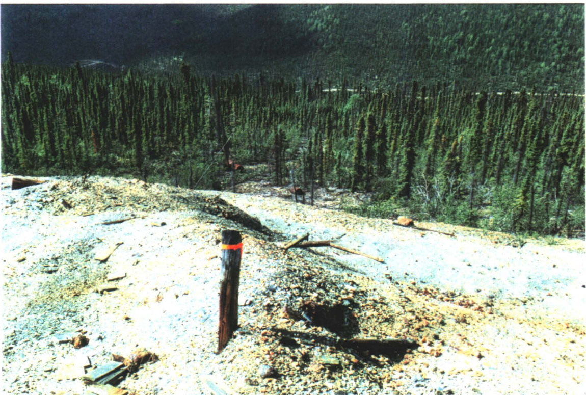
DOWNSLOPE OF WASTE ROCK DUMP SHOWING VEGETATION STRESS
