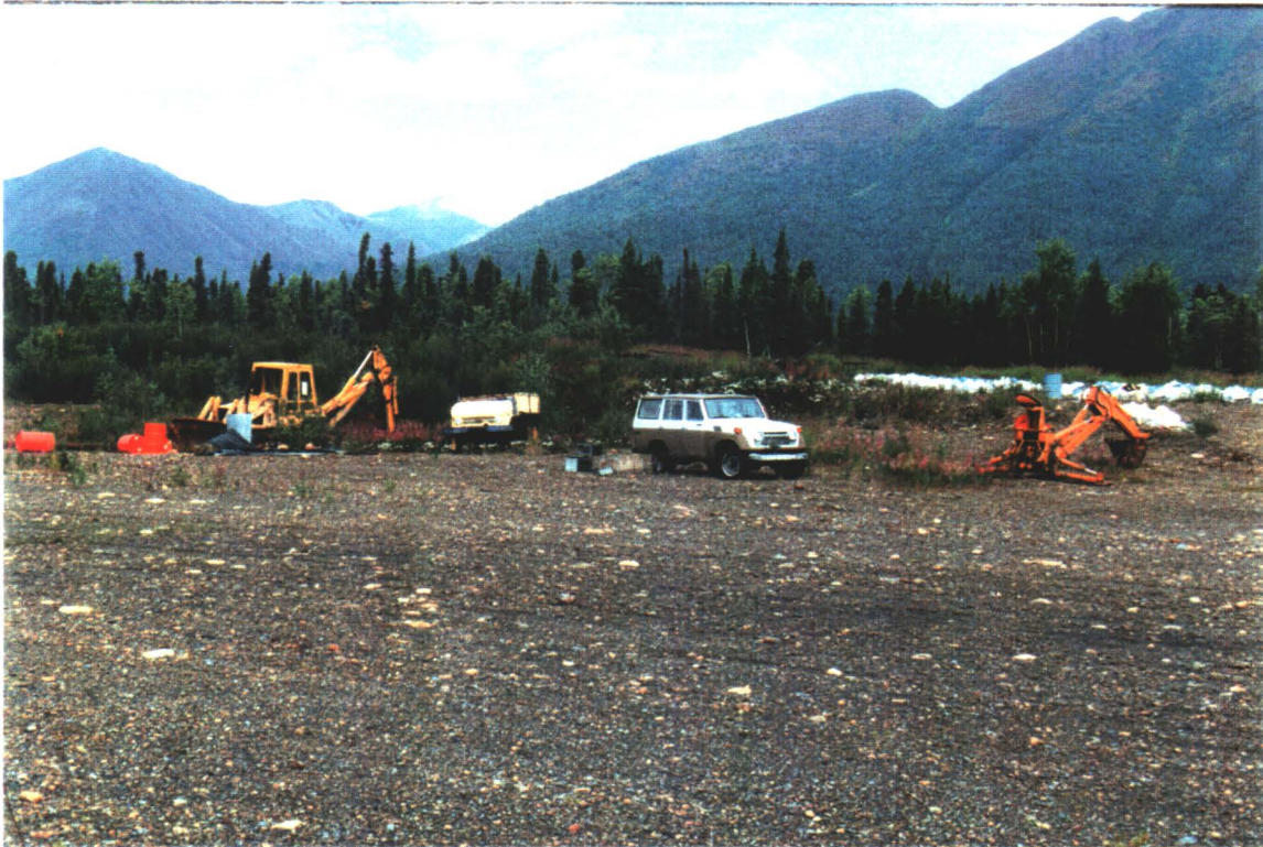
BACKHOE, BACKHOE ATTACHMENT, ALL-TERRAIN VEHICLE, AND LANDCRUISER
