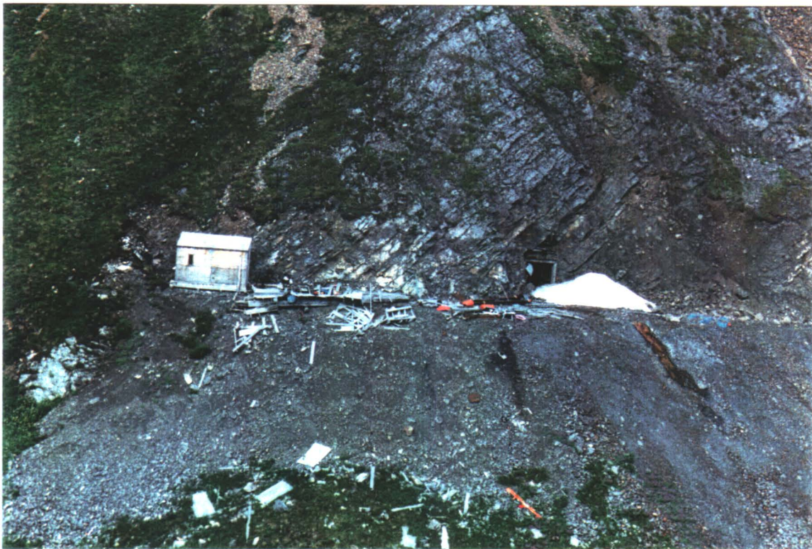
OPEN ADIT AND WASTE AT ADIT
