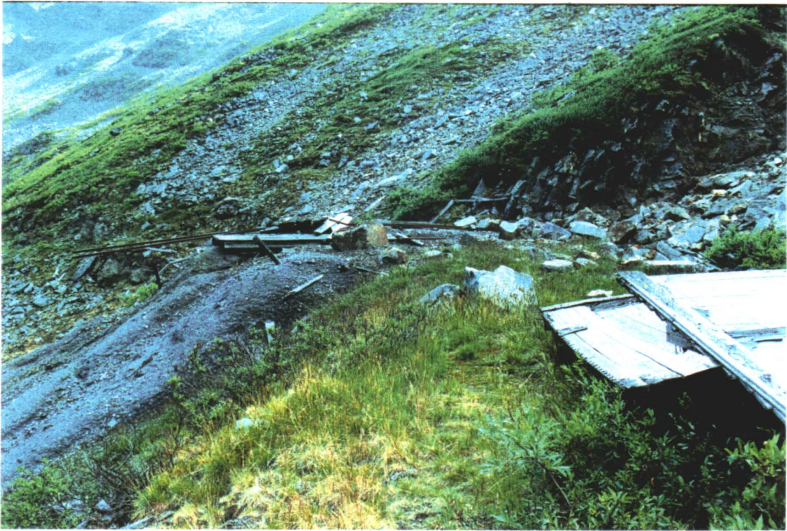
ROCK WASTE, RAIL, AND COLLAPSED BUILDING AT ADIT
