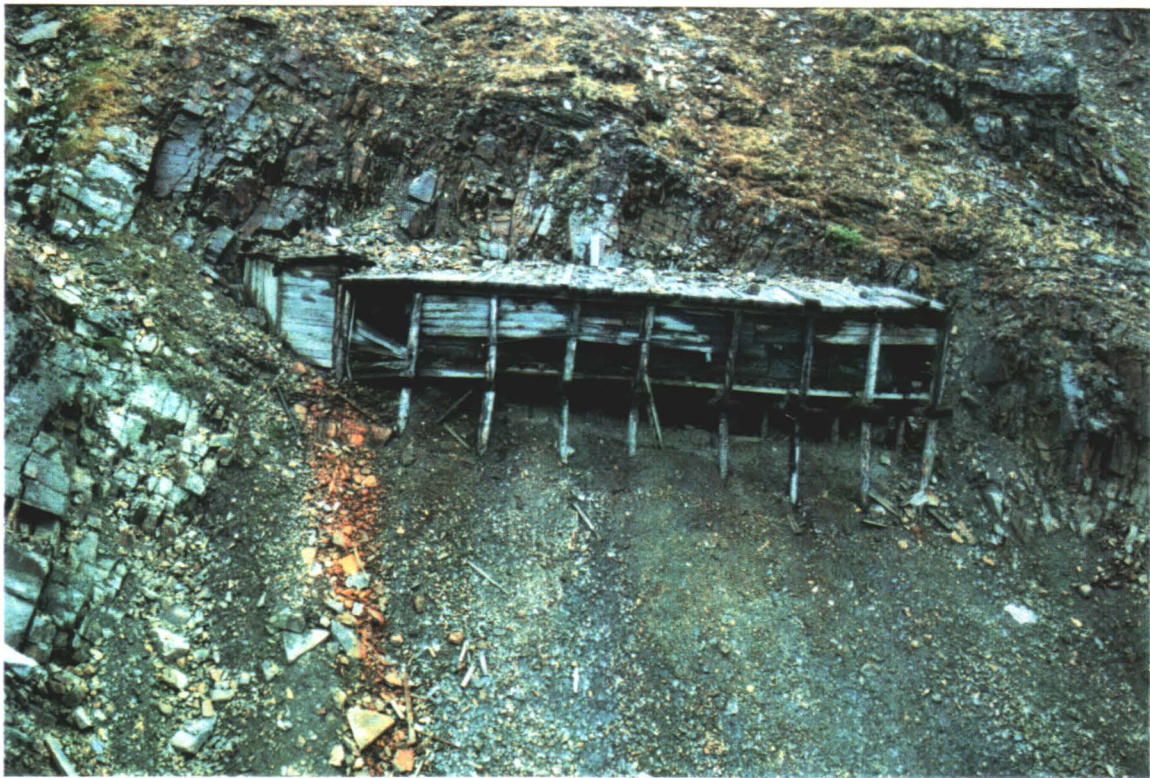
ADIT AND DUMP STRUCTURE ON ROCK FACE
