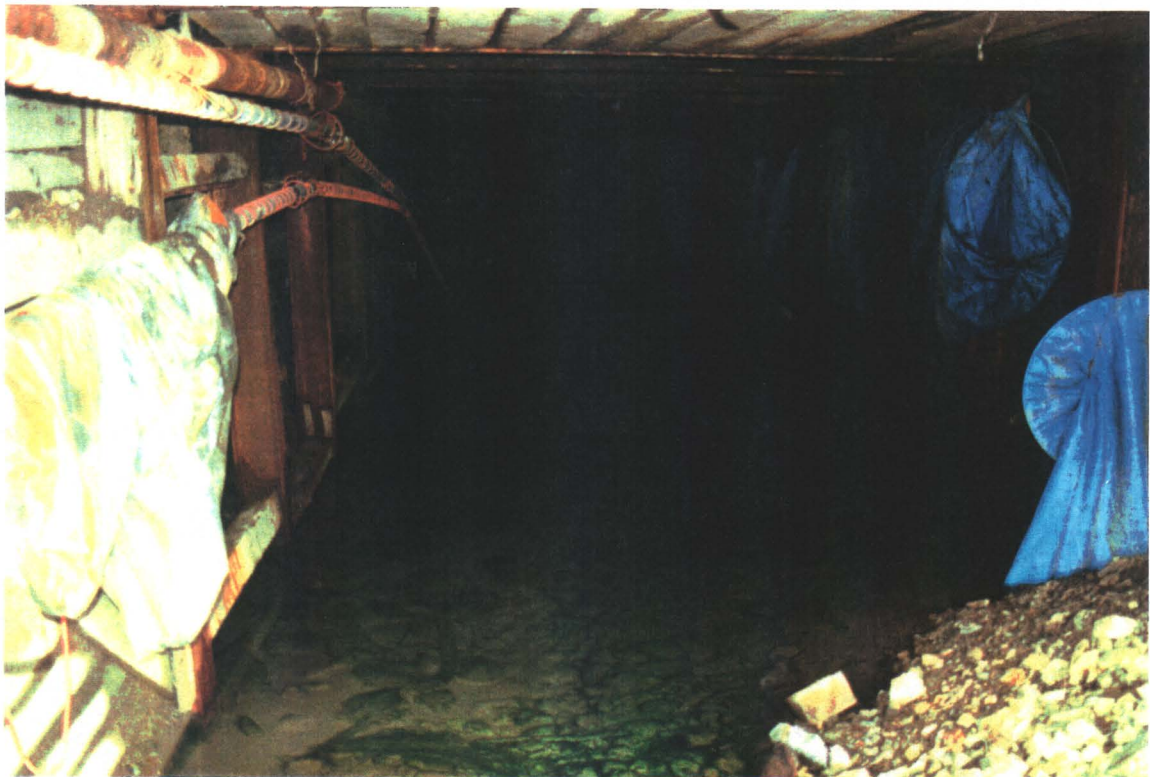
12. INTERIOR OF ADIT
