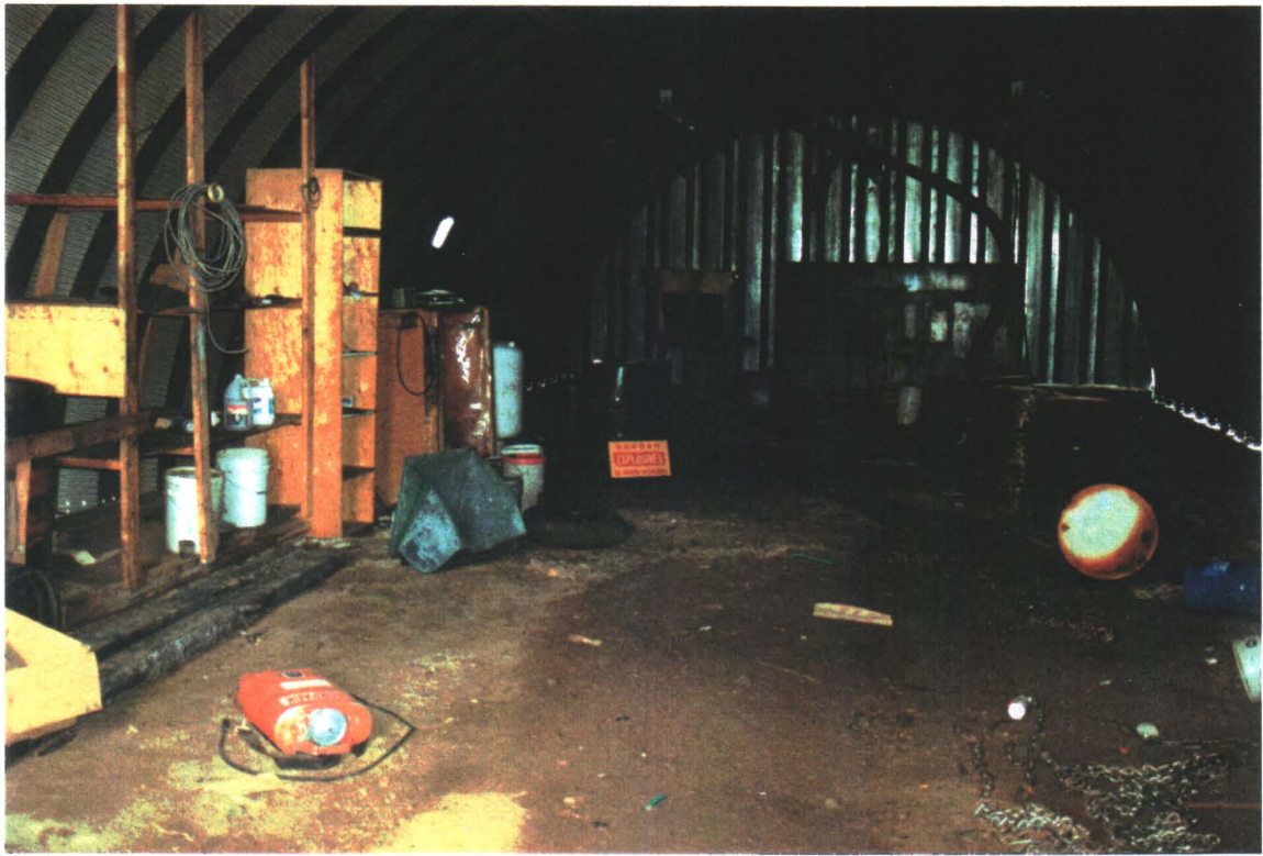
11. INTERIOR OF QUONSET SHED
