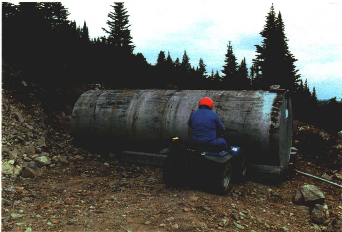
2. LEAKING FUEL STORAGE TANK
