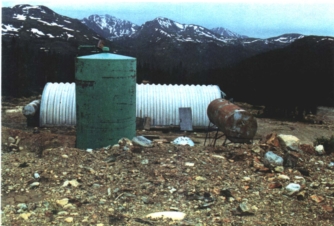
8. 4540 & 22700 LITRE FUEL STORAGE TANKS AND QUONSET SHED AT MAINTENANCE AREA
