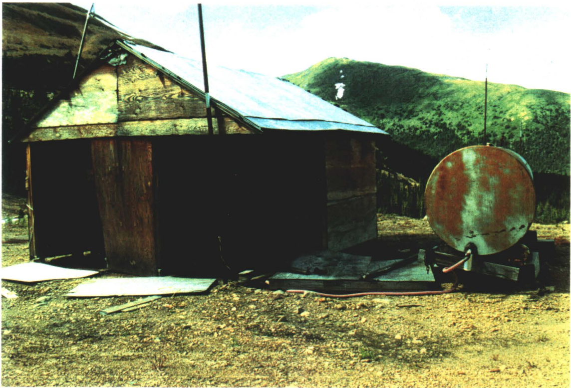
FUEL STORAGE BUILDING AND TANK
