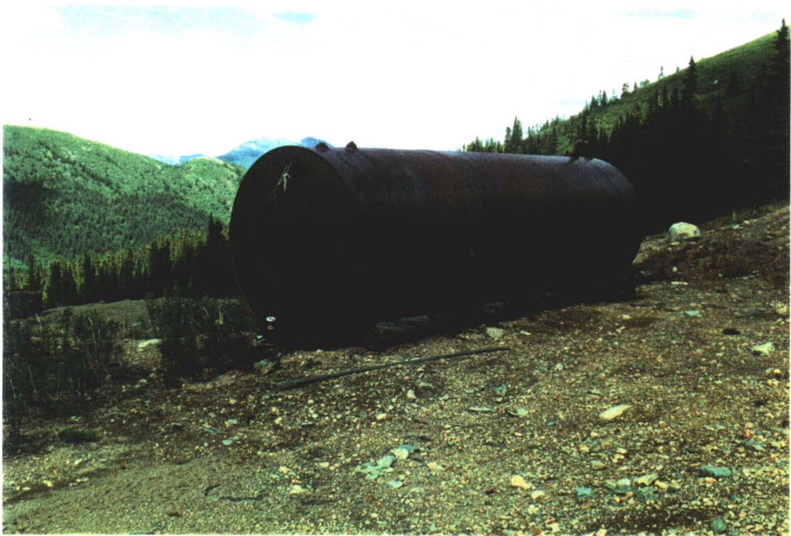
FUEL TANK NEAR CAMP AREA
