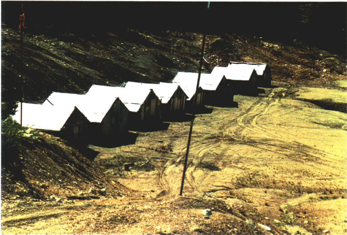
CAMP AREA AND CORE STORAGE BUILDINGS
