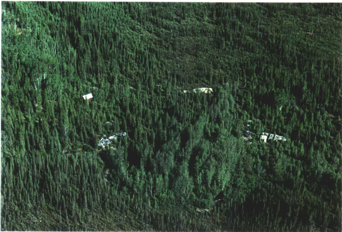
OVERVIEW OF SITE
