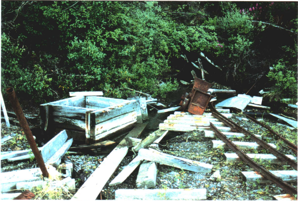
COLLAPSED ADIT AND ADJACENT SHAFT
