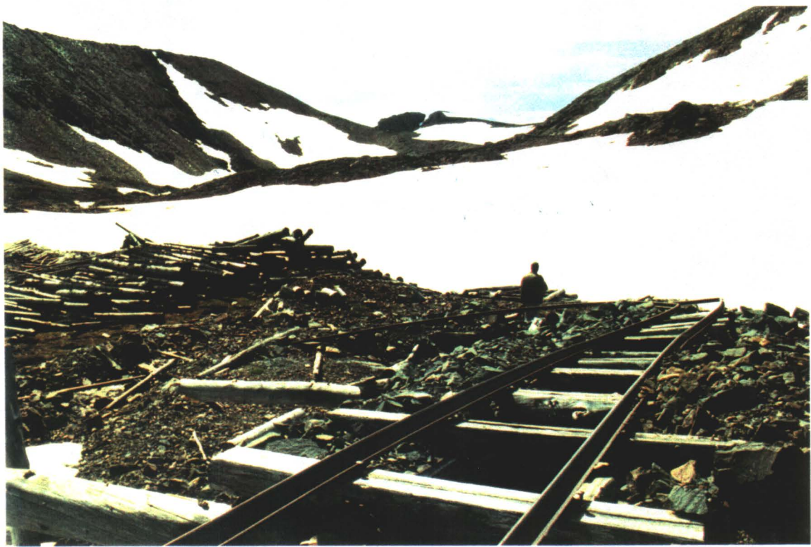
RAIL FROM ADIT, LAGGING ON LEFT
