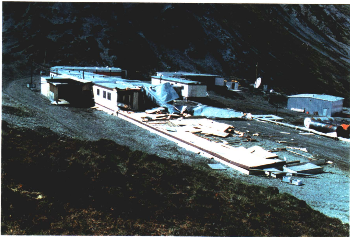
CAMP SITE AND DEMOLISHED TRAILERS FROM AVALANCHE
