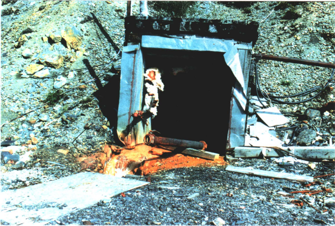
ADIT (NOTE WATER DRAINING AND VENTILATION AND WATER PIPES)
