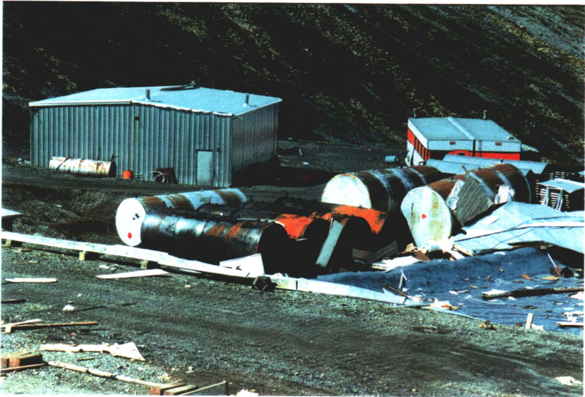
FUEL STORAGE TANKS, WORKSHOP, AND DEBRIS FROM TRAILERS
