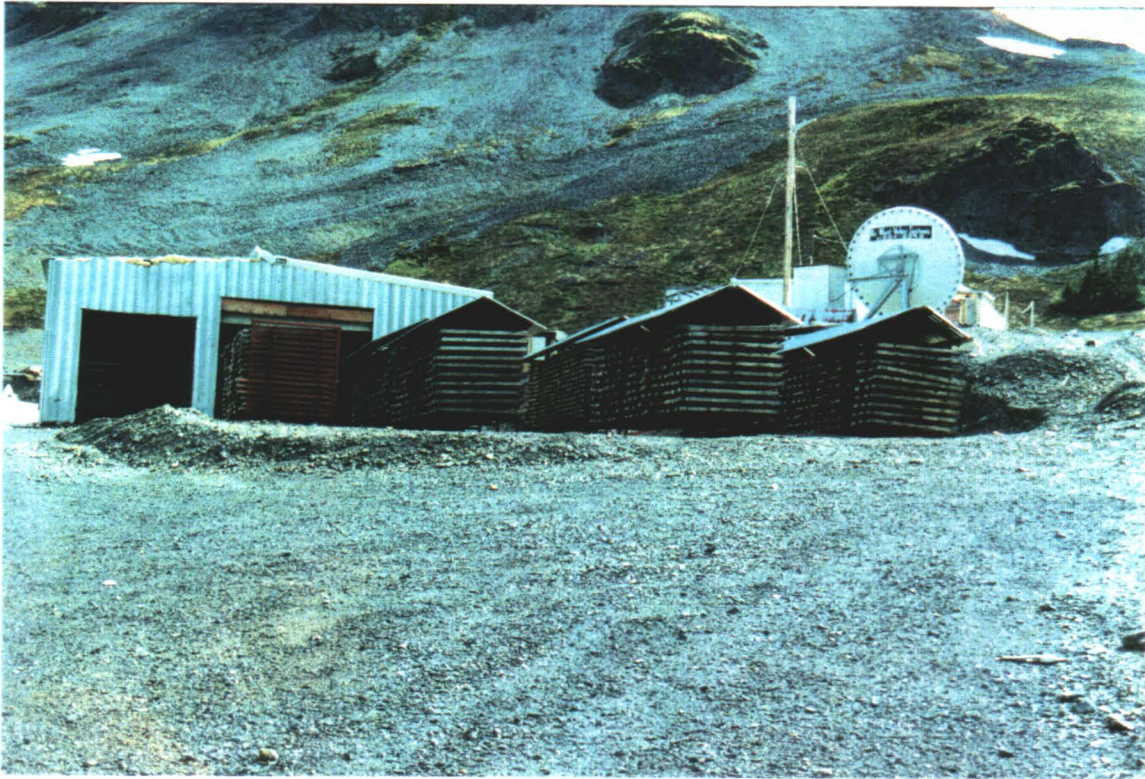
CORE STORAGE AND SATELLITE RECEIVING SYSTEM
