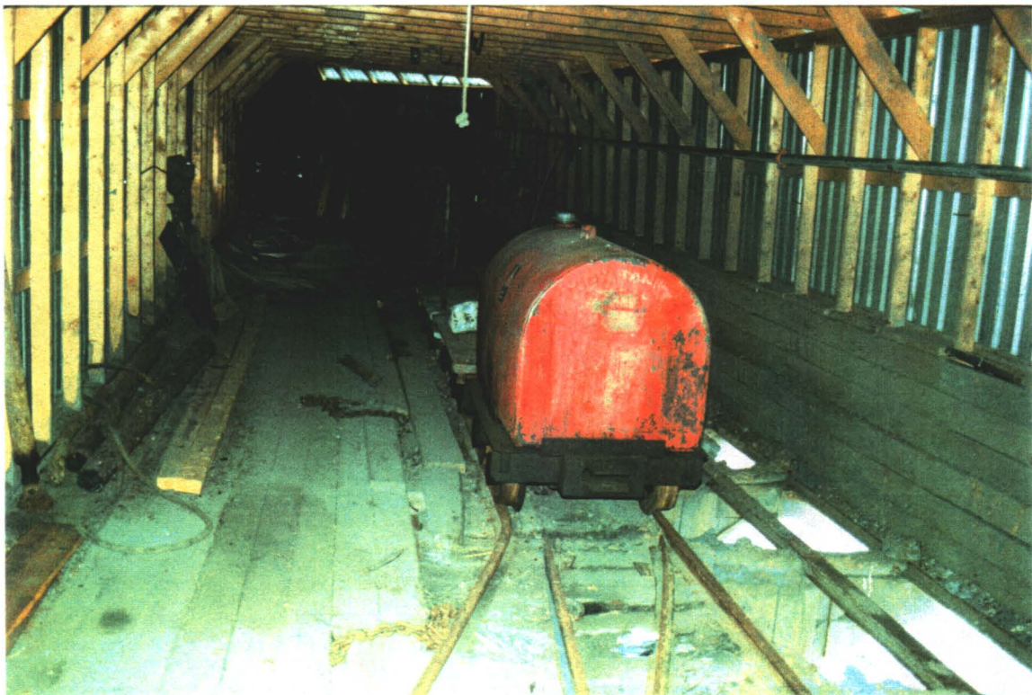
INTERIOR OF LOADOUT WITH ORE CARS AND FUEL TANK
