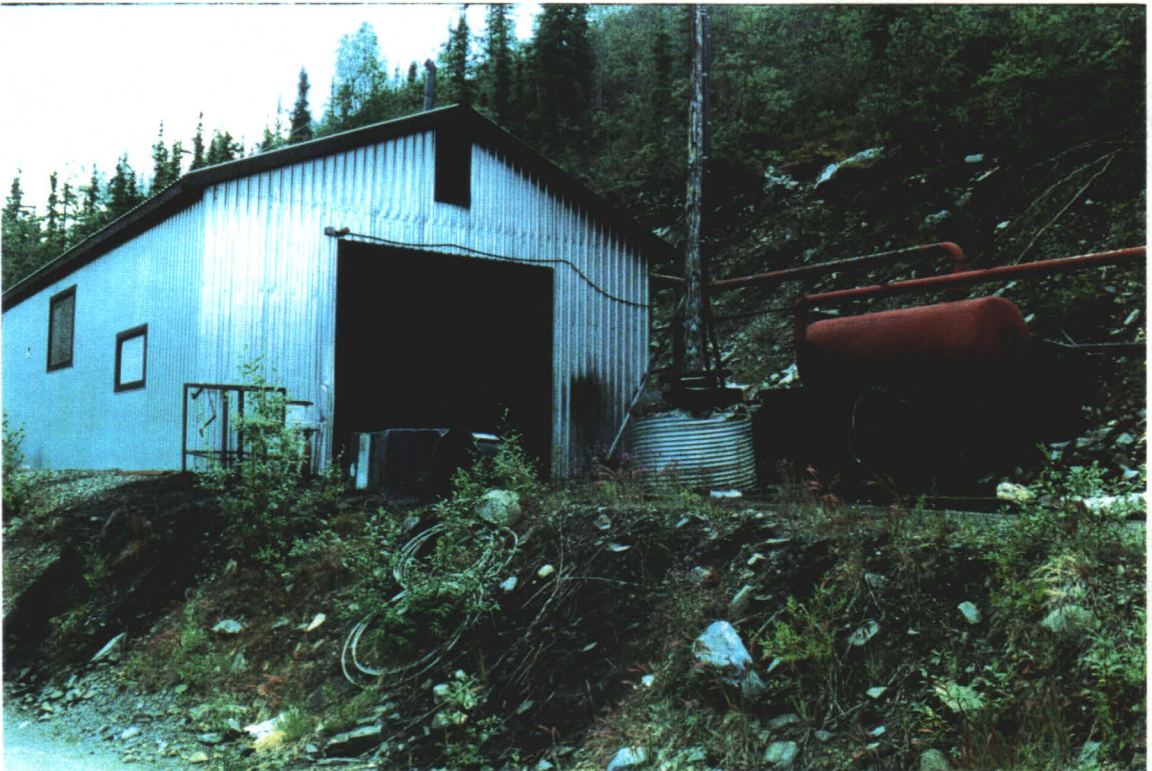
GENERATOR BUILDING (NOTE FUEL SPILL)
