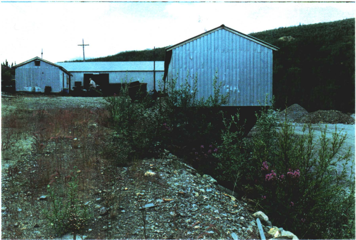
LOADOUT, ENTRANCE TO ADIT, AND STAFF BUILDING
